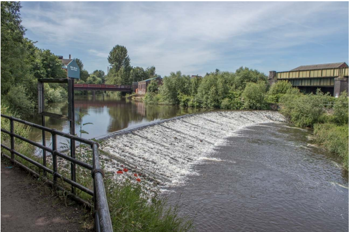
Plate 2: The weir prior to commencement of works. Looking south-west
