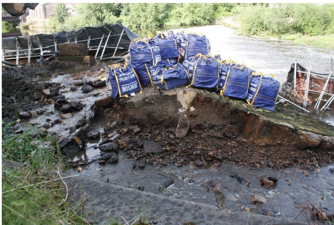
Plate 10: East-facing section through the weir. Looking south-west
