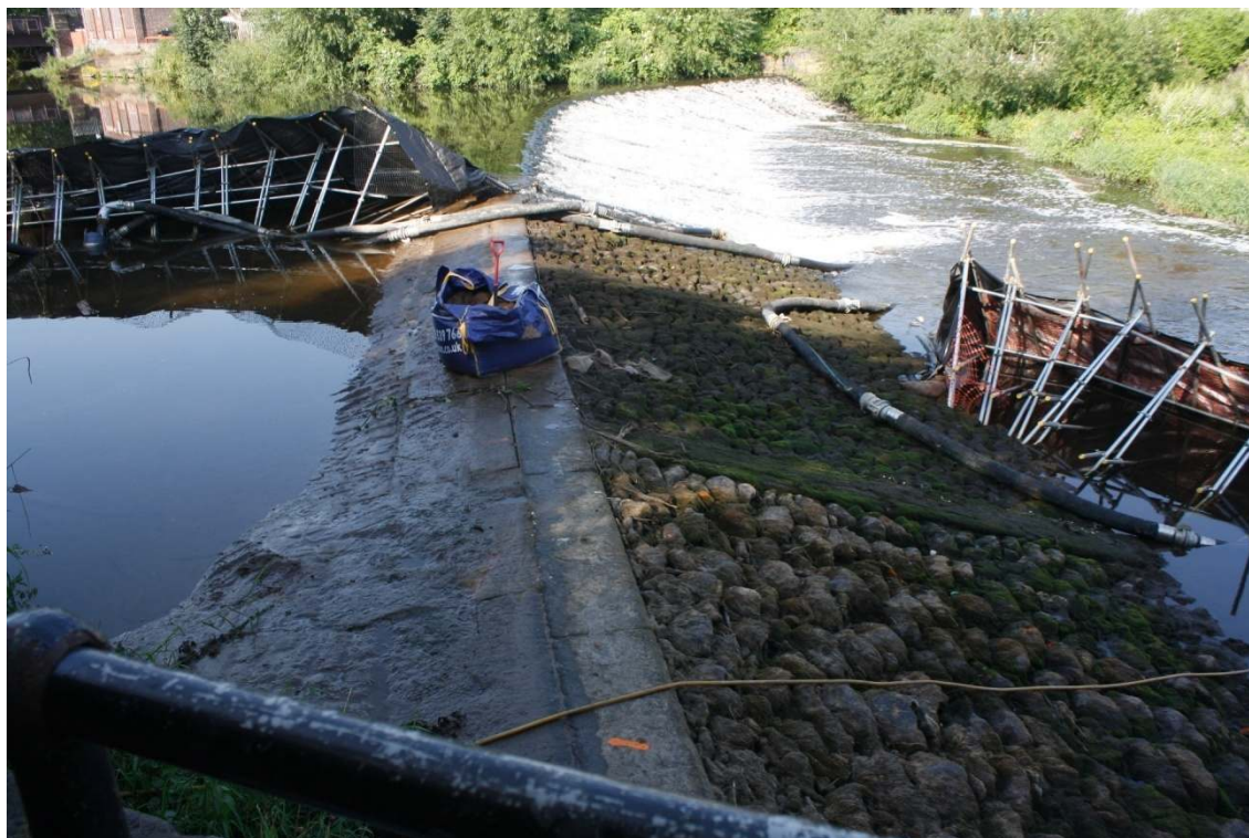
Plate 3: Pre-excitation shot of the exposed weir structure. Looking south-west
