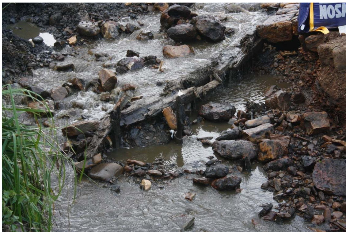
Plate 7: Detail of wooden beam (105) in situ behind stone structure (104). Looking south-west
