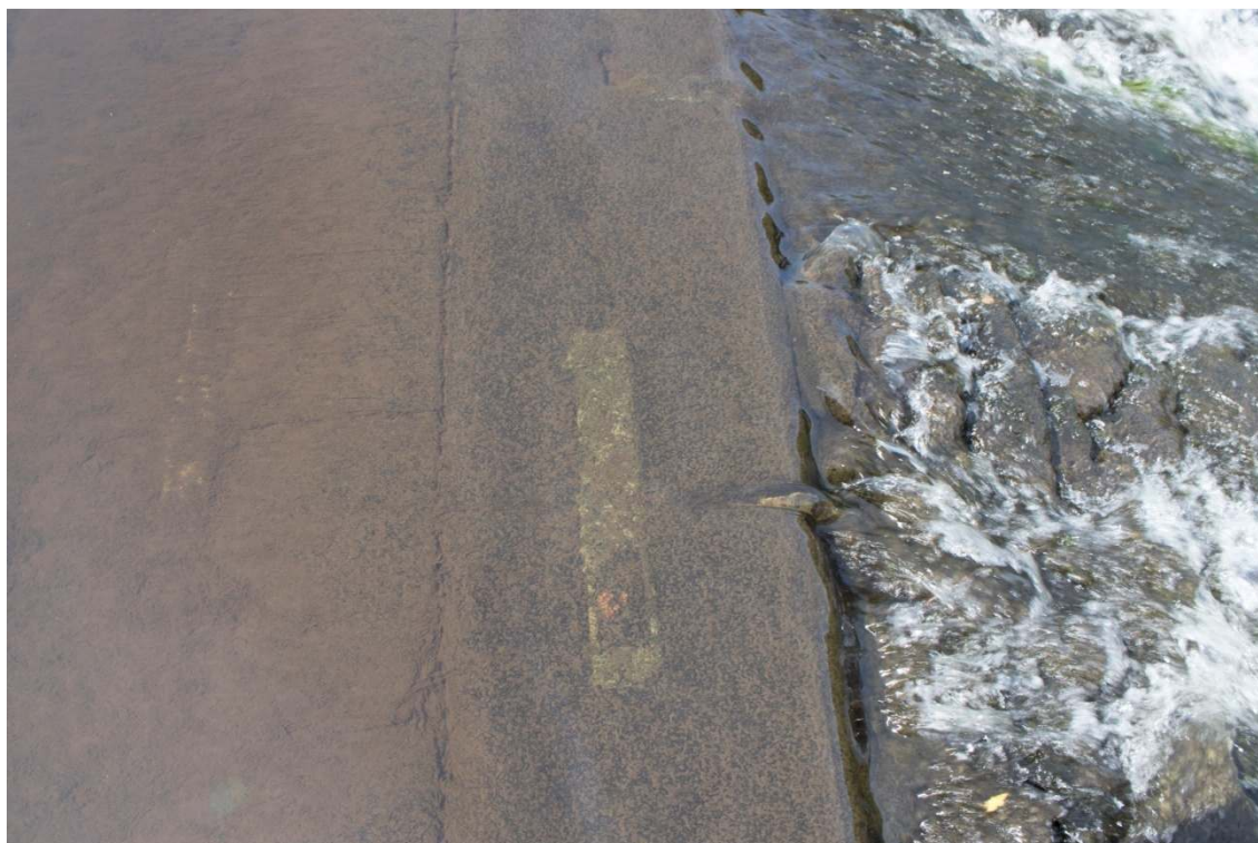
Plate 6: Detail of the metal strapping fastening together (102). Structure (103) also with metal strapping is just visible to the left, with the slag and crozzle structure (100) to the right. Looking south-west. Taken prior to commencement of works
