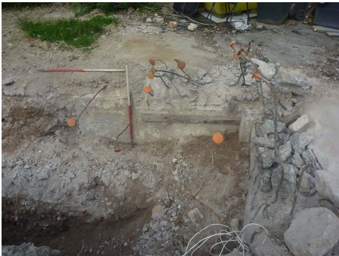
Plate 3: Wall 105, wooden planks 106 and base for metal pad 107 (at right end of trench), viewed facing north (scales in 50cm divisions)
