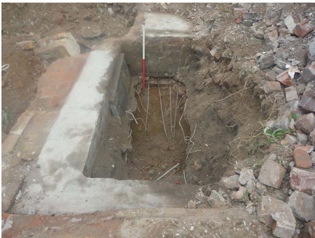
Plate 12: Structure 207 following removal of part of the floor, viewed facing north
