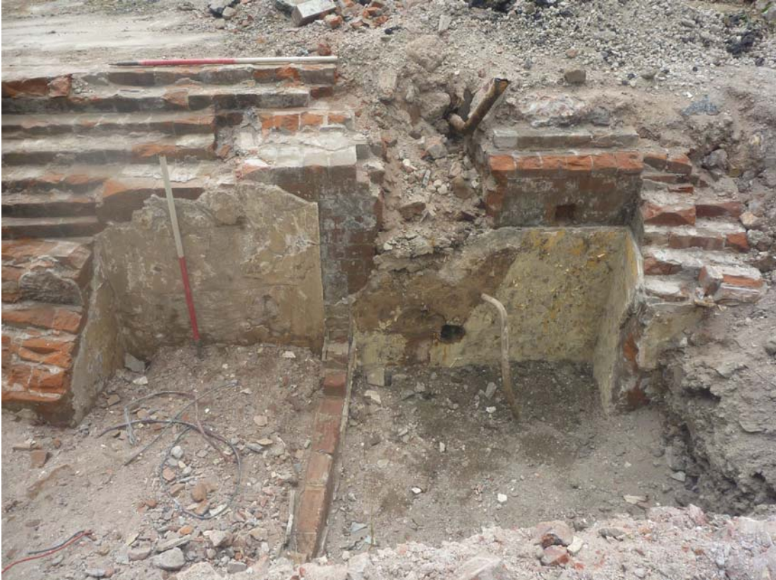
Plate 7: West part of wall 209, showing pipe cut 217, and partition wall 211 in the centre, viewed facing north
