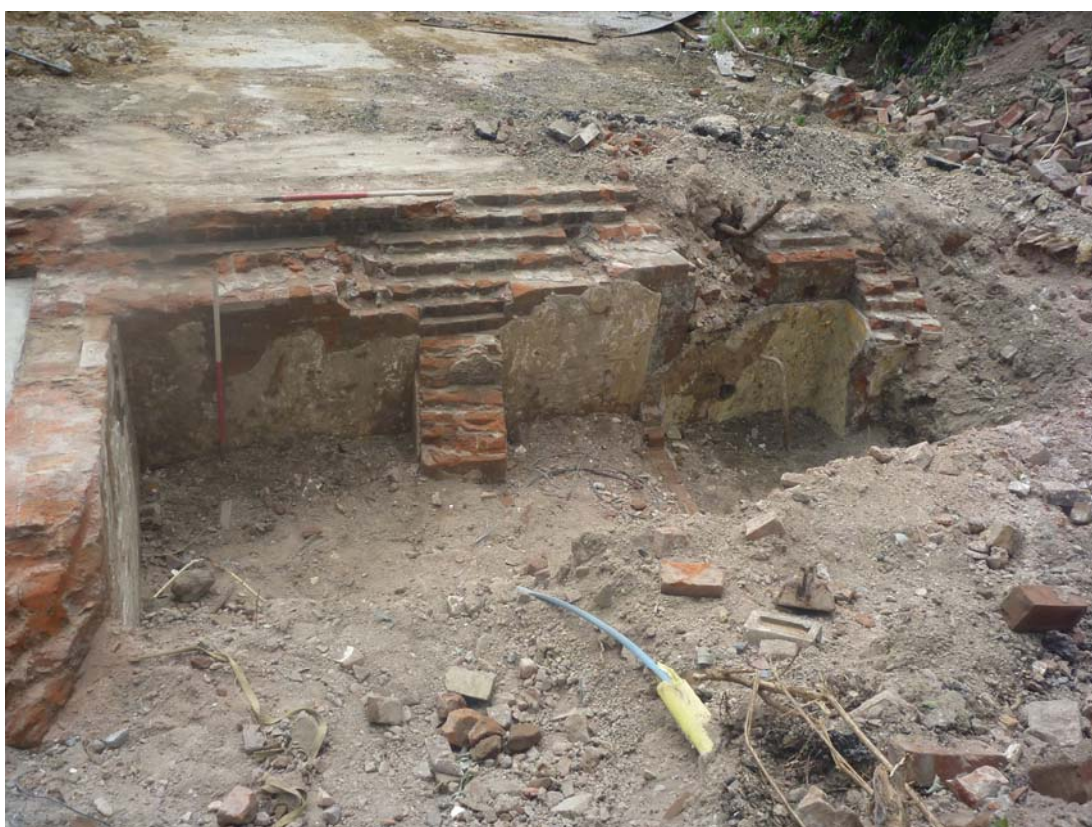
Plate 6: Wall 209, viewed facing south, with wall 208 to the left and buttresses 210 and 212 to centre and right
