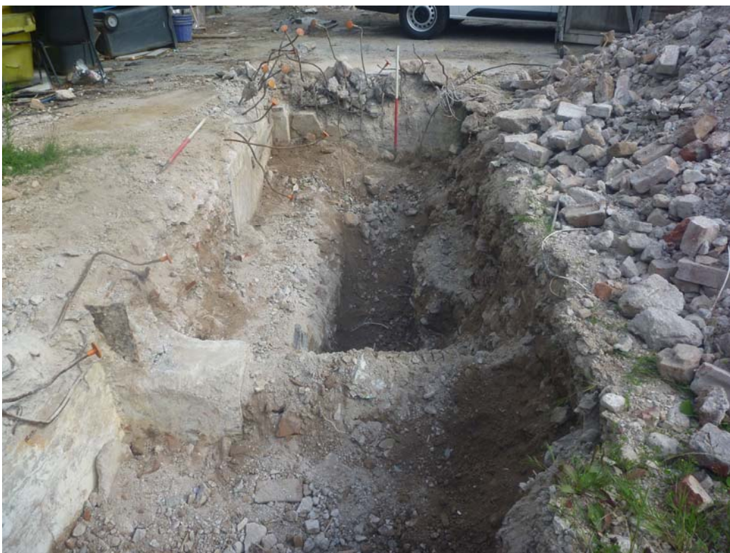
Plate 2: Trench 1, south end, viewed facing north
