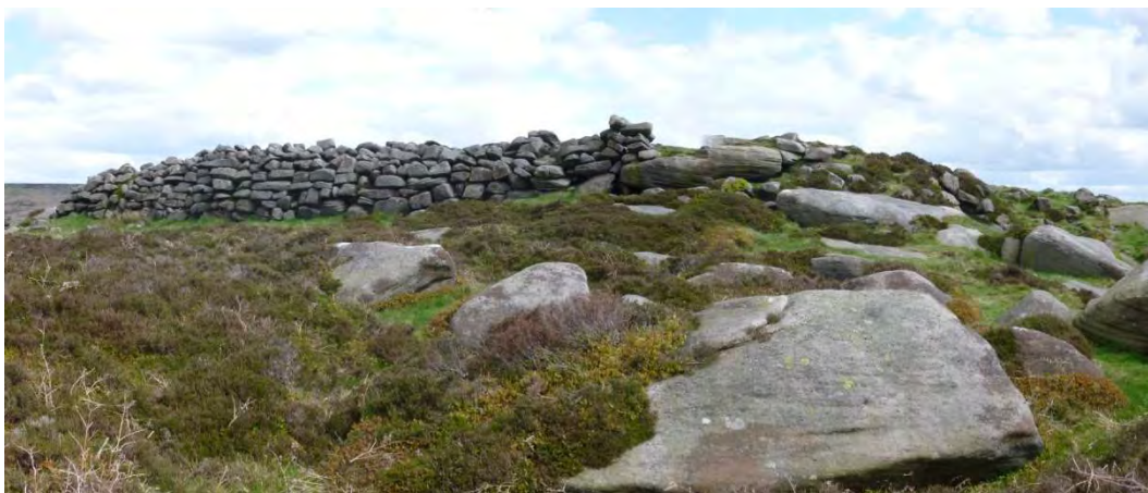
Plate 5: Rampart and revetment wall, west side of Carl Wark
