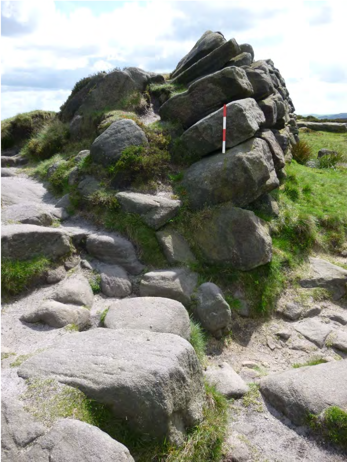
Plate 36: North 'entrance' to Carl Wark, showing section through rampart. Foundation stones in foreground show that the rampart originally continued to the cliff edge (feature 86)
