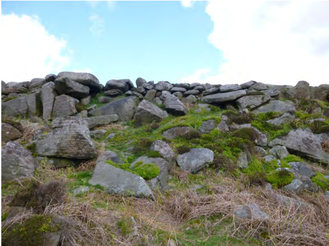
Plate 24: Boulder wall forming southern edge of Carl Wark, four courses high (feature 83)
