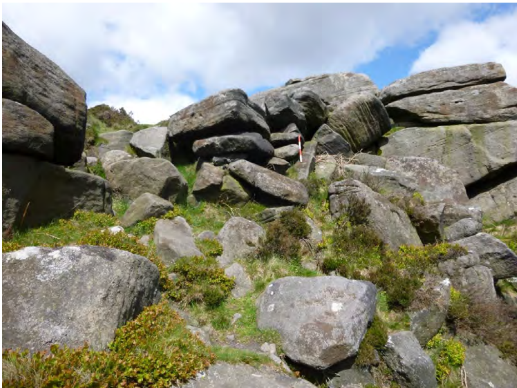
Plate 19: Boulder wall enhancing the natural cliff edge at east end of Carl Wark (feature 73)
