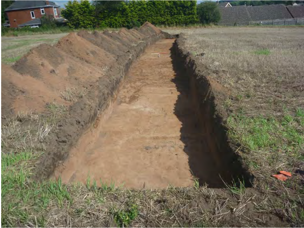
Plate 5: Trench 3 viewed facing west, 2 x 1 metre scales.
