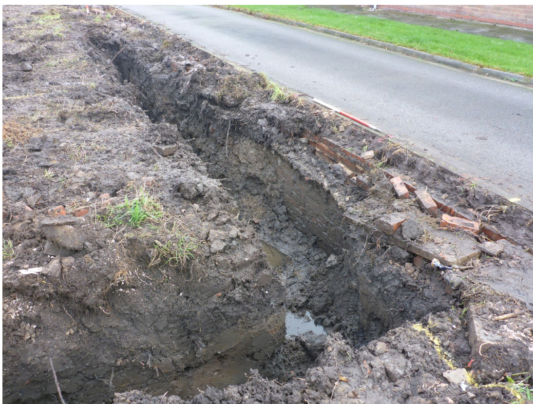
Plate 6: Wall 203 at the south edge of Plot 2, surrounded by fill 201, viewed facing southeast
