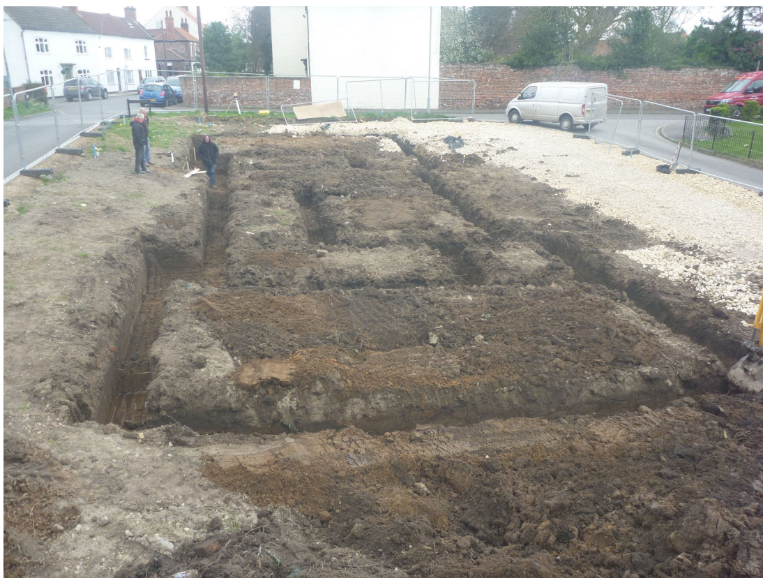
Plate 7: View east across the excavated foundations in Plots 3-5
