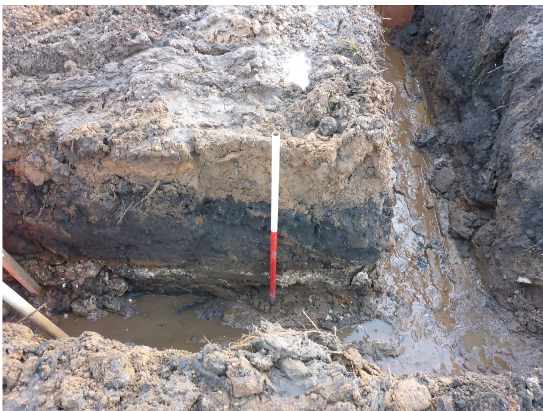
Plate 4: North-facing section of northern foundation trench in Plot 2, showing mortar spread
