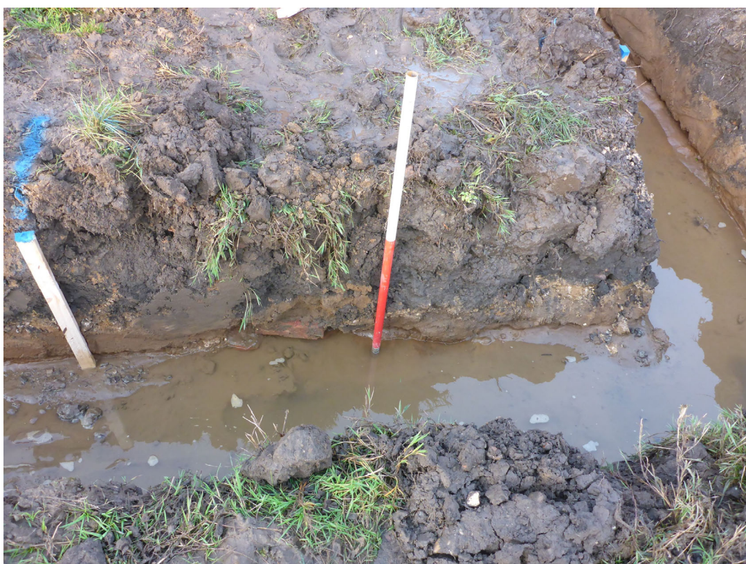
Plate 2: South-facing section of southern foundation trench in Plot 1, showing brick drain
