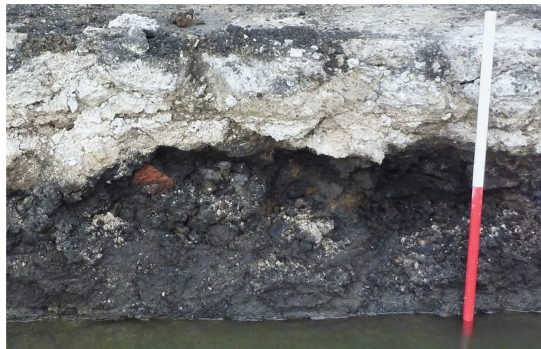
Plate 2 Trench 1, south-east facing section showing rust brown slag and black sand deposit (1003). Concrete 1001 above, Deposit 1004 below. 1m scale
