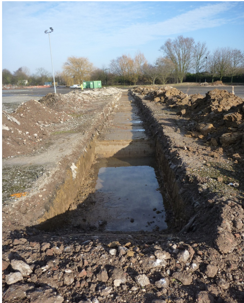
Plate 3 Trench 2, general shot looking north-east. Increased depth dig in foreground
