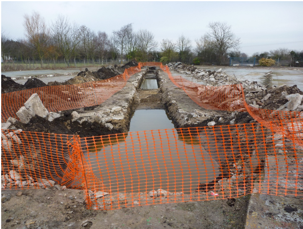
Plate 1 Trench 1, record shot looking North-east
