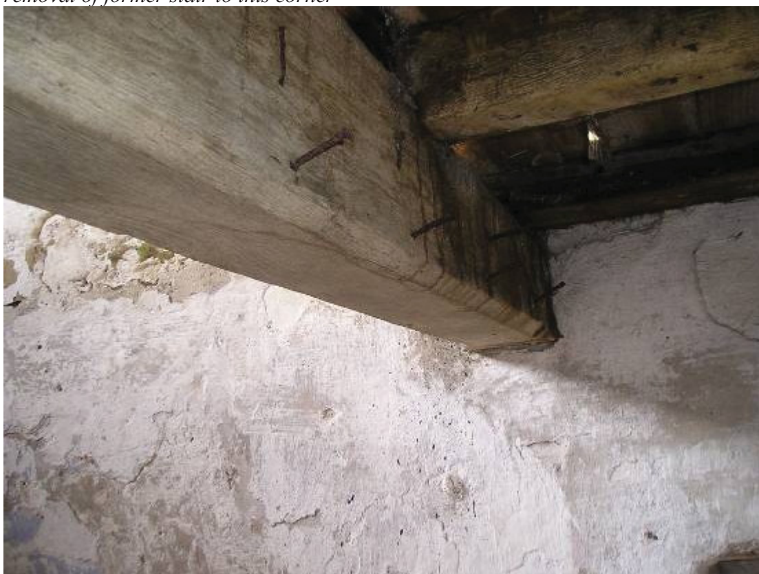
35. Detail of chamfered beam (with run-out stop) supporting loft floor in cottage bay
