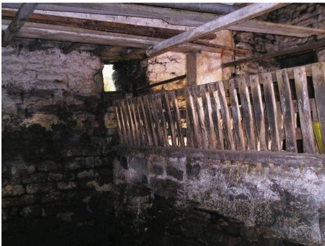
24. View in shippon bay to barn with low wall to the right showing drop in level from cart entry bay (right) to shippon floor.
