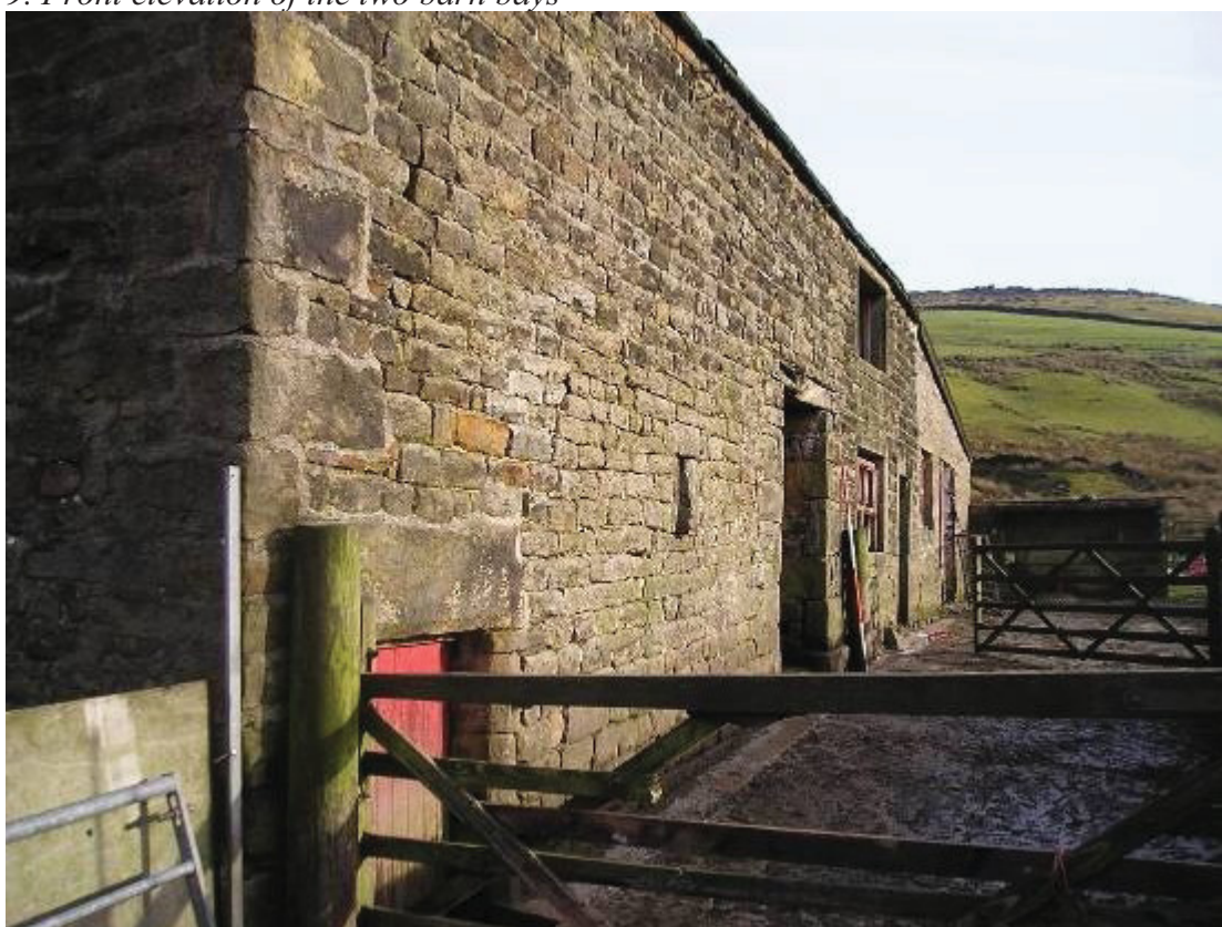
10. View along front elevation from the west. Note shippon entry door in the foreground with chamfered reveals serving shippon at lower level.
