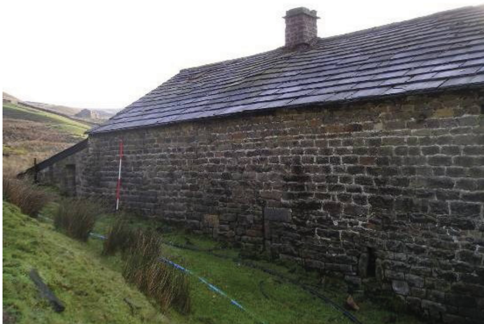
16. Rear elevation – note blocked former door to the centre (see also 17) which opposes cart door to the front elevation. This shows that land to the rear was once dug away to reveal more of the wall than is now visible.
