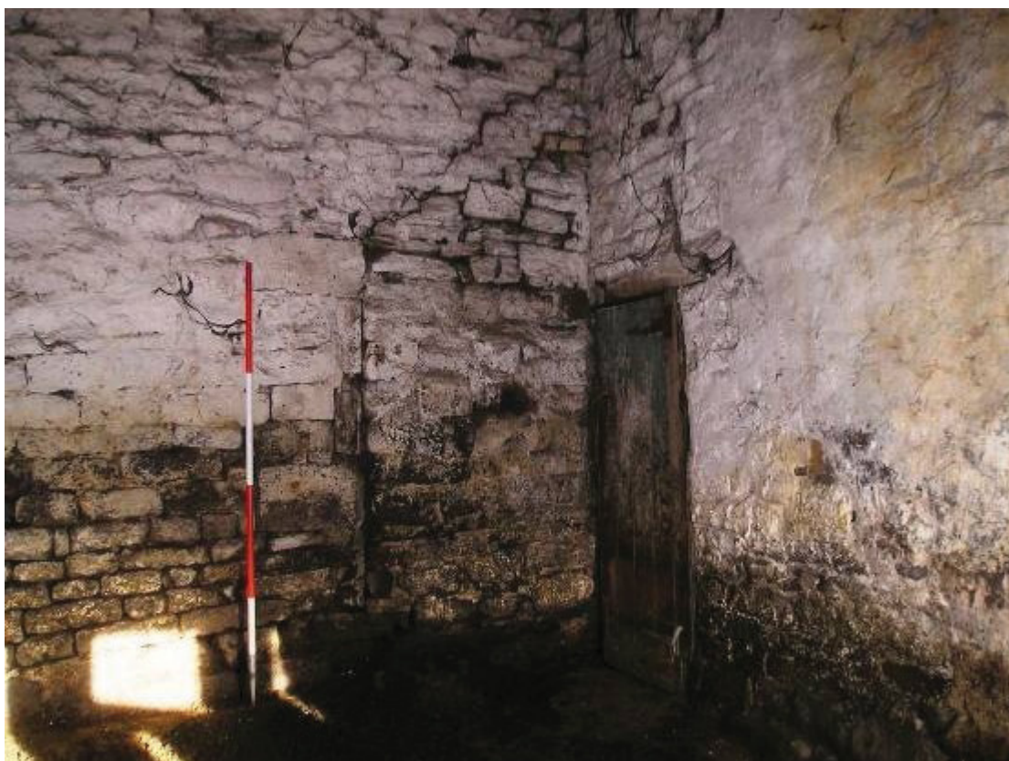
19. Barn interior – looking to rear wall and blocked former door with inserted door to the right giving access to the cottage bay
