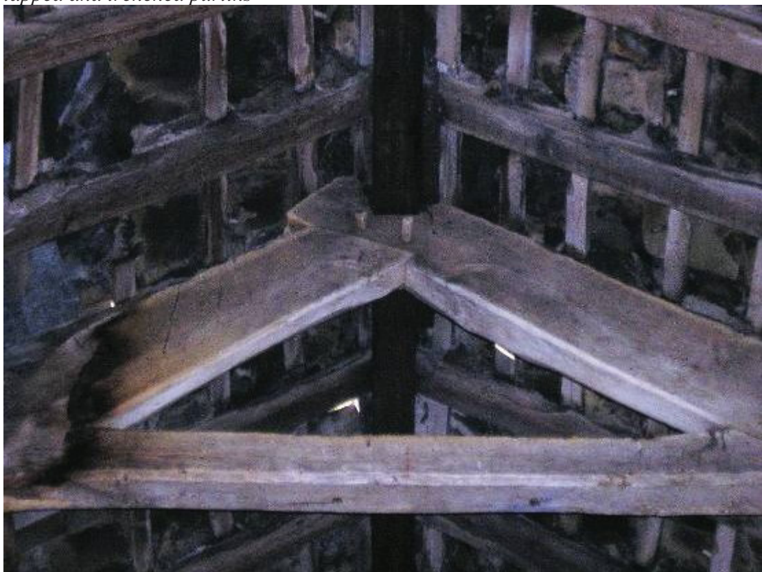
22. Detail of truss apex
