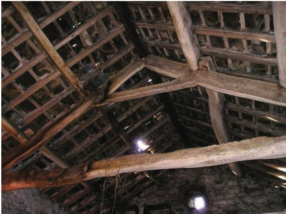
21. Truss to barn, with collar, overlapped and pegged principals at the apex and lapped and trenced purlins
