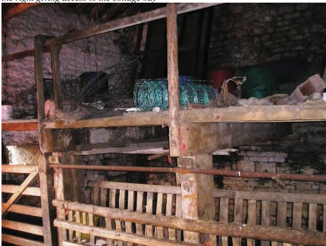
20. Barn, looking to west end with loft over lower shippon – note feeding rack
