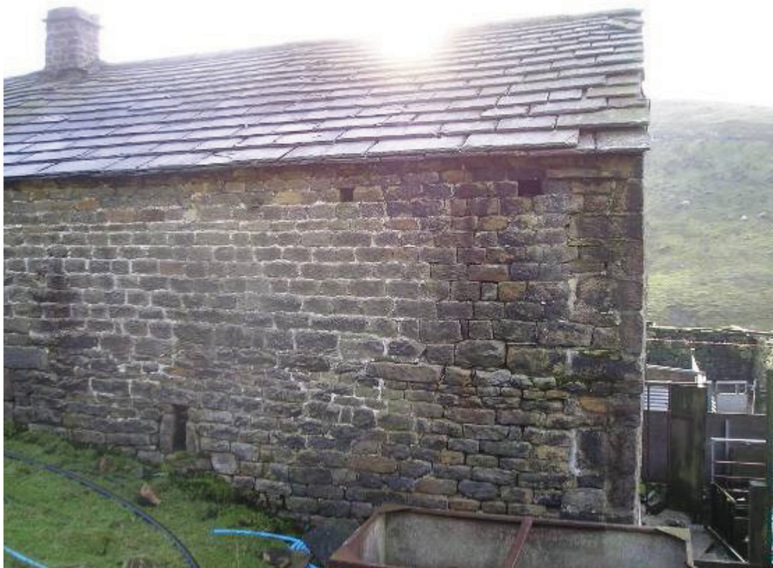
15. Rear elevation of the barn part. Note the variation in coursing to upper and lower levels: this might indicate past alteration or even evidence of an older building that has been reused. The exact nature of such variation, though, remains unclear.
