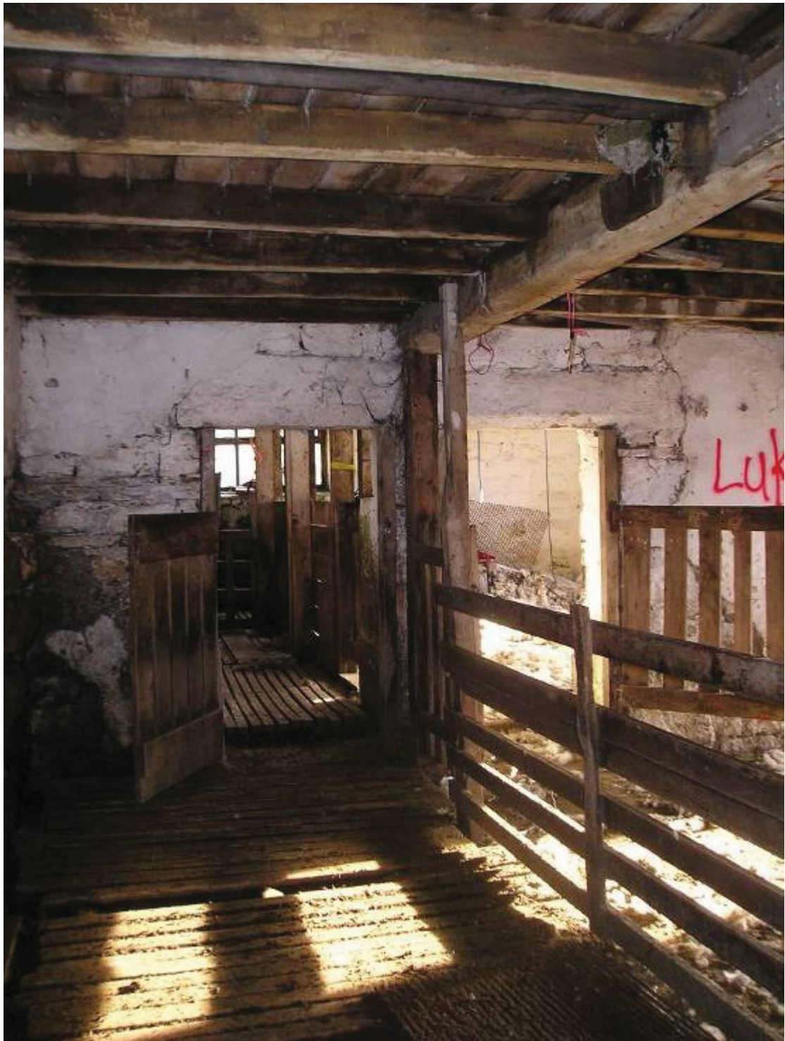
29. View east along rear part of cottage bay (ground floor) showing inserted wooden railing and walkway for movement of sheep into shearing area (east end of the building)
