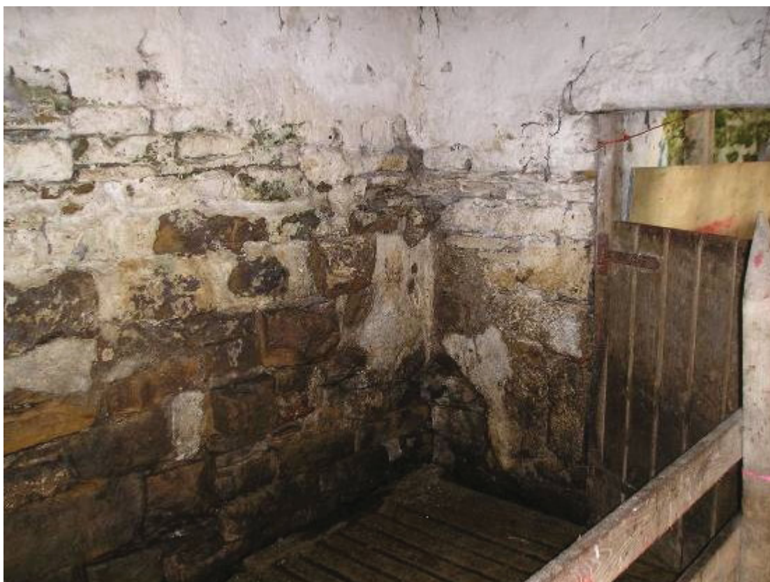
34. Rear part of cottage bay showing stepped stones to rear wall suggesting possible removal of former stair to this corner
