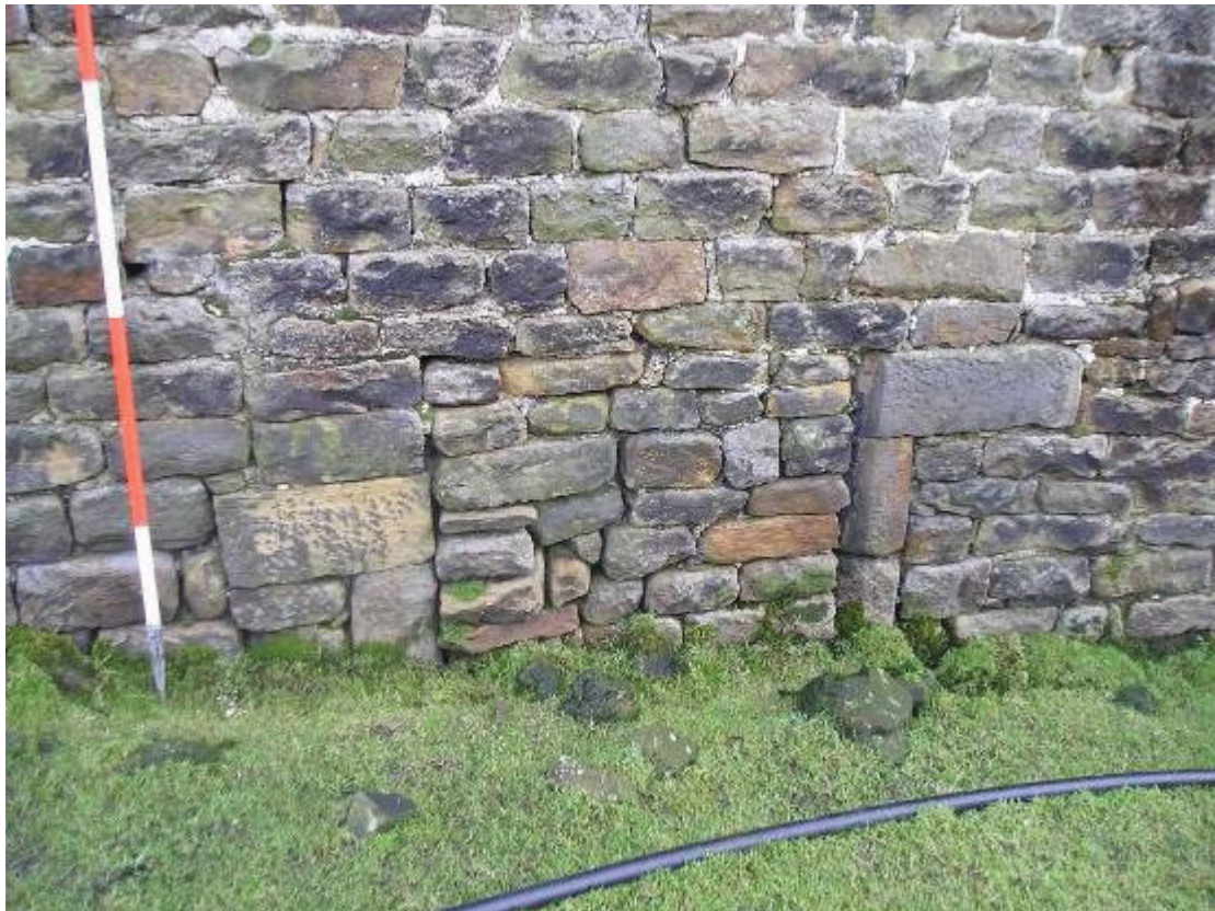
17. Detail of blocked former door to rear elevation
