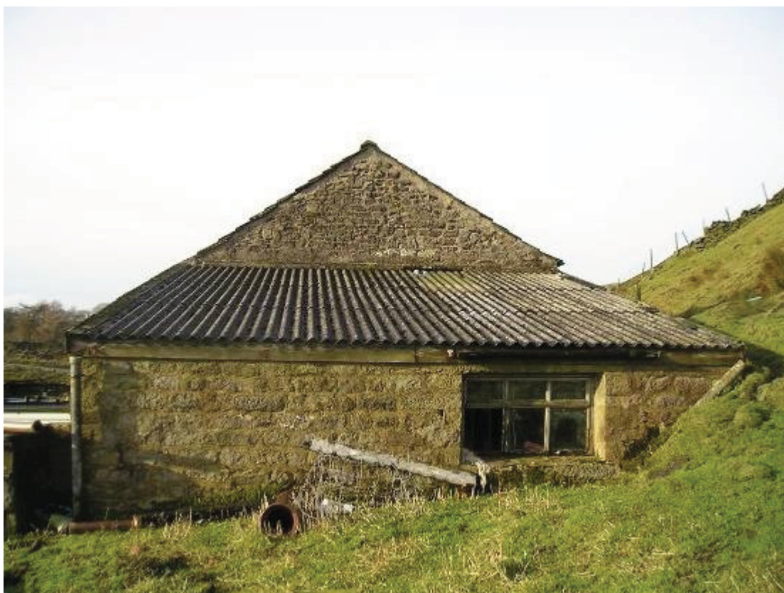
11. Eastern elevation, with lean to in the foreground and rising gable of the cottage above. This upper wall bears no real evidence of ever having been plastered for interior use, thus questioning whether the dwelling did indeed continue to this western end of the range
