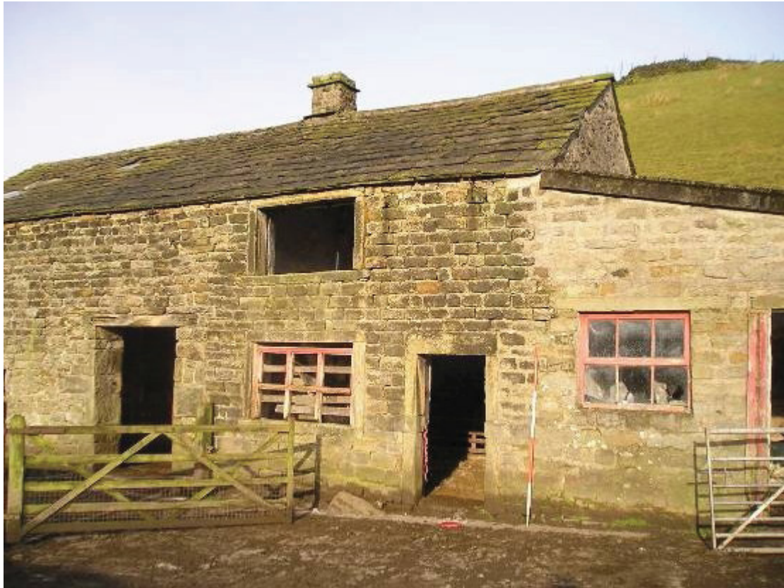
6. Front elevation – centre part showing cottage bay with adjoining altered single storey part to the right and barn to the left. Disturbance of the upper coursing where cottage and single storey part meet indicates that the single storey may have been added or lowered (as mentioned earlier). Evidence in the interior suggests (connecting doorways) that the single storey part was in fact two storey and once part of the dwelling.
