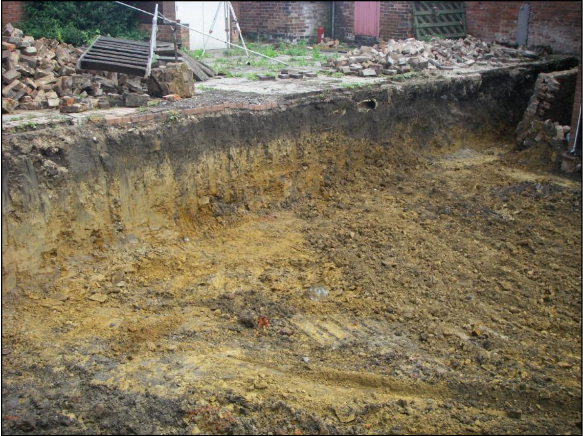
Plate 5: South-facing section of area cleared behind the Masonic Hall, Ilkeston.
