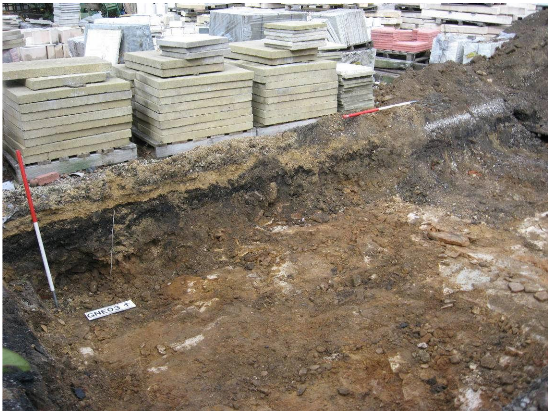
Plate 10: Trench 03 south facing section, looking north-east.
