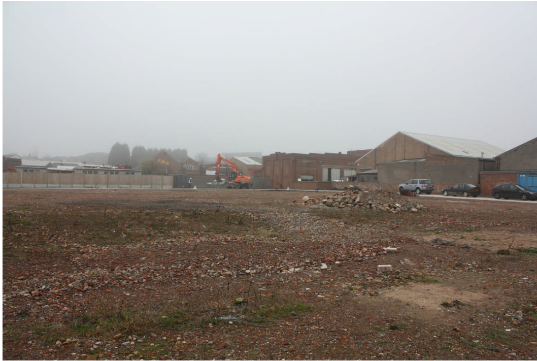
Plate 1: The site prior to evaluation taken from the south-east corner, viewed looking north-west
