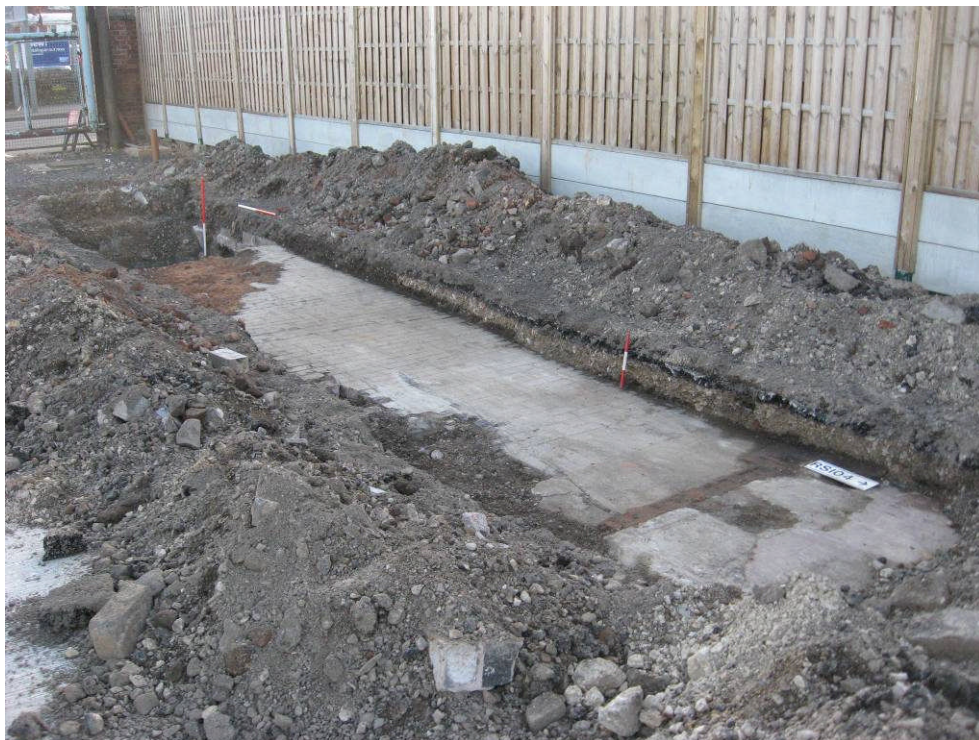
Plate 12: Trench 04 brick floors and walls 0082-0086, viewed looking south-west
