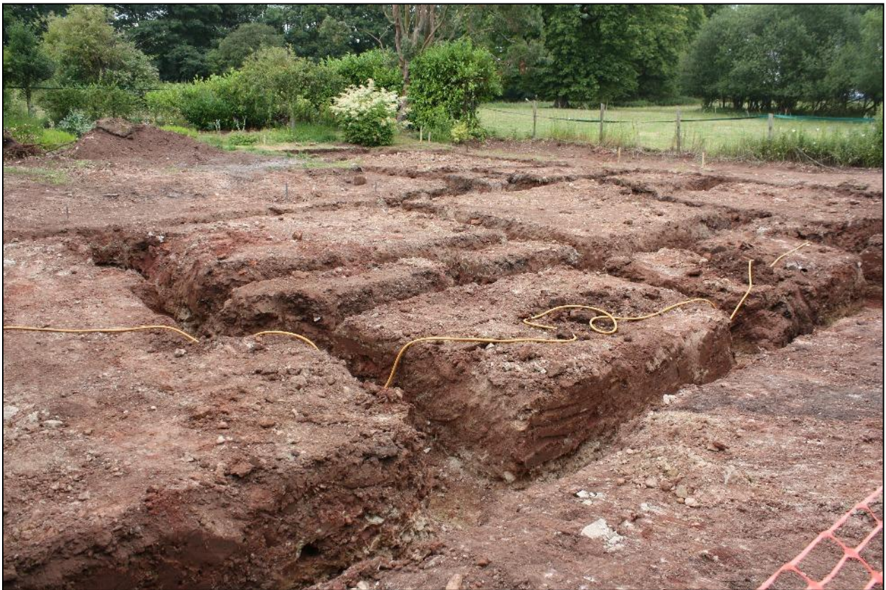
Plate 2: General site appearance after trenching, viewed looking north
