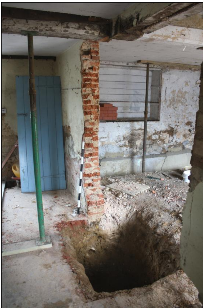
Plate 37: North end wall seen from the interior with new brick patching where the walling had deteriorated and in places found to contain soil.
