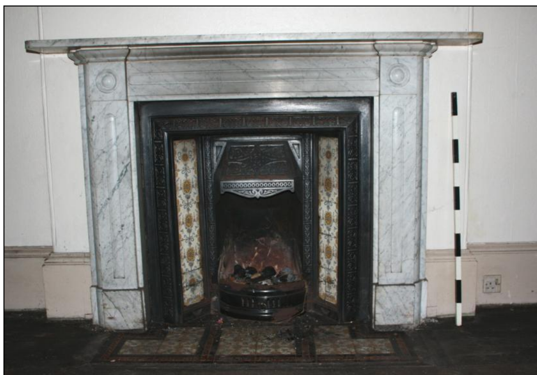
Plate 24: Late Georgian / Regency style marble surround to the fireplace (with later tiled grate) in the Drawing Room.
