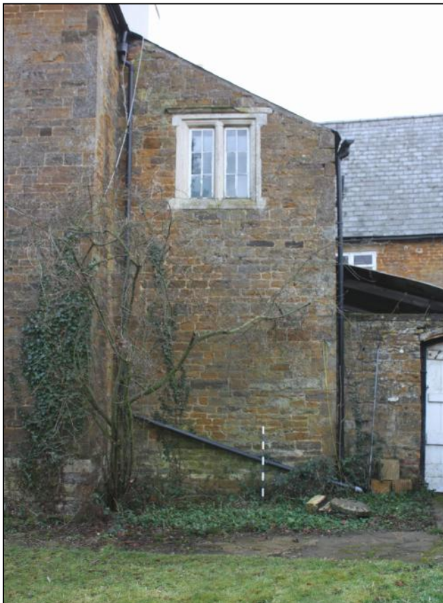
Plate 4: East side view of the lower service part of the Phase 3 wing, here showing a reused mullioned window.
