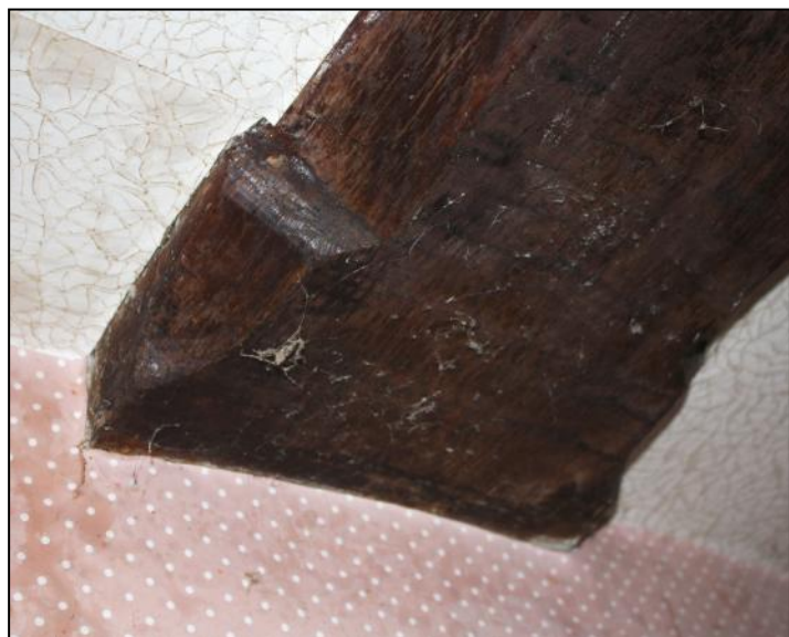
Plate 14: Decorative chamfer stops on a ceiling beam in Bedroom 4.
