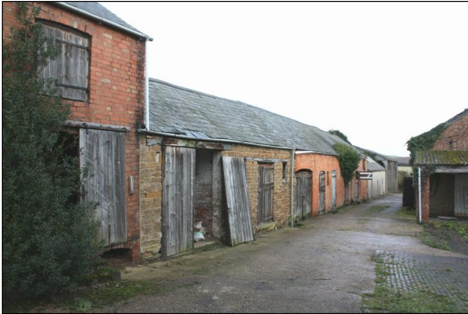
Plate 33: North row of brick and stone-built outhouses / farm buildings.
