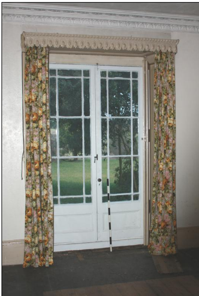
Plate 22: Doorway to garden with margin glazing in the Drawing Room in the later south wing of Parkfield House.
