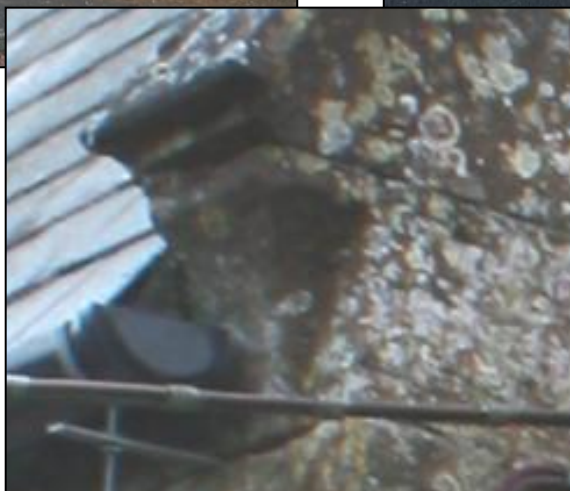
Plate 9: One of the two moulded kneeler stones at the north gable end.
