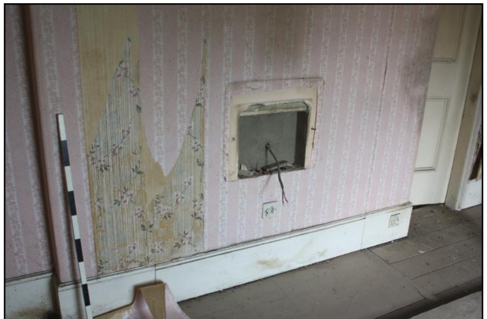
Plate 52: Possible surviving section of early 19th century wallpaper exposed in bedroom on first floor level of the Phase 4 south wing (to right of scale).
