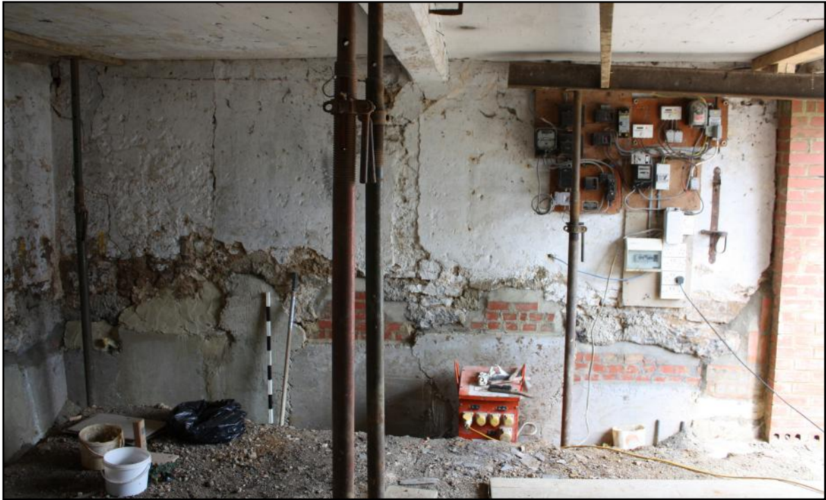
Plate 37: North end wall seen from the interior with new brick patching where the walling had deteriorated and in places found to contain soil.
