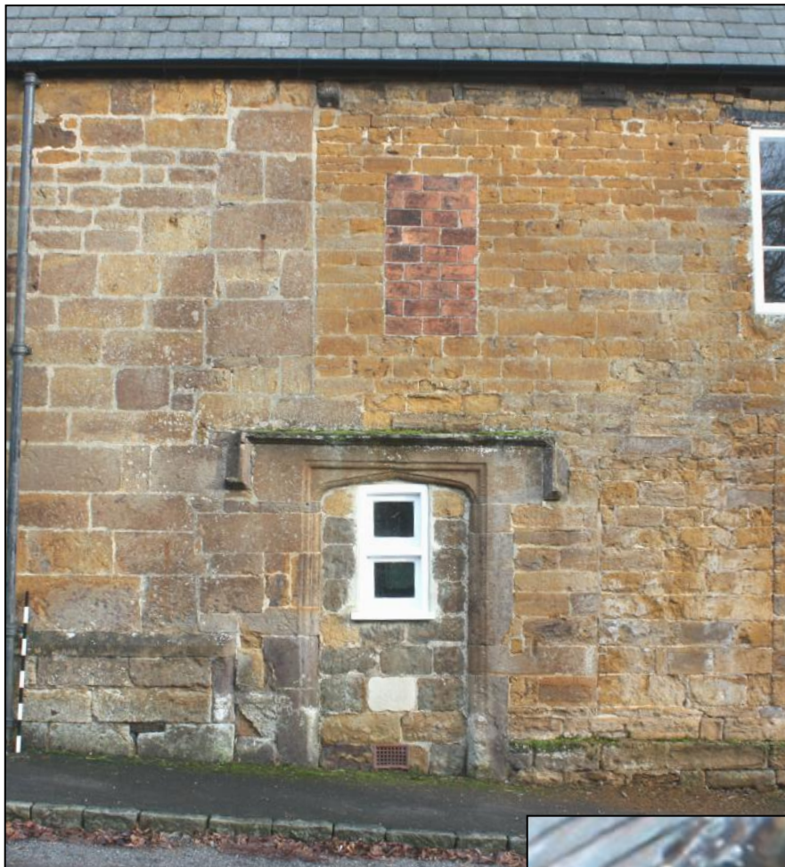
Plate 6: Infilled 17th century moulded doorway, stone plinths and straight joint above doorway on Nether Street frontage.
