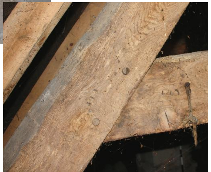
Plate 21: Matching carpenters' marks III showing on truss 2 in Attic 2.
