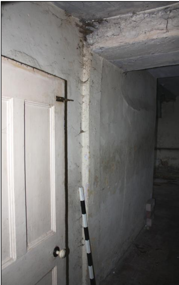
Plate 43: Timber post for doorway set into side walling above possible entrance threshold stone.
