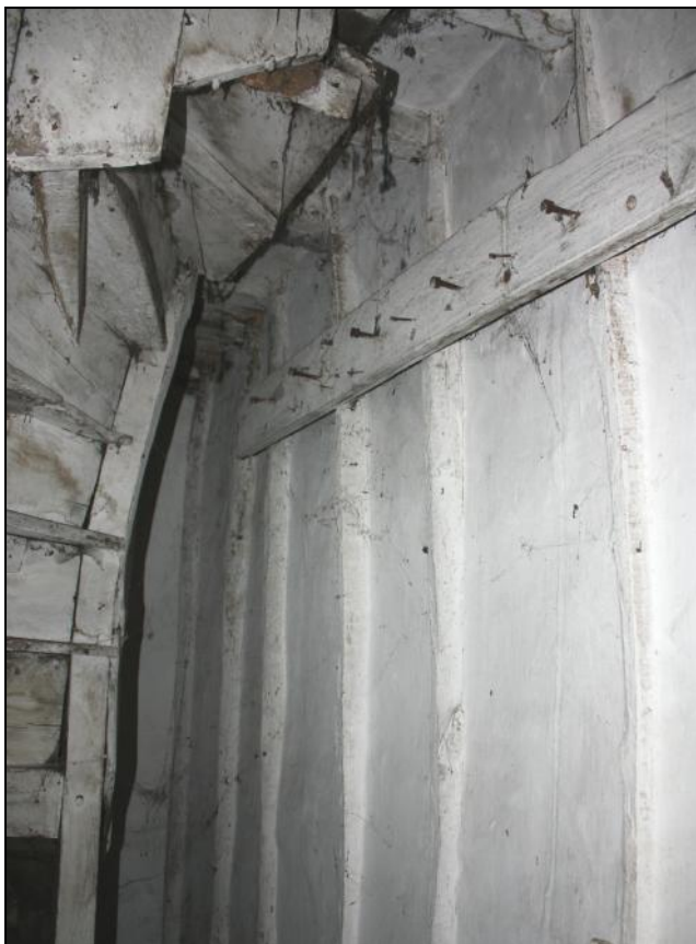
Plate 13: Narrow cupboard to Bedroom 4 with stud walling and the back of the staircase to the attic.
