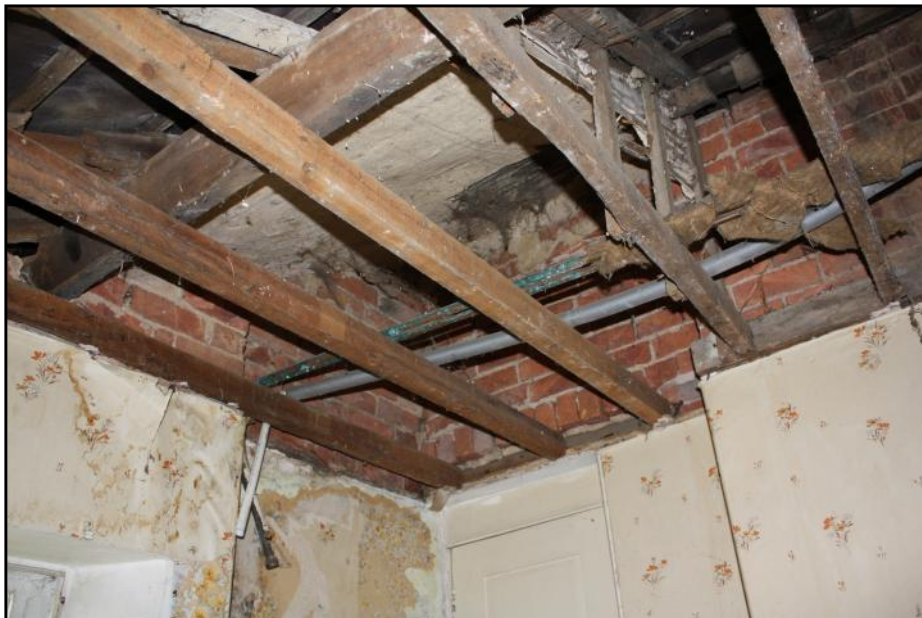
Plate 51: Internal brick walling showing in the Phase 4 south wing.
