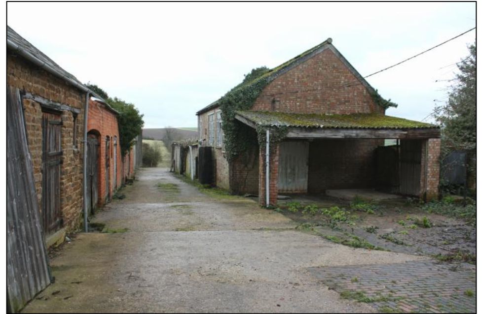
Plate 34: North and south rows of outhouses / farm buildings.
