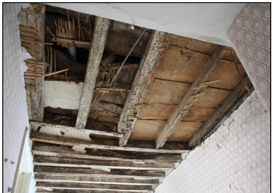
Plate 47: Change in direction of timber joists where a staircase may originally have risen to the garret of the Phase 2 building.
