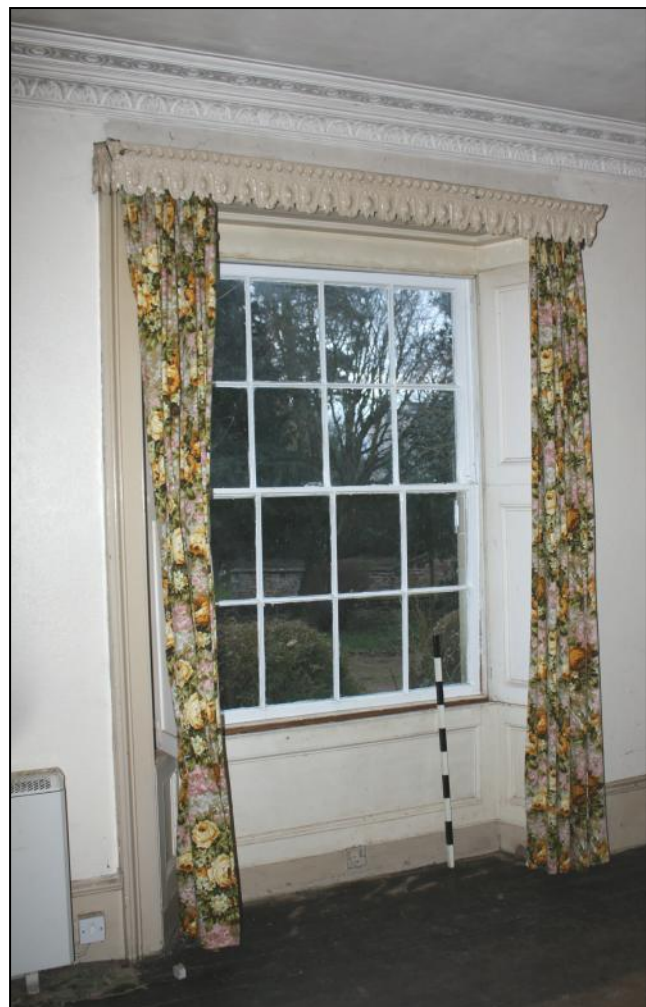
Plate 23: Late Georgian / Regency style 16-pane sash windows in the Drawing Room.
