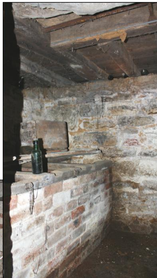
▲ Plate 32: Secondary mainly stone-lined cellar below the Drawing Room.
