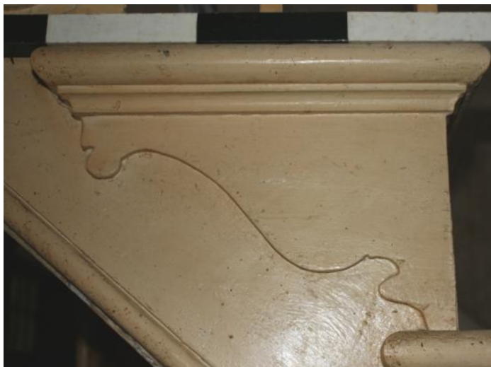
Plate 30: Curvi-linear design of probable early 19th century date at the end of the treads of the staircase.
