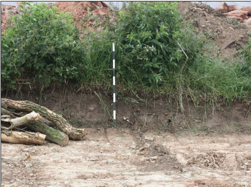
Plate 7: Section at side of a bund near top of south-west slope where topsoil and subsoil was of relatively shallow depth.
