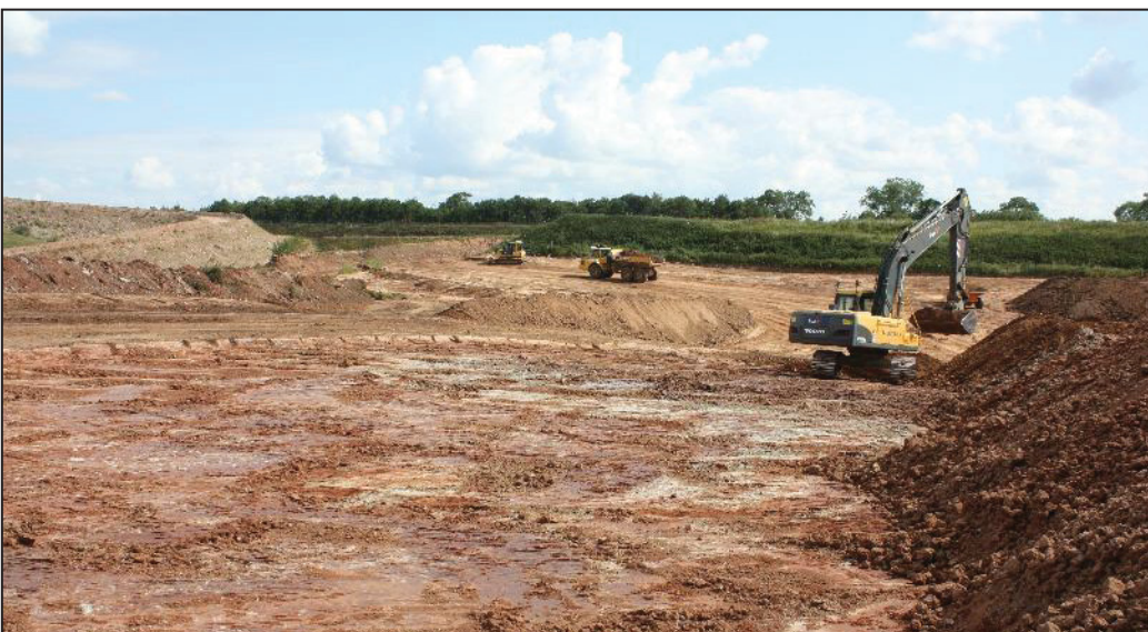
Plate 3: Later view with second-stage subsoil stripping underway across the site.
