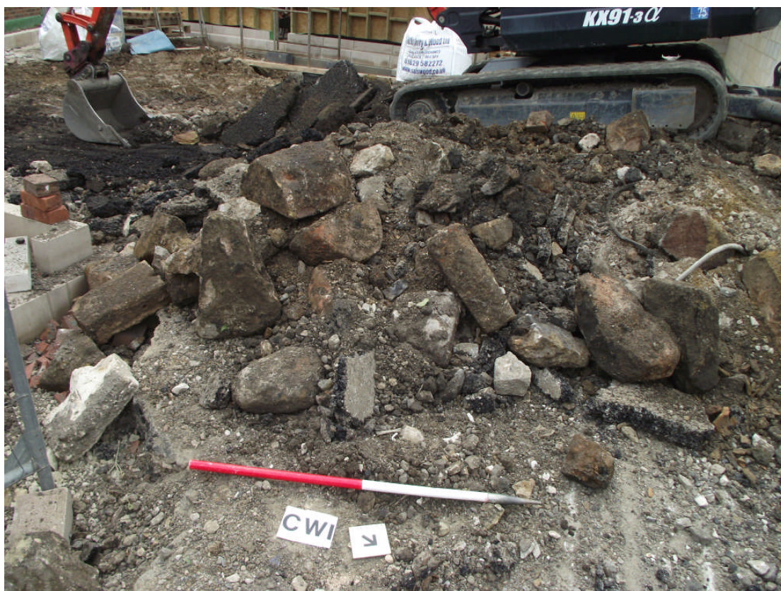
PLATE 14. Area 07. Stones from demolished boundary wall in 0009. Looking west.
