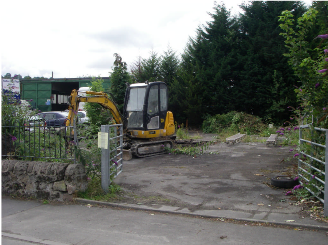
PLATE 1. Site prior to trial trenching. Looking south west.
