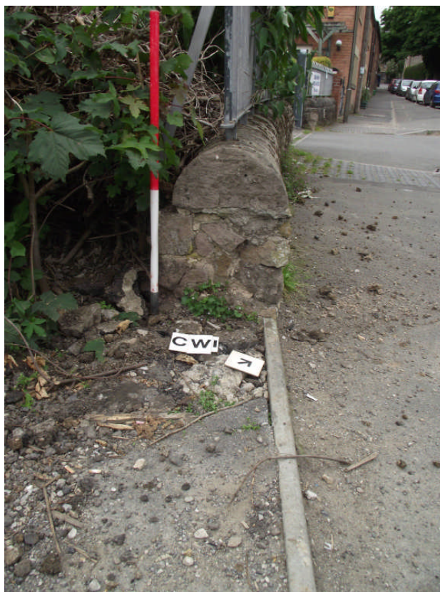
PLATE 15. Area 07. Existing boundary wall and entrance. Looking north west.
