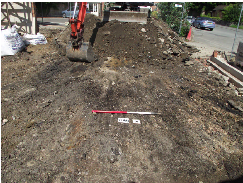
PLATE 13. Area 07 with 0001 removed. Looking north west.
