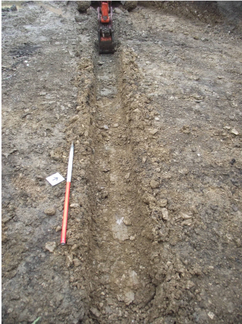
PLATE 9. Service trench cut into base of Area 04. Looking north west.
