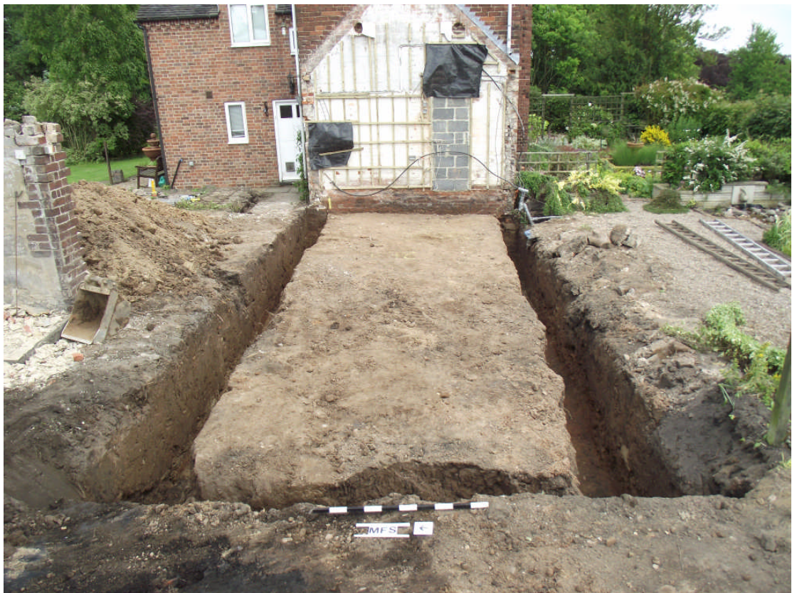
PLATE 5. View of completed ground works. Looking east.
