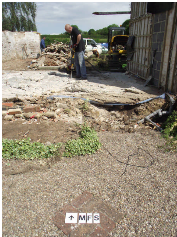
PLATE 3. 0001 being broken up prior to removal Looking north.
