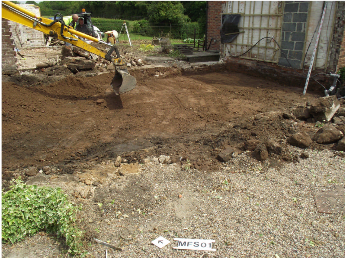
PLATE 4. Ground in Areas 01 and 02 being reduced to formation. Looking north east.
