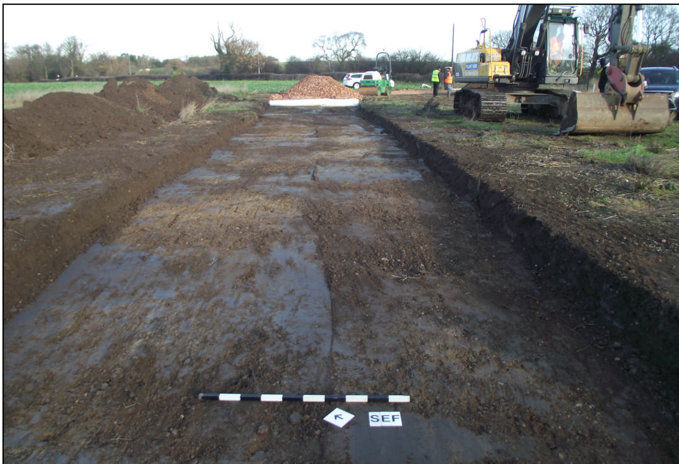
Plate 3: Area 02, Topsoil strip for the new access road, looking North East
