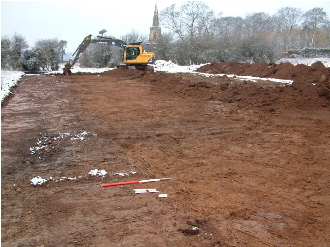
PLATE 2. Machine stripping in Area 02. The fill of the original pipe trench is on the left Looking south west.
