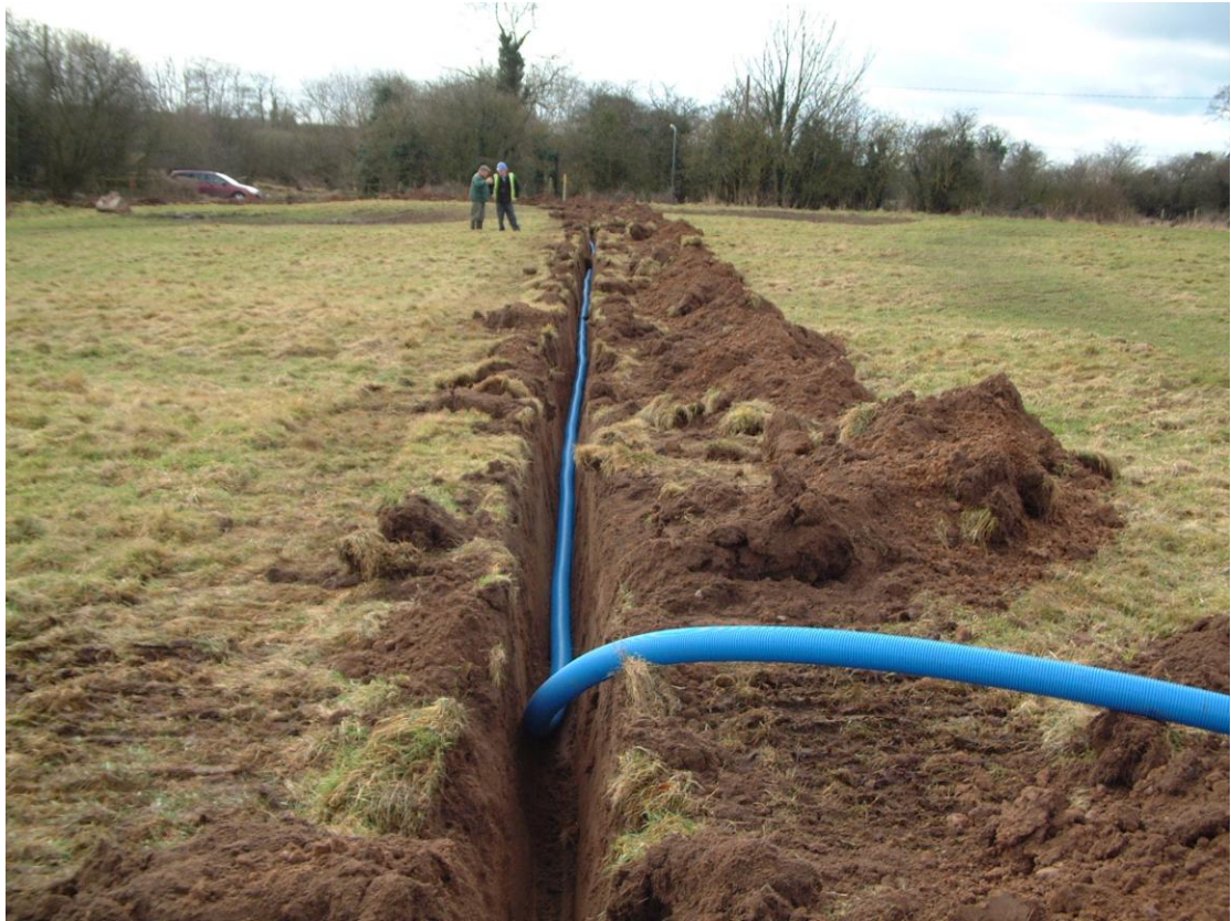
PLATE 1. The pre-drainage pipe in Area 02. Looking north east.
