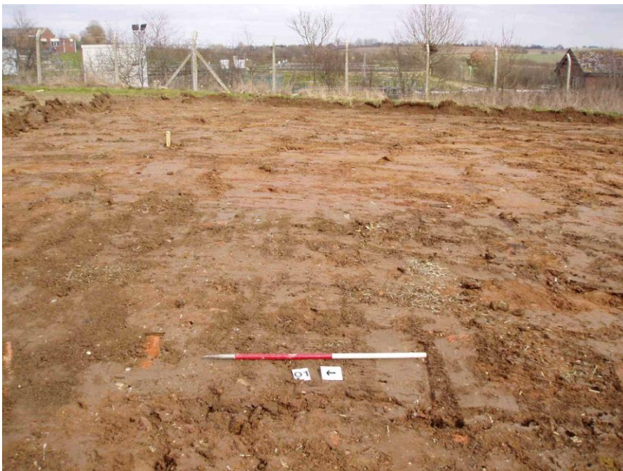
Plate 2 North east corner of Area 01 after topsoil stripping showing brick rubble in the subsoil, 0002. Looking east.
