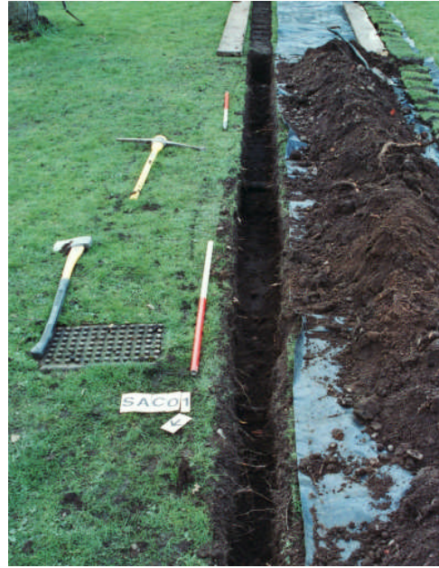
Plate 2: Area 01. Looking south.
