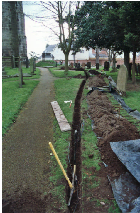
Plate 6: Area 03. Looking south.
