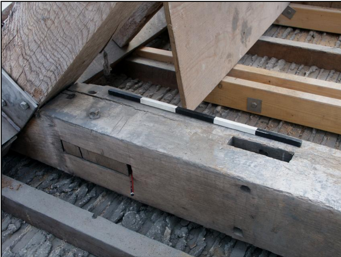
Plates showing Apethorpe Hall. 27: one of a sequence of ten large collars set between principal rafters with mortices that indicate reuse from elsewhere (photo 625); 28: an example of close-set mortices in one of the larger collars. The acute angle of the mortice with the intact tenon is indicated by a projecting pencil (photo 611).
