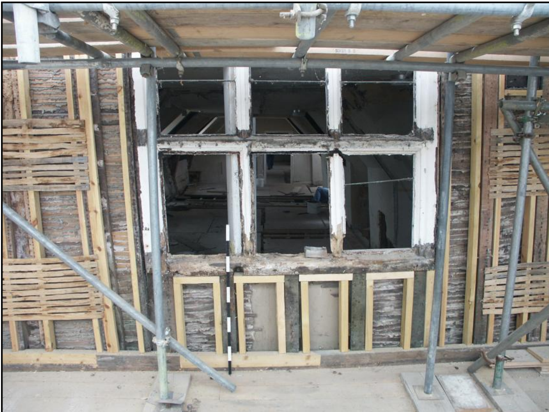
Plates of the East Range of Apethorpe Hall. 39: wooden-framed window in the south end-wall of the attic, with part of the frame of an earlier larger 6-light window showing to the right and above (photo 284); 40: a 6-light wooden-framed window in the north-end wall of the attic (photo 265).
