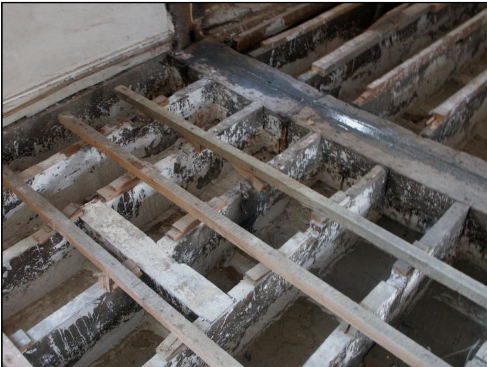
Plates of the East Range of Apethorpe Hall. 49: one of the surviving pieces of sleeper beam under the floor of the attic that may have supported a corridor partition wall, here indicated by the arrow (photo 718); 50: one of several short cross-pieces along the line of the supposed corridor where the sleeper beams were absent (photo 720).
