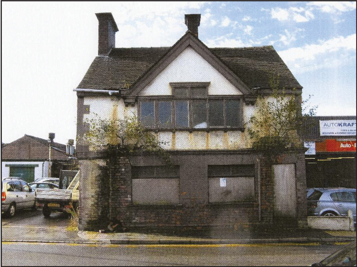
Plate 3: North frontage of 124 Uttoxeter Road, Longton before scaffolding was erected around the building.
