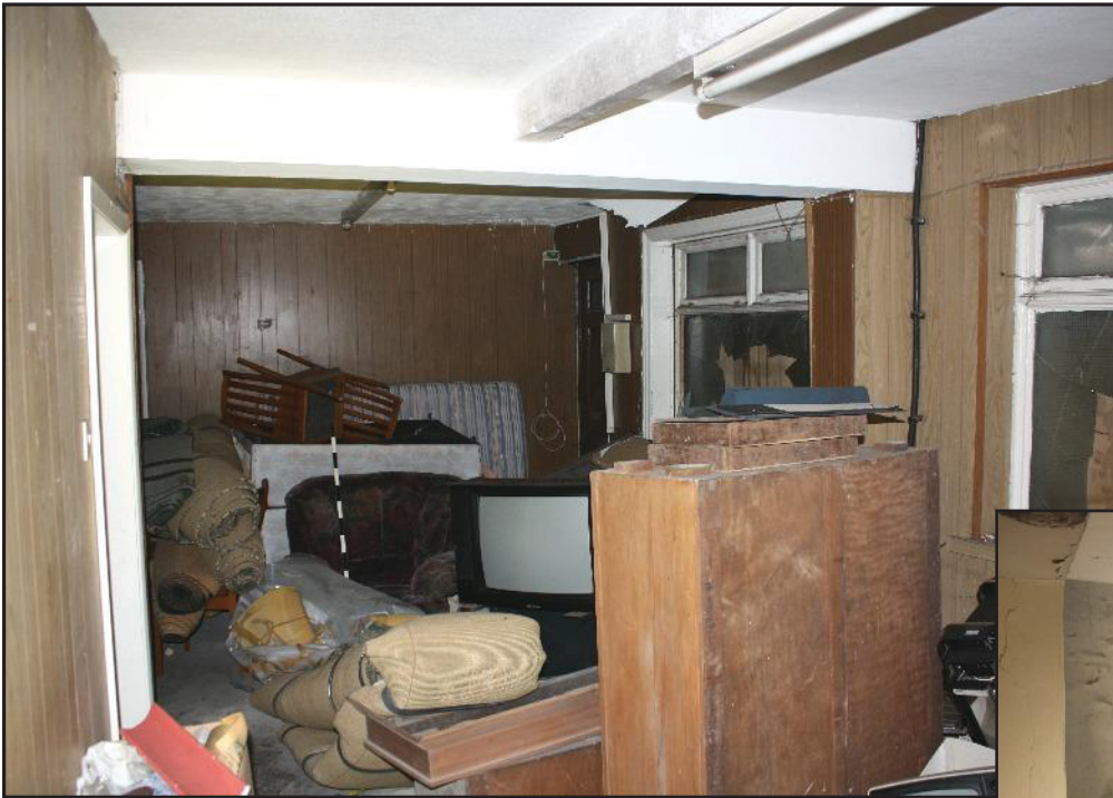
Plate 10: View looking across Rooms 1A and 1B with panelling on walls showing. 1m scale shown.
