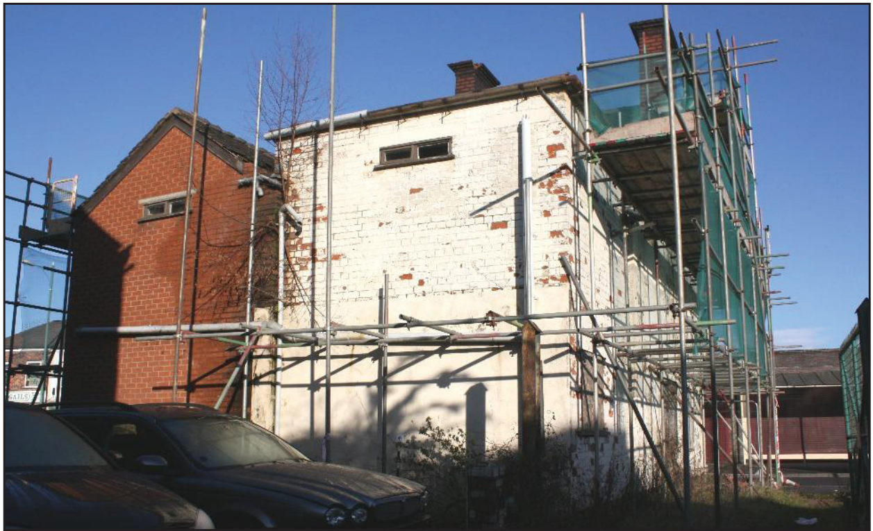
Plate 8: South elevation of 124 Uttoxeter Road, Longton showing a rebuilt gable end wall to left and a flat-roofed, slightly recessed part to right.
