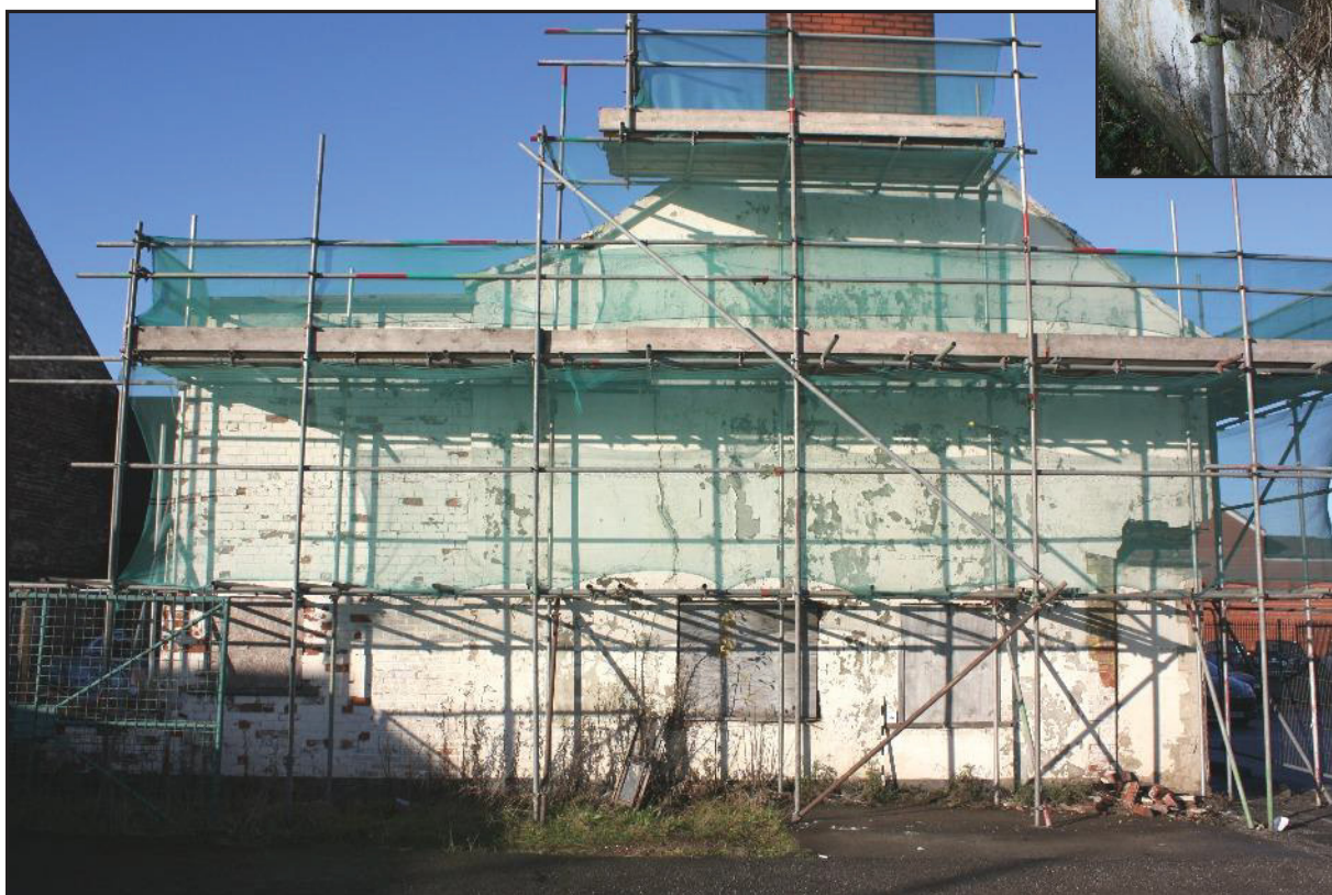
Plate 7: East elevation of 124 Uttoxeter Road, Longton. 1m scale shown.
