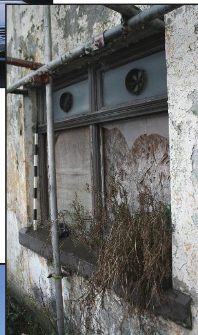
Plate 6: Detail of window showing to centre in Plate 5. 1m scale shown.
