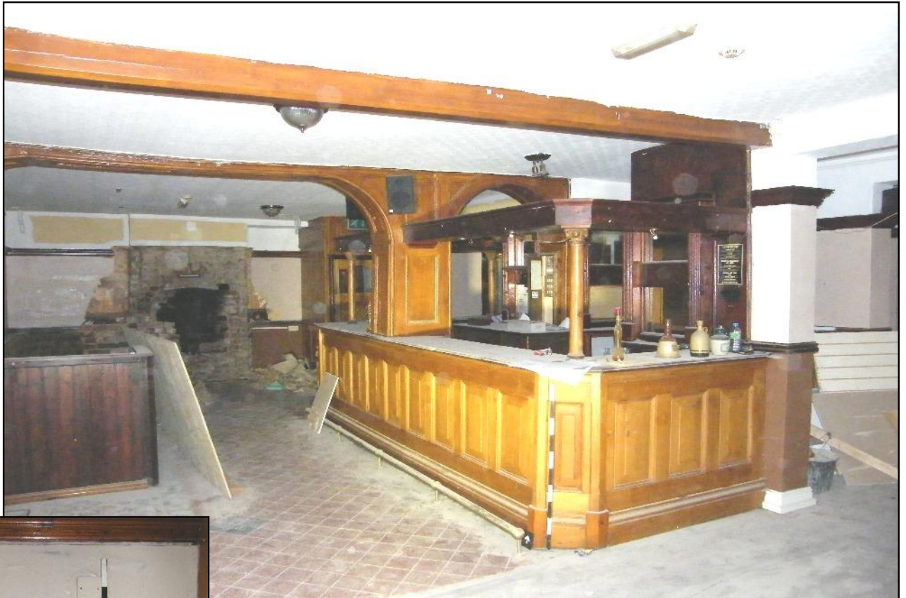
Plate 6: View of bar in Room 2, with position of removed kitchen range of former Room 3 showing in background.
