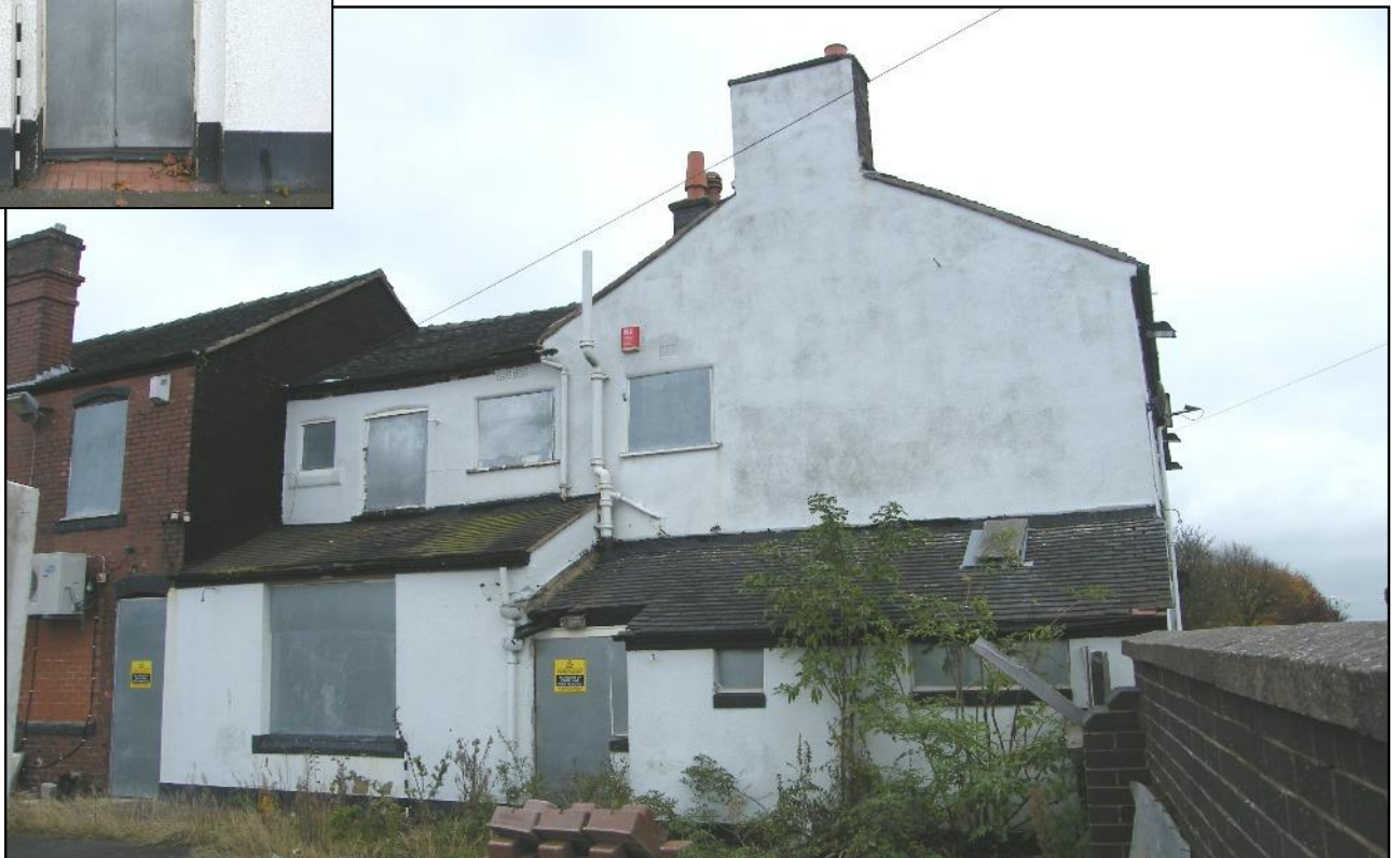
Plate 5: Rear view of the Red Lion public house showing the added middle range (in centre) and its extended lower room, a toilet block (lower right) and part of the function room block (brick showing, far left).
