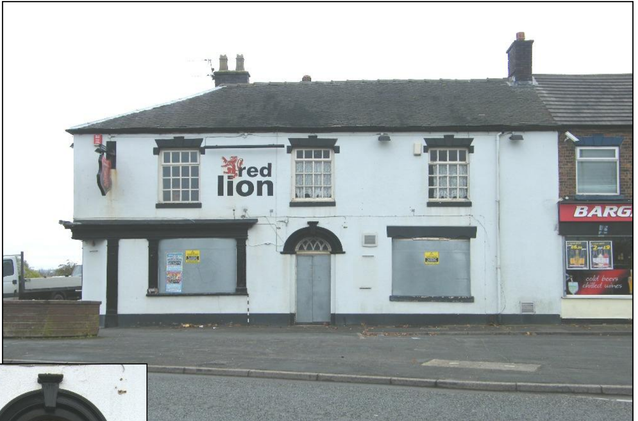
Plate 3: Symmetrical arrangement of door and window openings on the east frontage.
