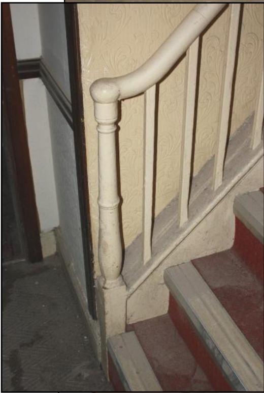
Plate 13: Newel post of staircase.
