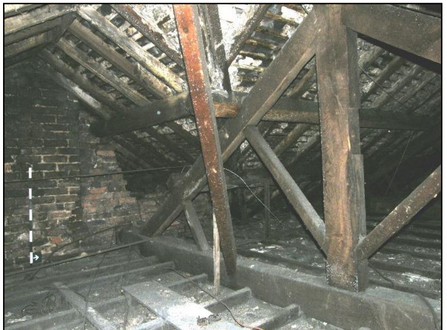
Plate 22: East Roof, Truss 2, viewed looking north-west.
