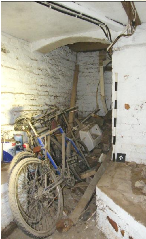
Plate 16: View of Cellar 3, with rear part that underlies the adjacent property.
