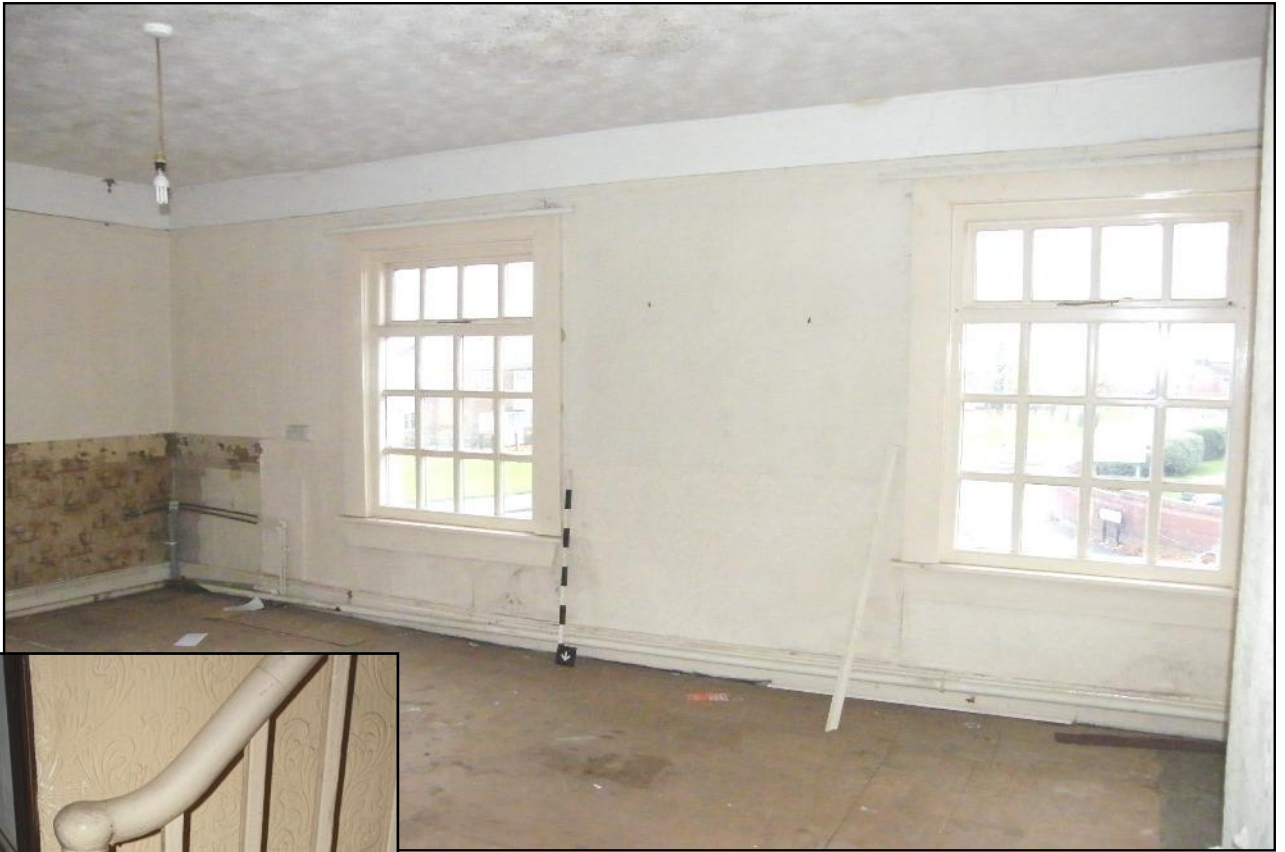
Plate 12: View of windows and exposed wallpaper in Room 11.
