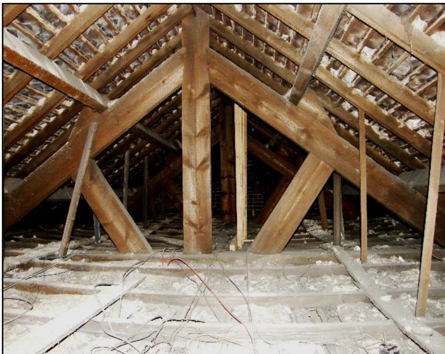
Plate 18: North-west Roof, Truss 1, viewed looking north.
