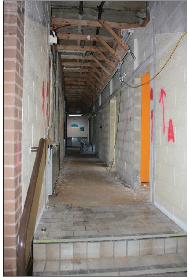
Plate 23: Corridor with pipework showing above timber joists and bracing.
