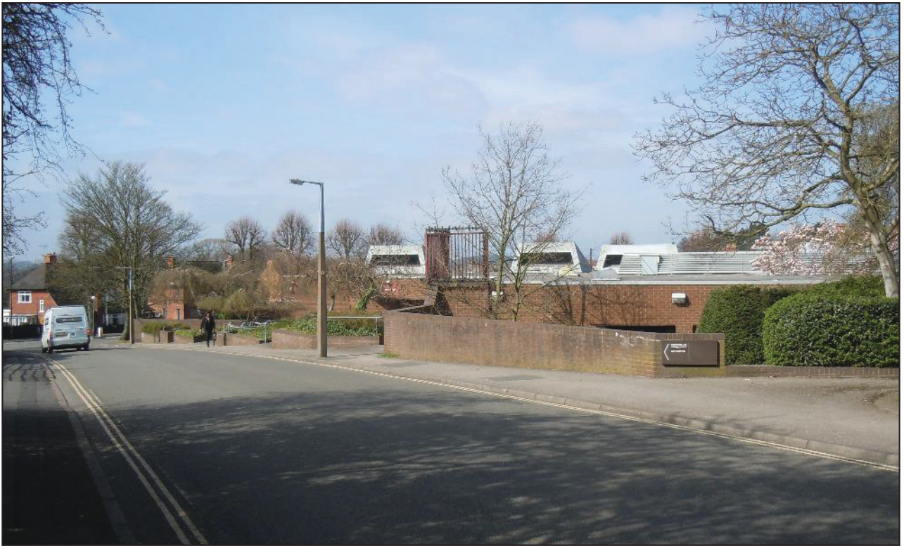
Plate 1: View of the Ilkeston Magistrates' Court House looking westwards along Pimlico. This view shows the raised roof structures over the courtrooms and, to right, the upper plant room.
