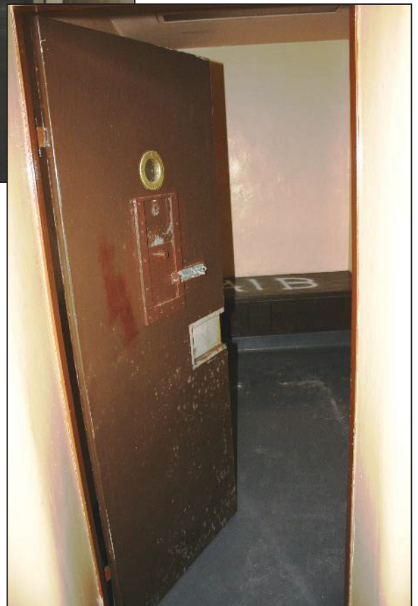
Plate 20: One of the cells, showing standard fitted bench to the rear.
