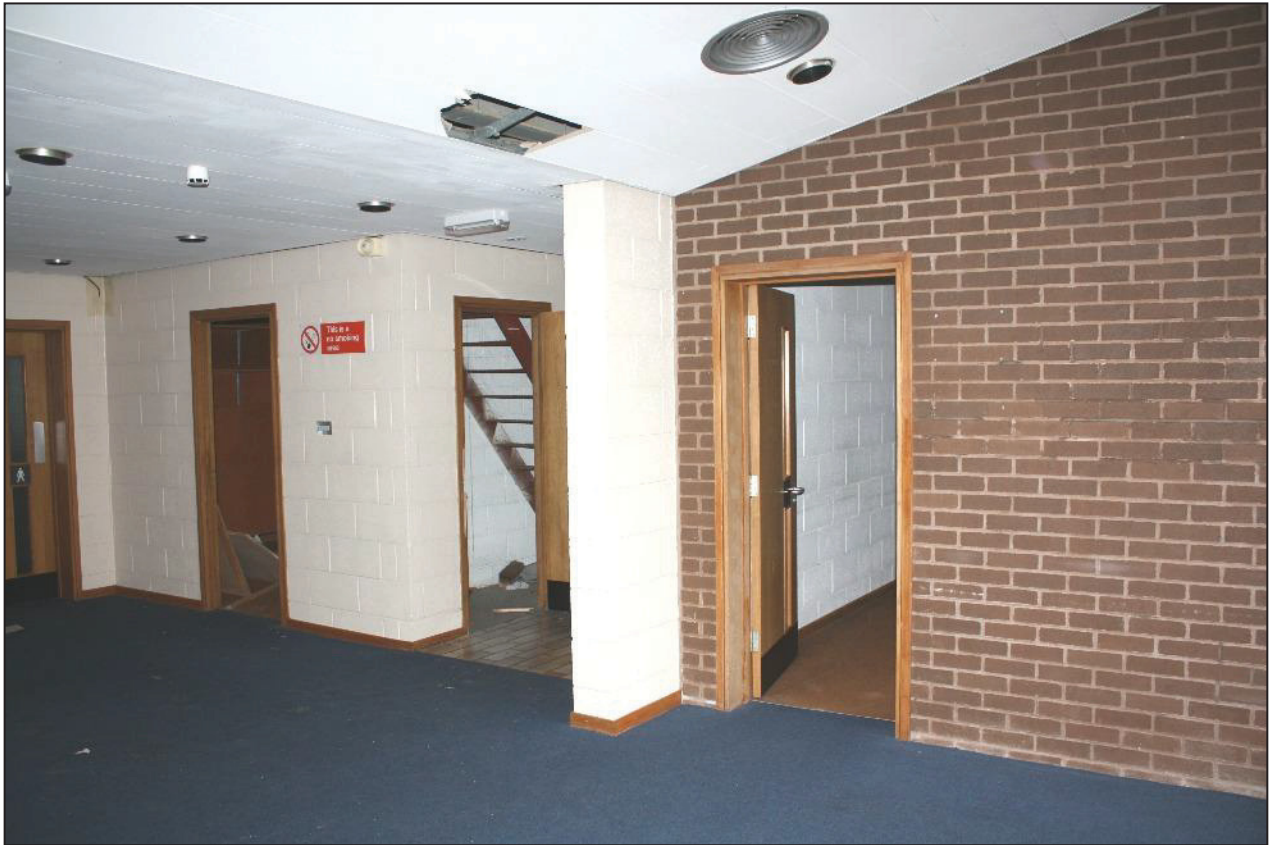
Plate 11: Contrasting brick and white blockwork finishes. The staircase in the middle leads to the upper plant area.
