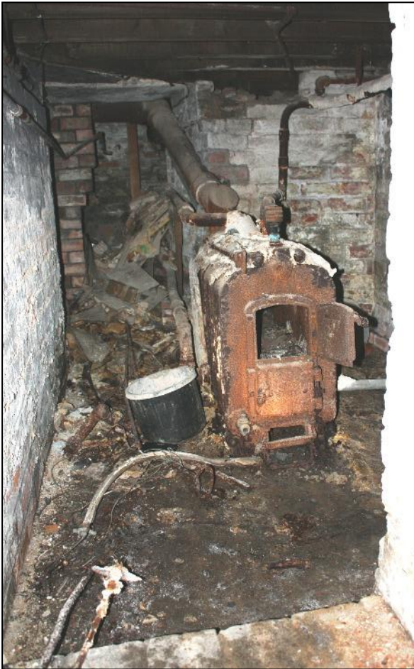
Plate 18: Old stove in Cellar 2 beneath unit G, No. 201 High Street.
