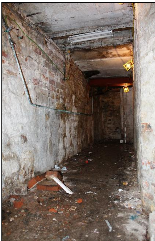
Plate 11: Passageway to Cellar 1 beneath No. 200 High Street, with walling built from both stone and brickwork.
