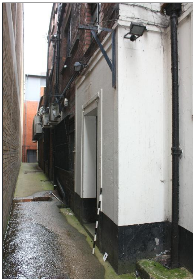
Plate 3: View along narrow side alley running between Nos. 199 and 200 High Street.
