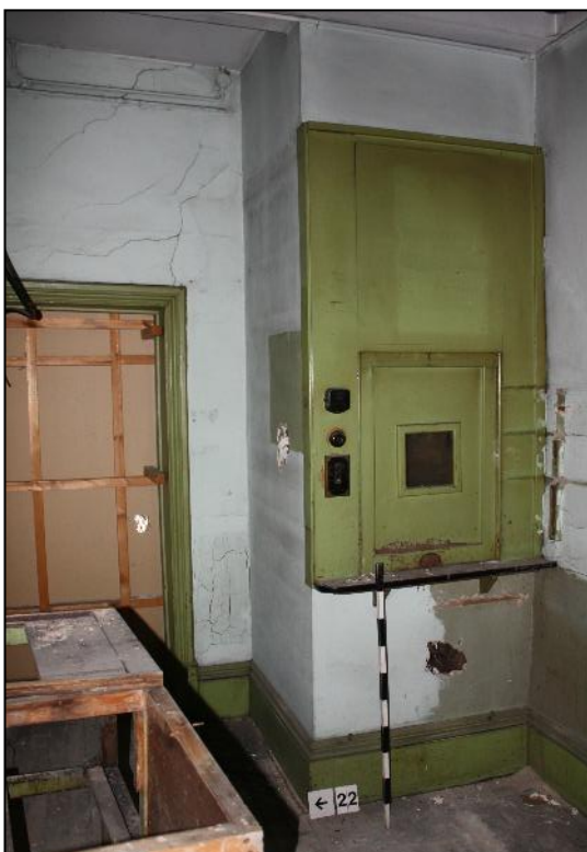
Plate 33: Dumb-waiter lift at east end of unit G and, to left, blocked access to unit E.
