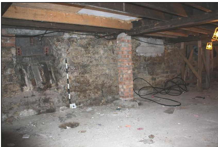
Plate 13: South side of Cellar 1, showing walling built mainly with stone.
