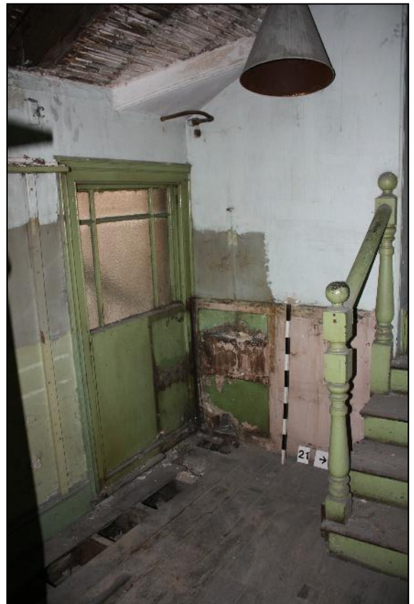
Plate 32: Possible former doorway access from the first floor unit G to an enclosed gully.
