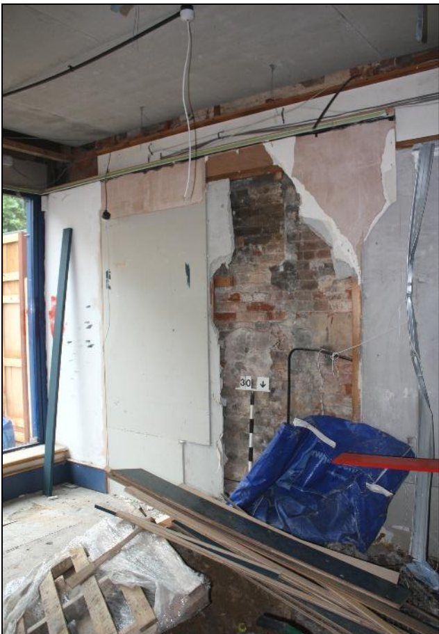
Plate 16: South wall of unit D with brickwork revealed under plasterwork.
