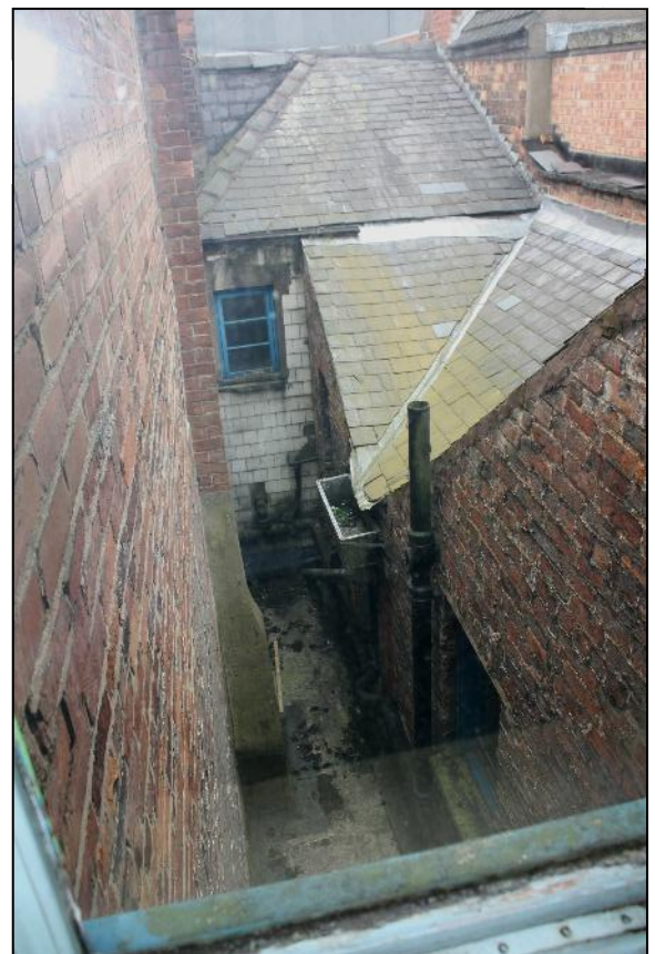
Plate 37: View of enclosed gully seen from second floor window.
