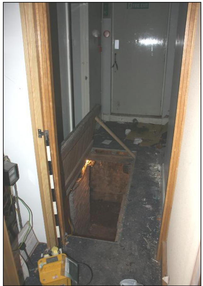
Plate 17: Staircase in unit C down to passageway in Cellar 1.
