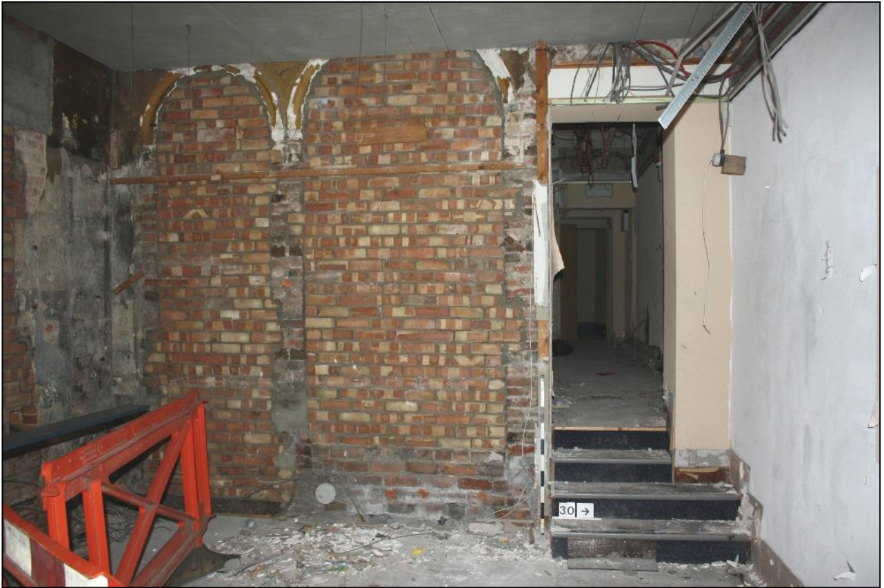
Plate 15: Ground floor area of unit D in No. 200 High Street, Lincoln, with infilled arched recesses revealed in west end wall.
