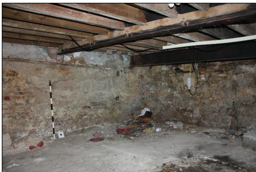
Plate 14: View of north-east corner of Cellar 1 with bricks showing beneath plasterwork.
