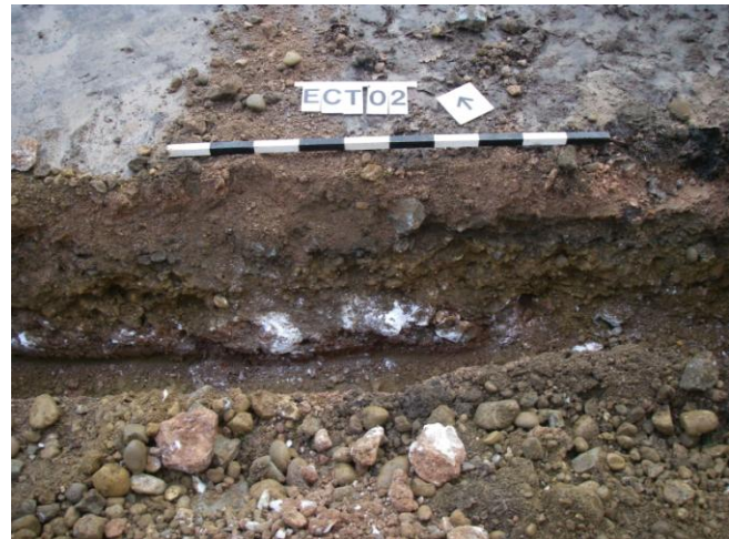
Plate 02. Marble rocks in lowest levels of road makeup. Looking north east.
