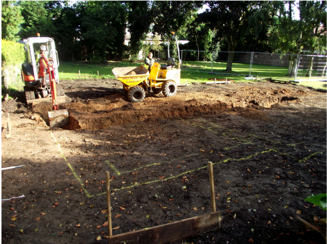
Plate 1. Trenching on site. Looking north east.
