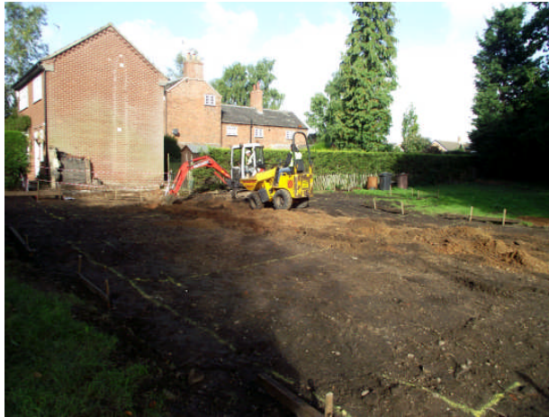
Ground works at Ten Ward Lane, Breaston.
