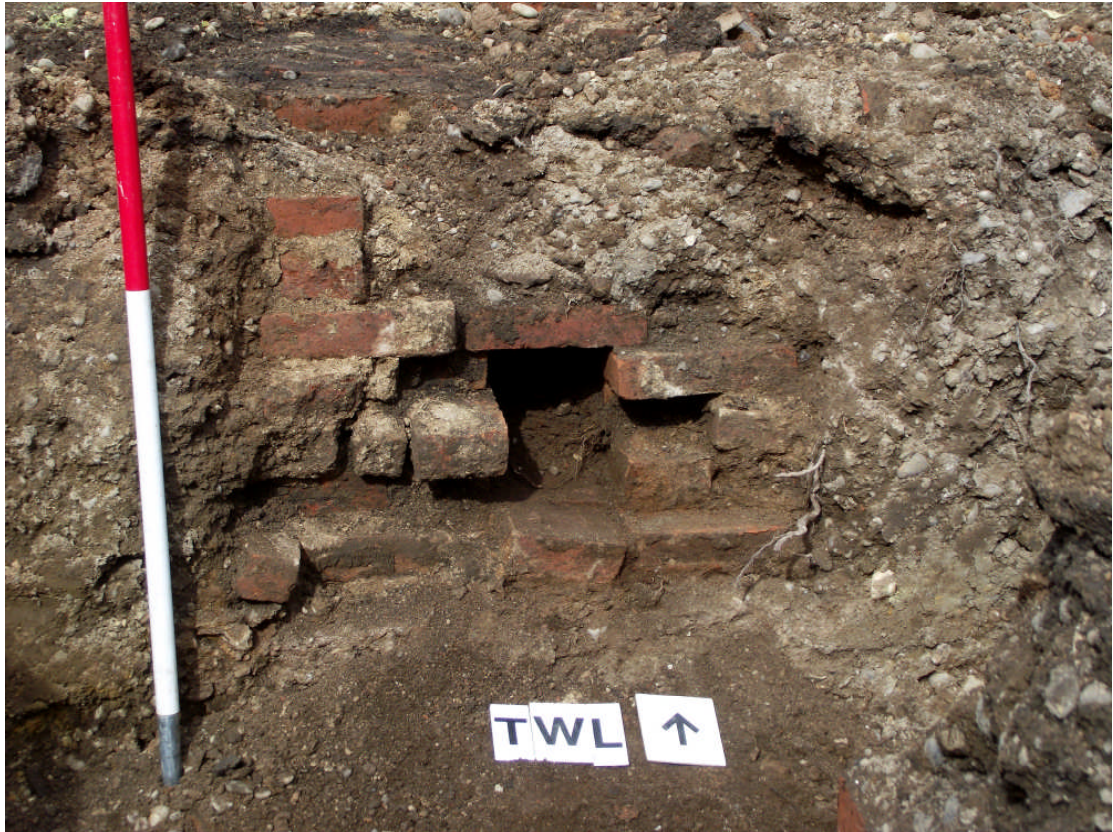
Plate 5. South facing section of brick culvert, 0006, at the junction of Area 01 and Area 13. Looking north.
