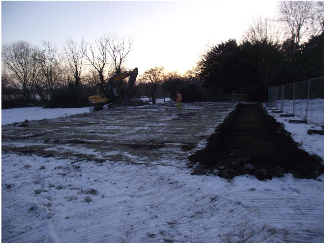
Plate 1. Start of the top soil strip. Looking west.
