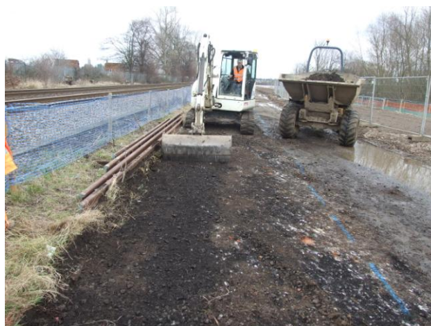
Excavating in Area 01 between the rail way and the haul road.
