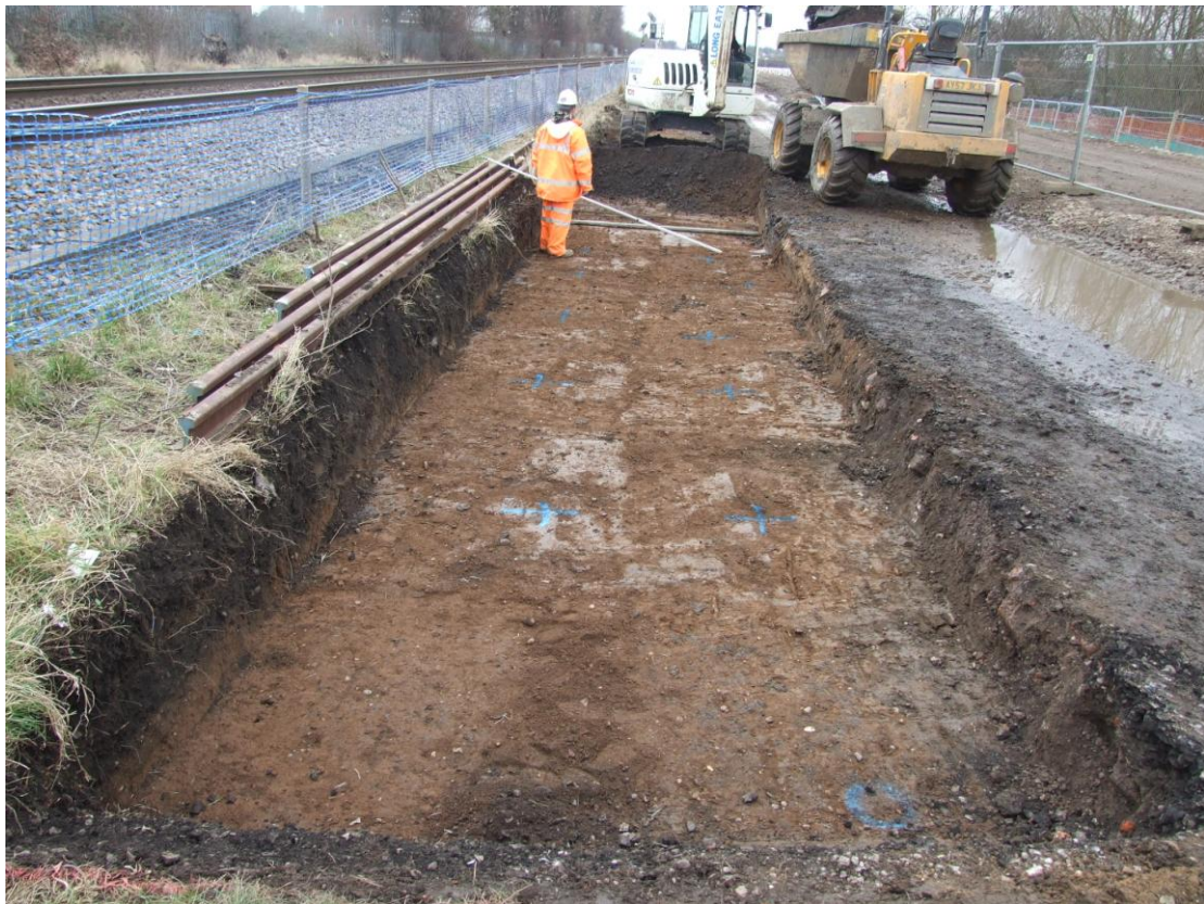
Plate 2. Stripping in the centre of Area 01. Looking north east.
