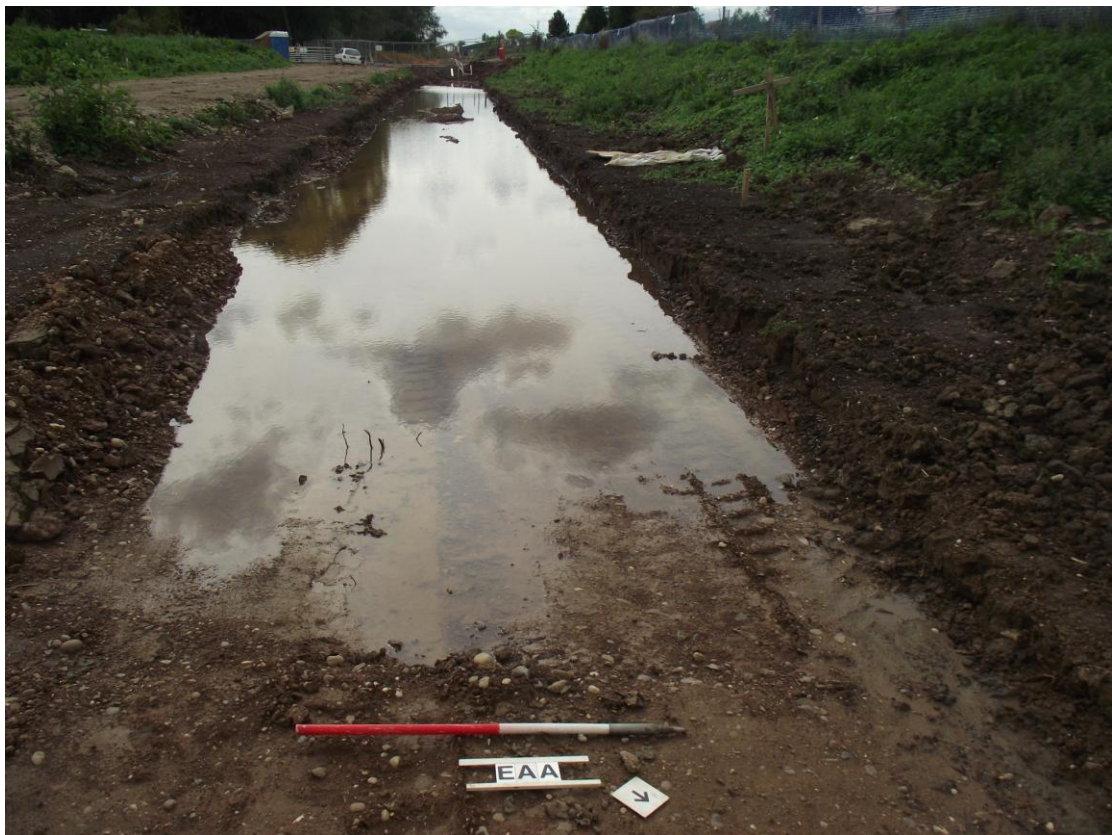
Plate 8. Area 03 flooding after topsoil strip. Looking north east.
