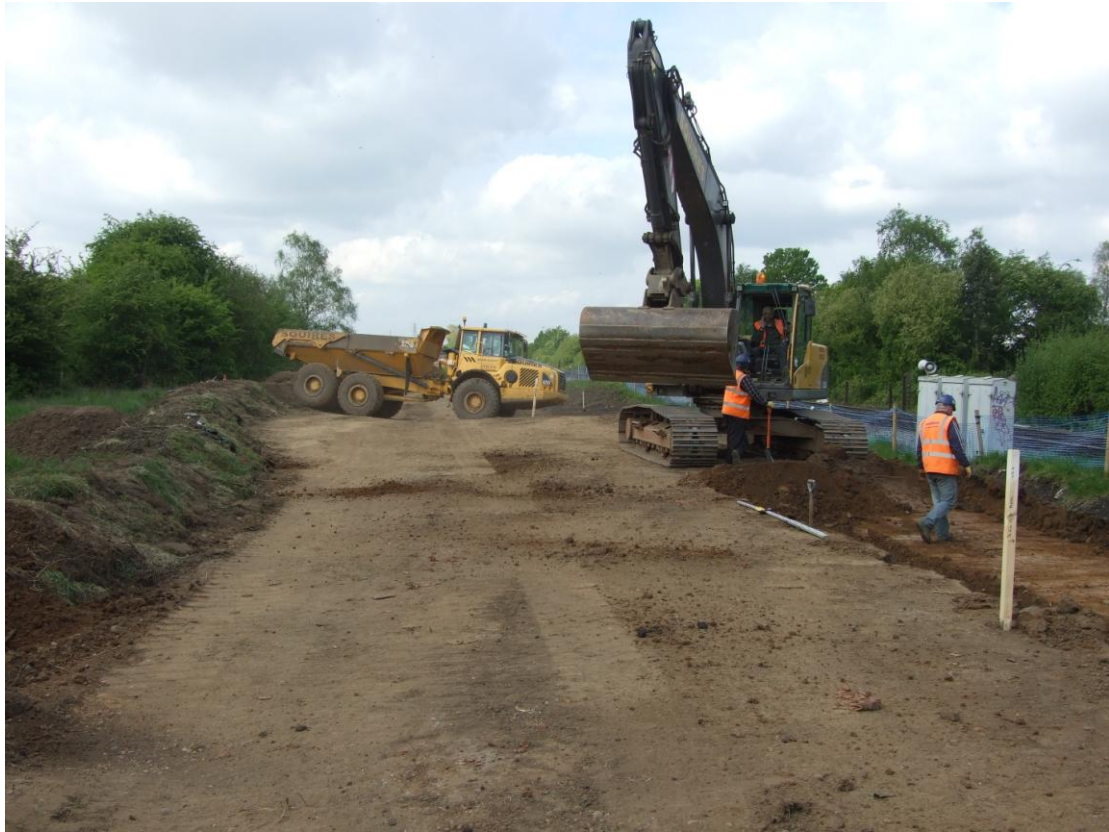
Plate 5. Soil stripping in Area 02. Looking north east.
