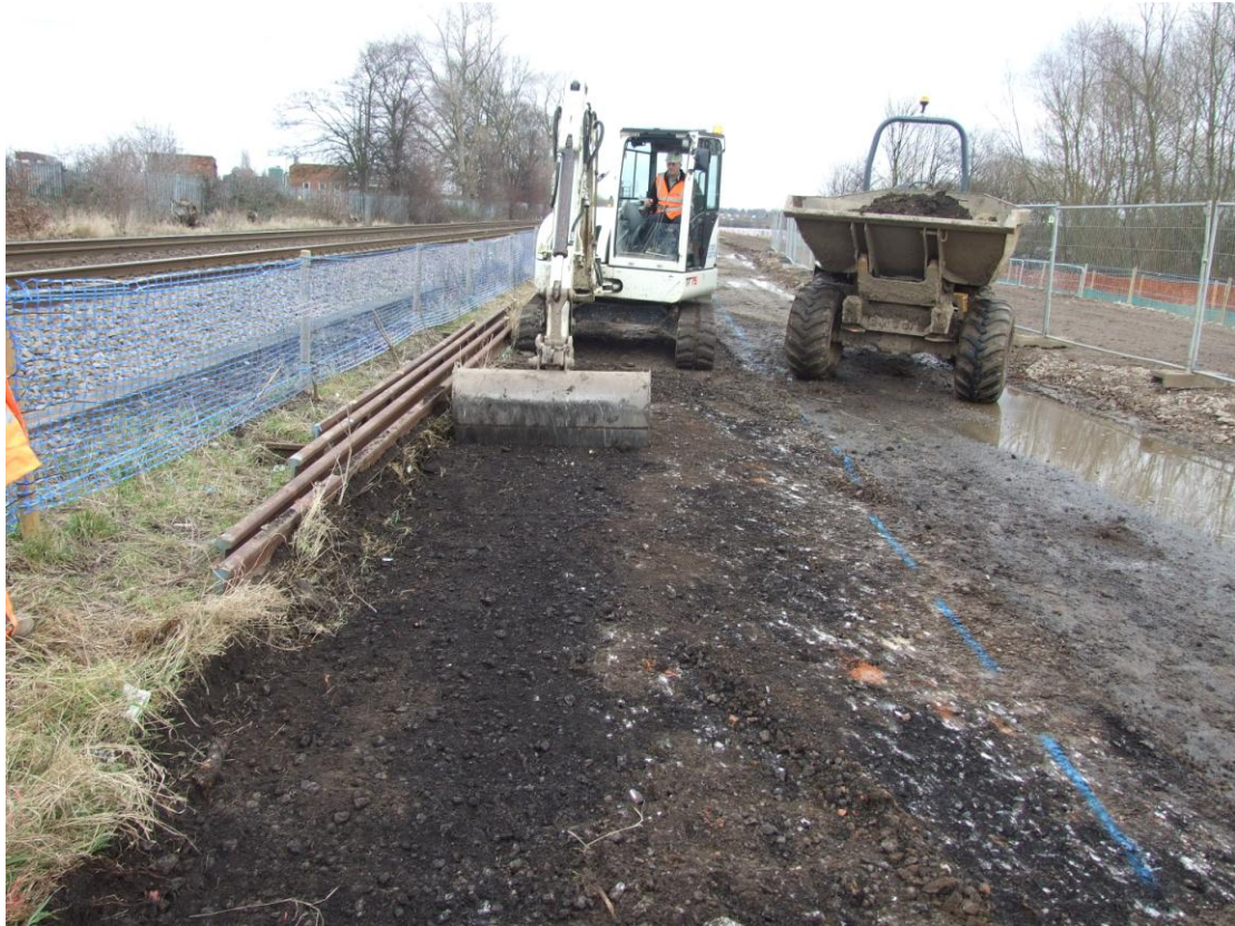
Plate 1. Stripping at the start of Area 01. Looking north east.
