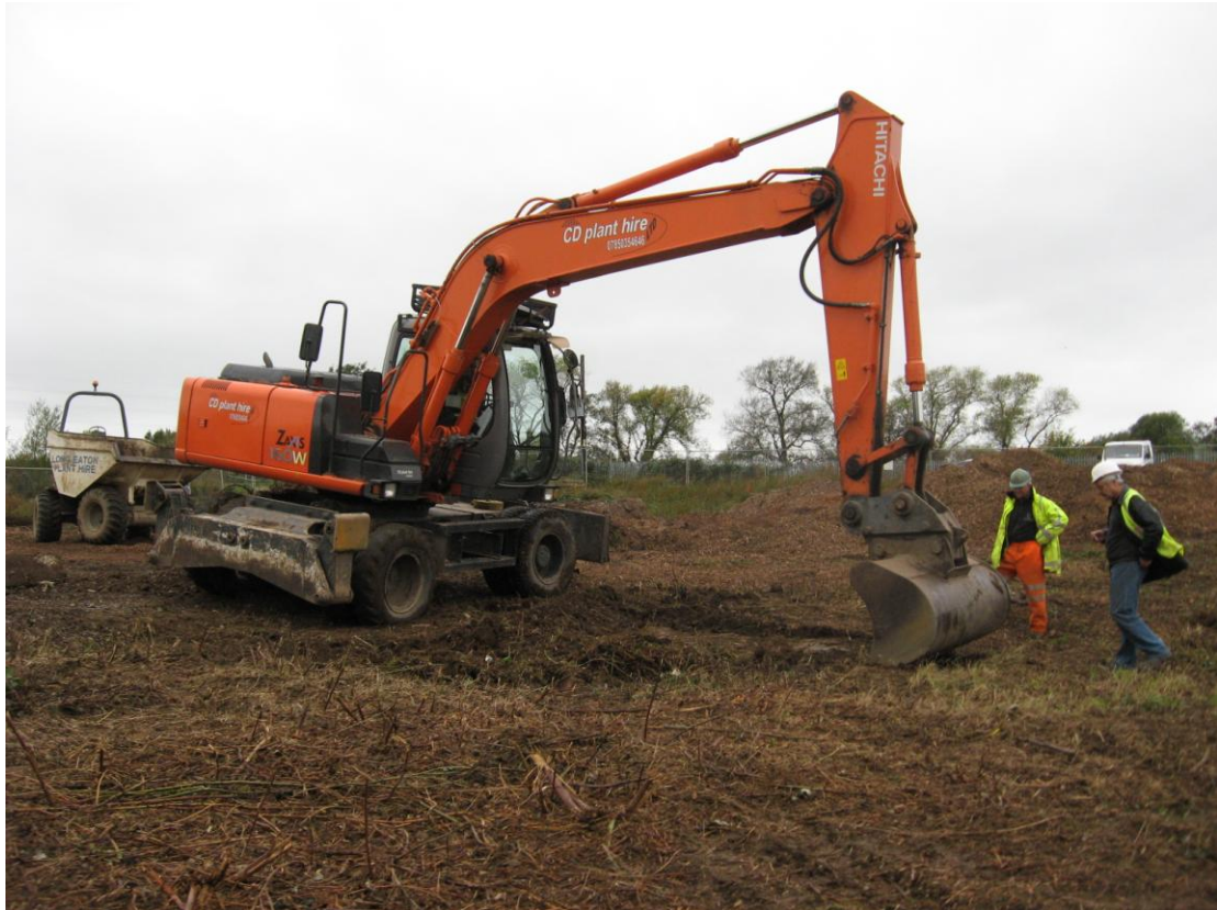
Plate 9. Start of soil stripping in Area 04. Looking west.
