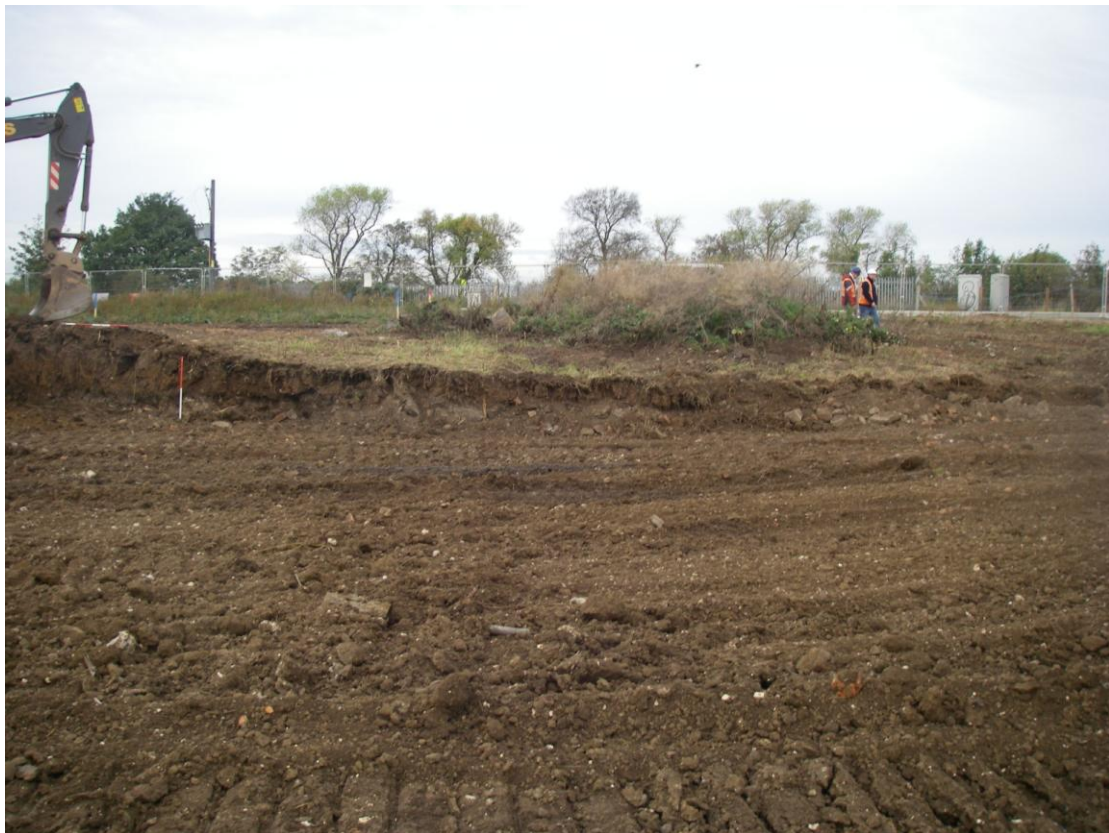
Plate 10. The surface after the upper layer has been removed. Looking west.
