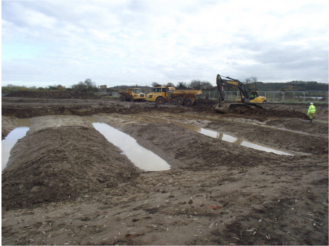
PLATE 3. Constructing the ridges. Looking north north-east.
