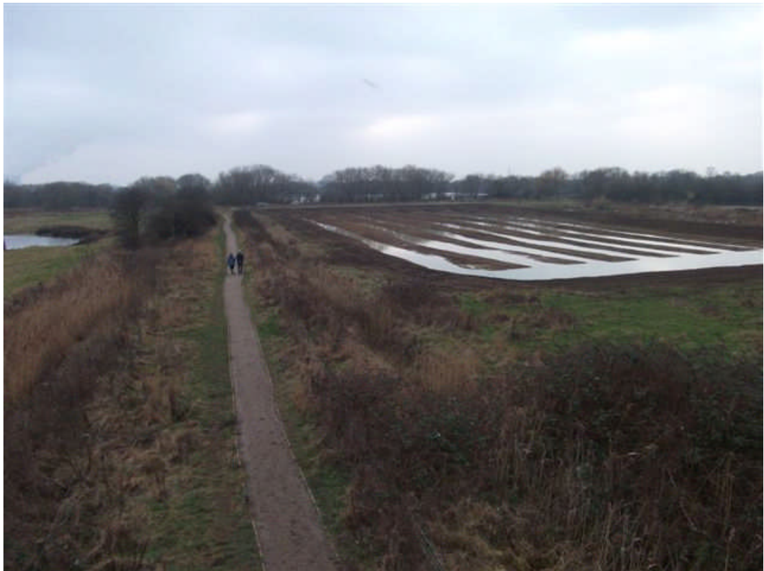
PLATE 4. The completed ridges. Looking southsouth-west.
