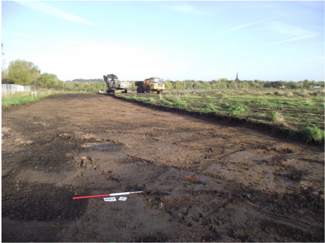
PLATE 1. Topsoil stripping at the south-west end of Wheatear field. Looking north-west.
