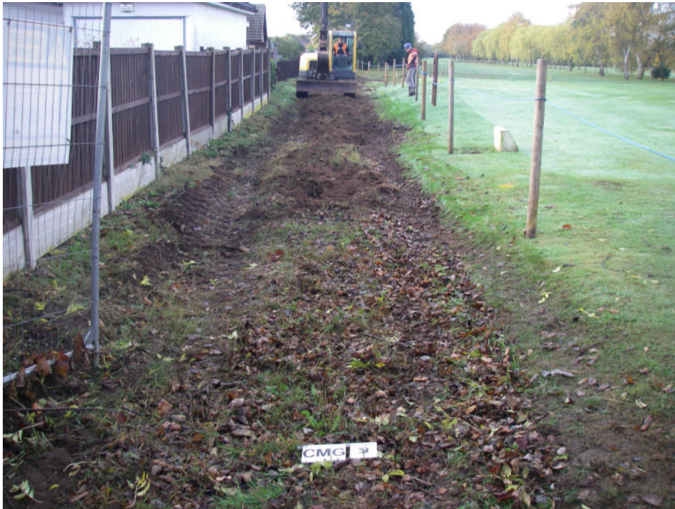
Plate 1. Tree stump removal at beginning of watching brief. Looking south west.
