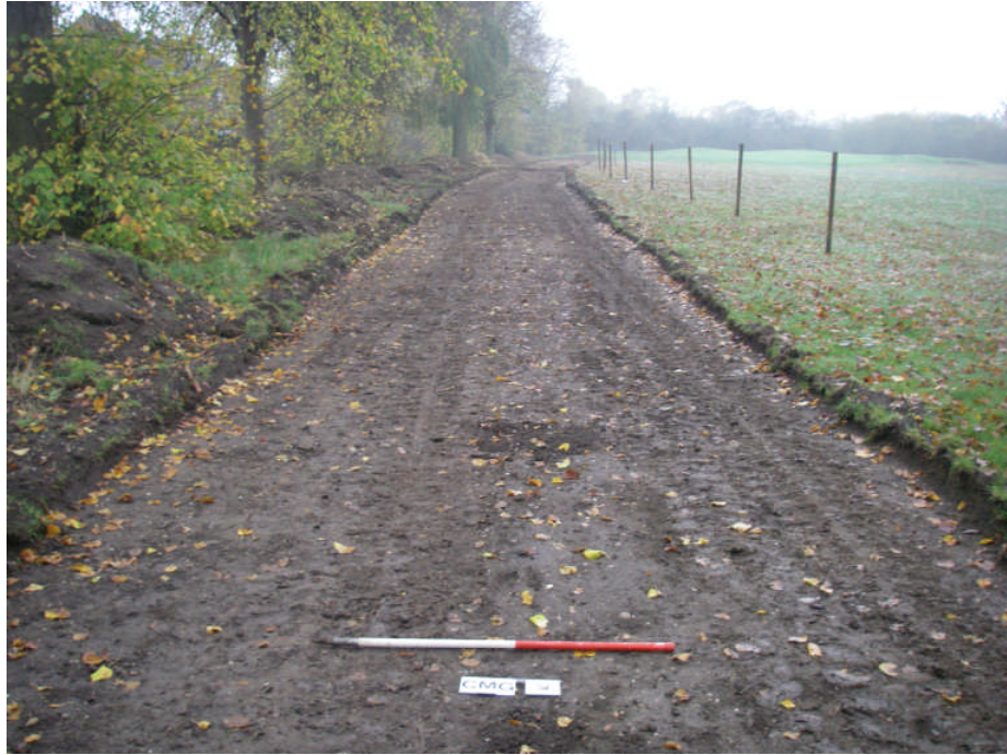
Plate 5. Topsoil stripping continued. Looking south west.
