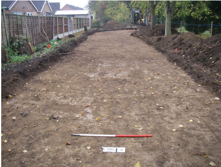
Plate 3. Topsoil stripping continued. Looking south west.
