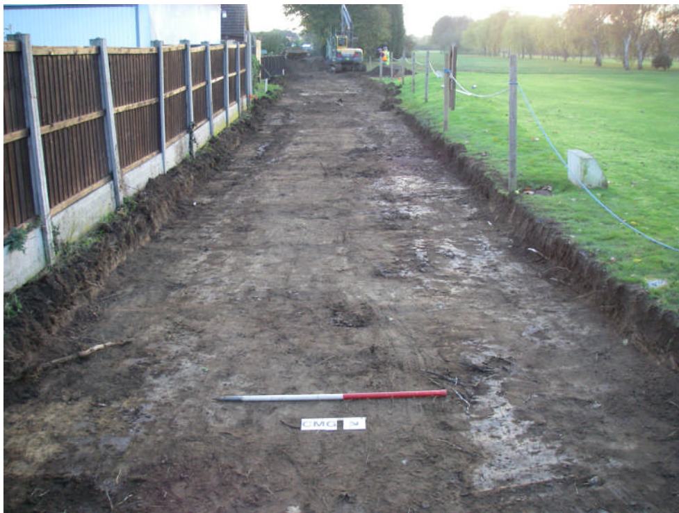
Plate 2. Topsoil removal from meadow lane end. Looking south west.
