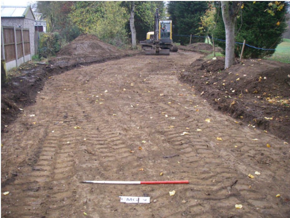
Plate 4. Topsoil stripping continued. Looking south west.
