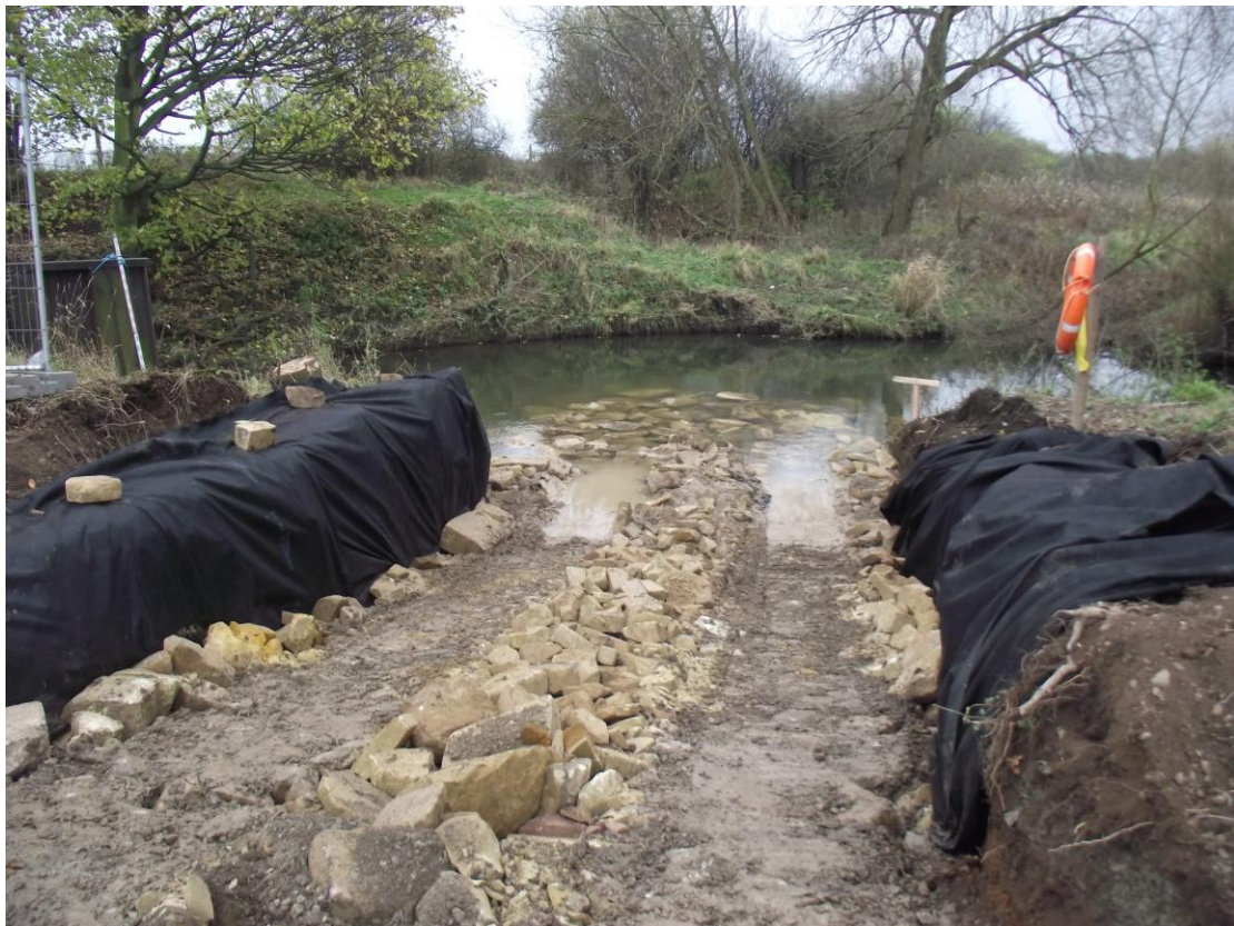
PLATE 5. Stone laid over the surface and into the river to construct a ford. Looking south west.
