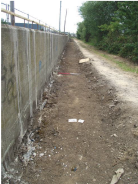
PLATE 7. Area 06 after top of flood defence stripped. Looking north-east.
