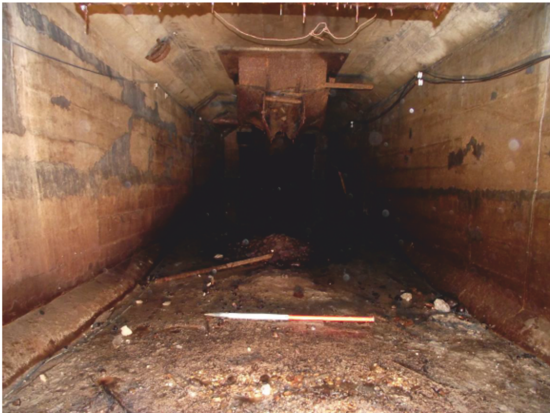
PLATE 8. Interior of concrete chamber, Area 04. Looking south-east.
