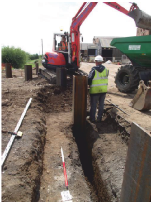
PLATE 6. Inserting sheet piles in Area 03. Looking south-east.
