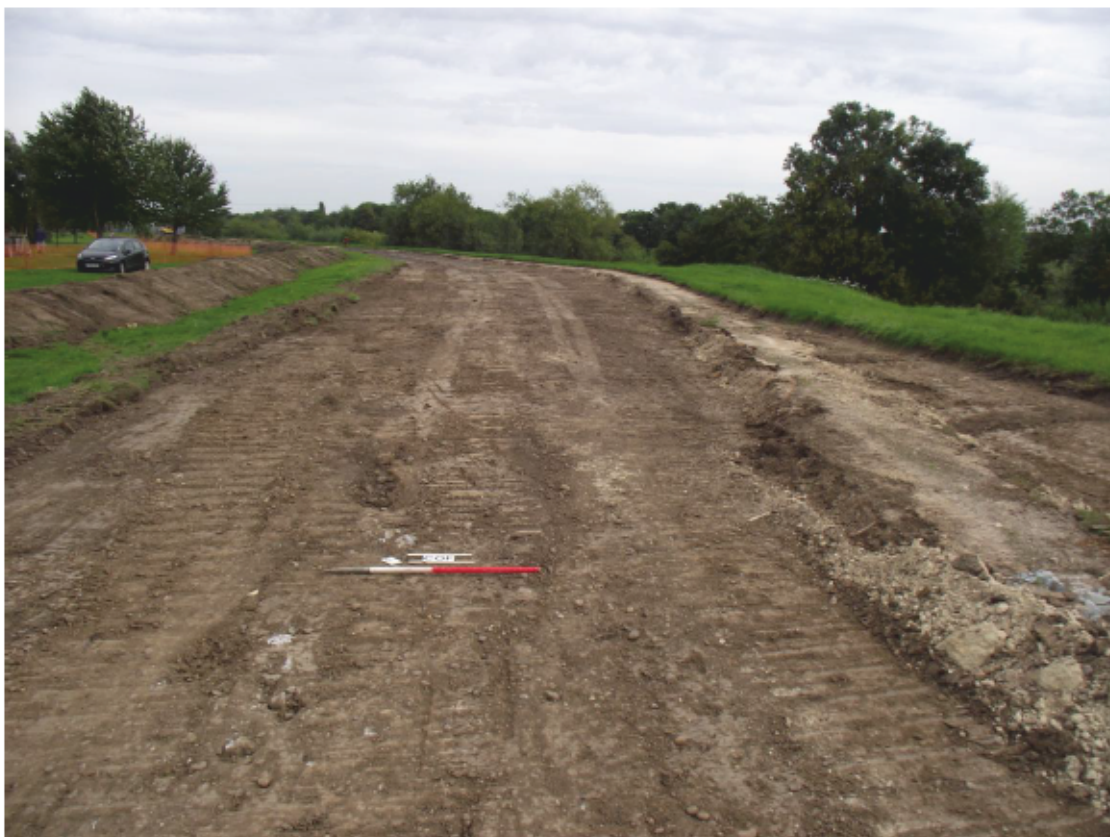
PLATE 2. Stripped flood bank, Area 02, looking north-east.
