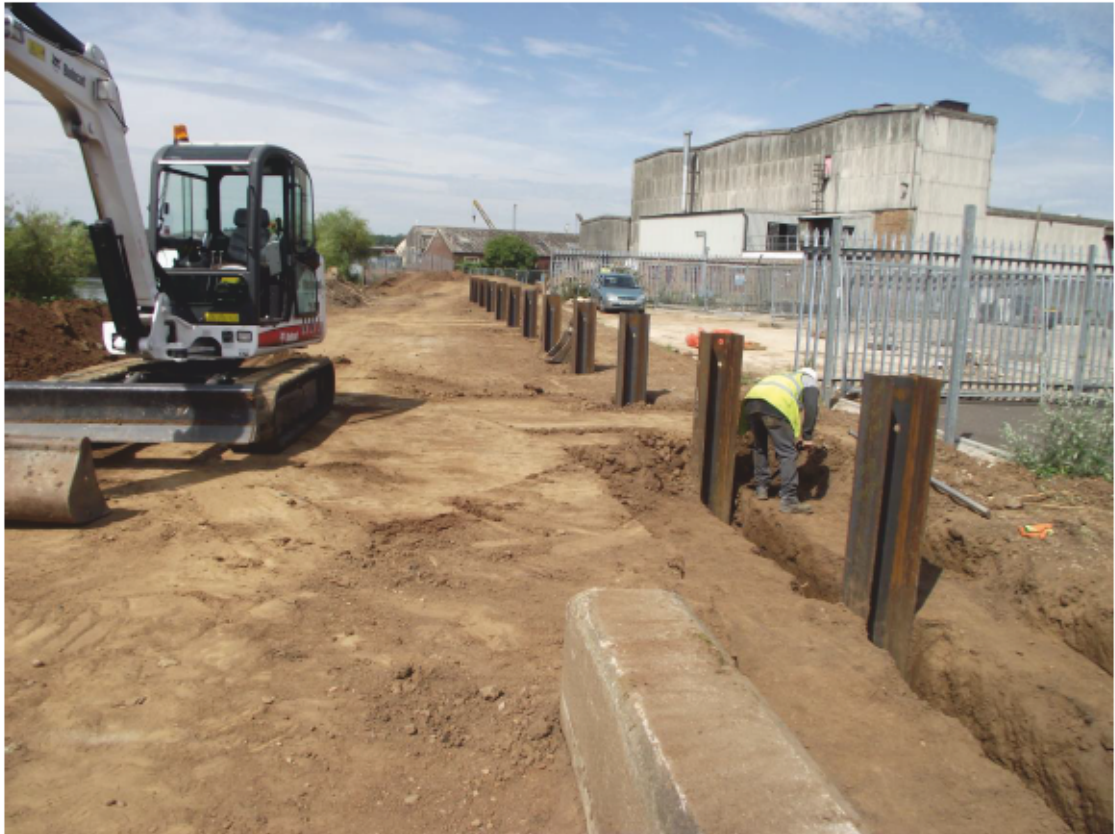
PLATE 9. Area 05, sheet piles inserted in lead trench. Looking south-east.
