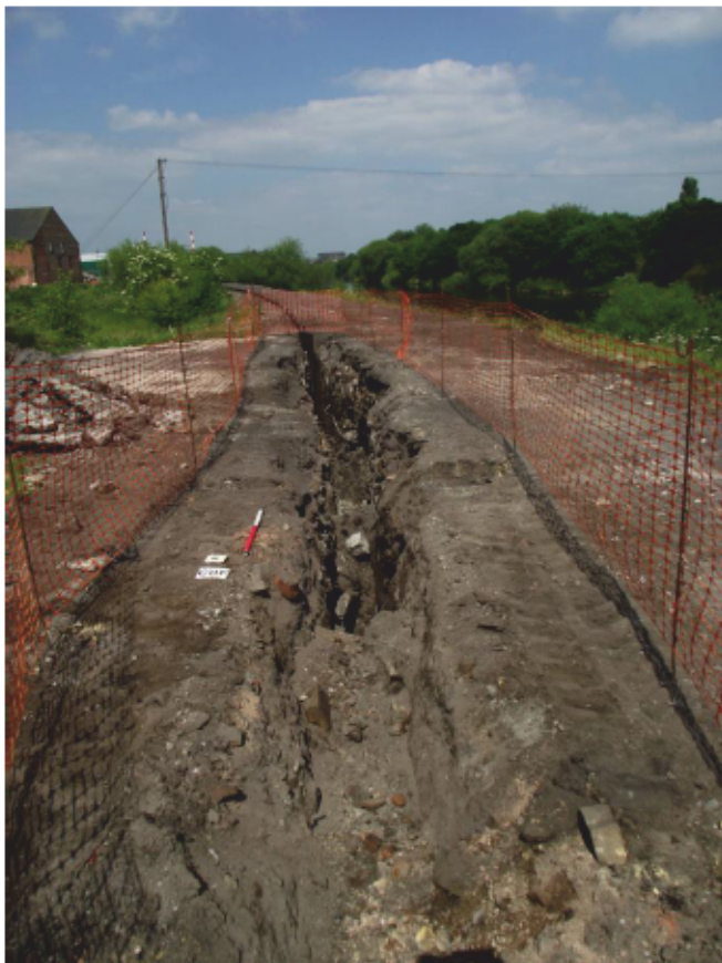
Plate 10. Deep excavation at the eastern extent of Area 02.
