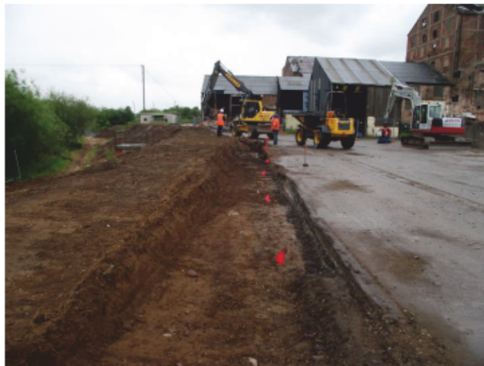
Trenching along the edge of the existing flood defence, Area 03.
