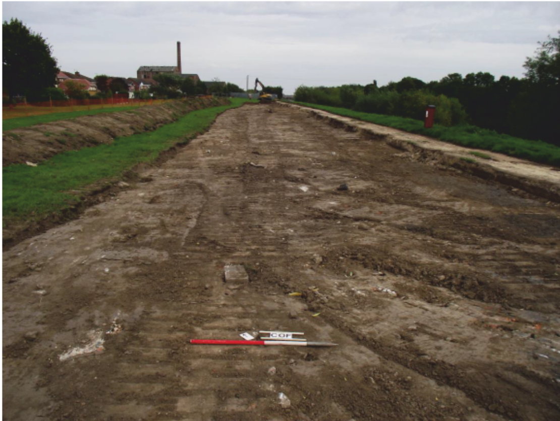
PLATE 3. Stripped flood bank, Area 02, looking south-east.
