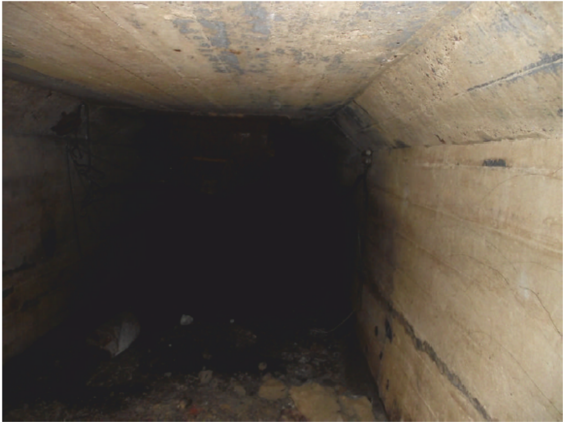
PLATE 1. Looking down the chamber from the entrance. Looking south.
