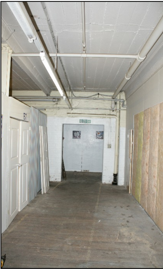
Plate 5: The interior of the showrooms in Phase C. Note the timber floor and concrete plank ceiling, viewed looking north.
