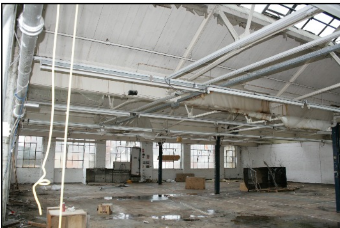
Plate 14: The first floor of Phase F, viewed looking north-east.
