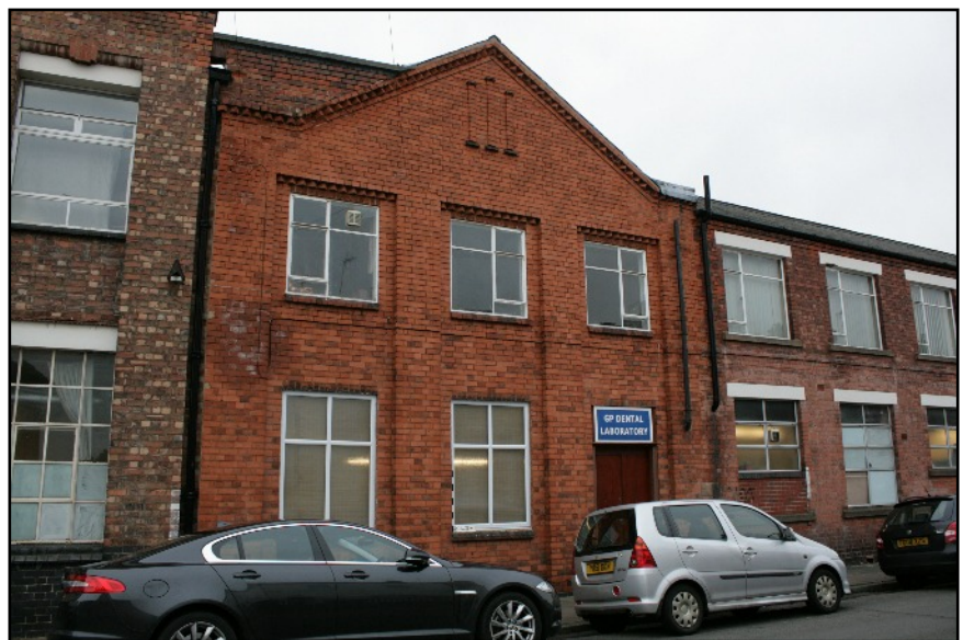
Plate 3: Post 1928 office building fronting Walton Street (Phase B), viewed looking south-east.
