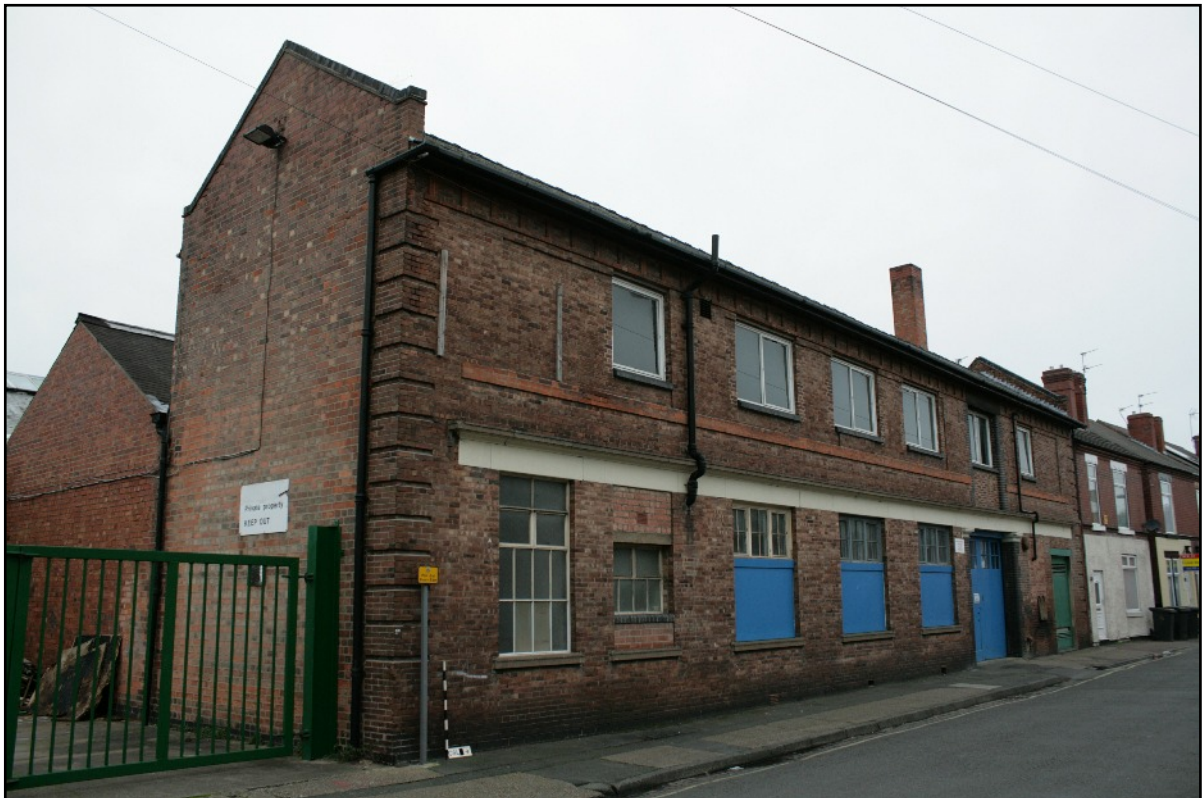
Plate 7: The building range fronting Cranmer Street (Phase D), viewed looking north-west.
