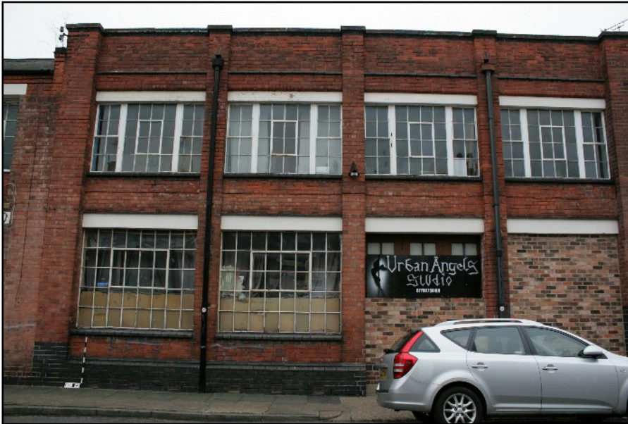
Plate 8: General view of the dispatch building fronting Walton Street (Phase E), viewed looking east.
