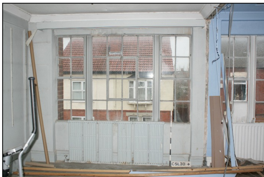
Plate 10: Original radiator and window, including tiled cill, on the north wall of the first floor of the dispatch building (Phase E), viewed looking west.
