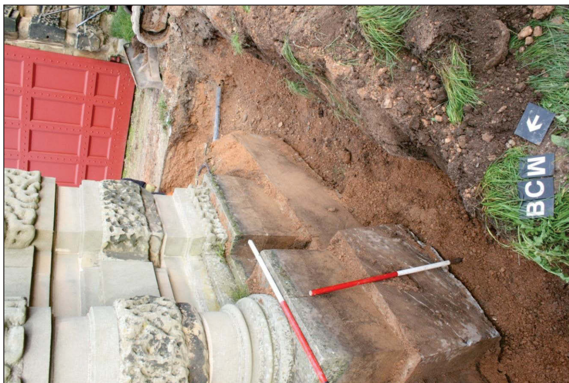
Plate 11: Section at concrete base of the northern side of the gate wall
