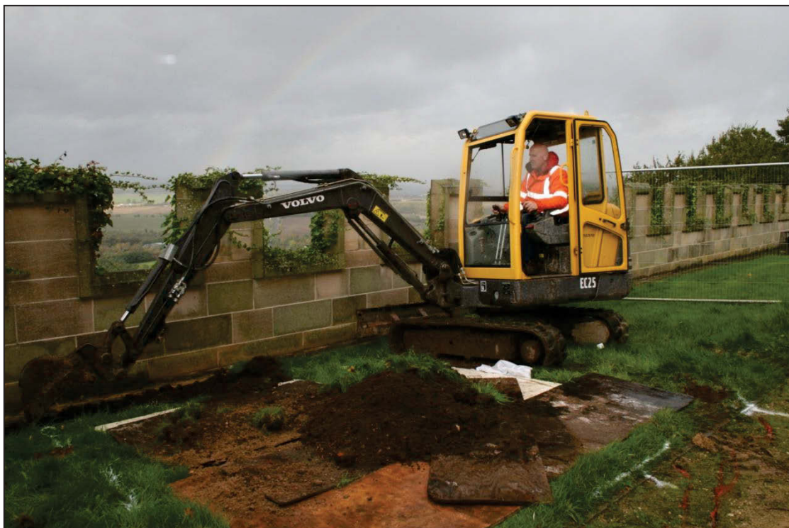
Plate 3: Excavation of area
