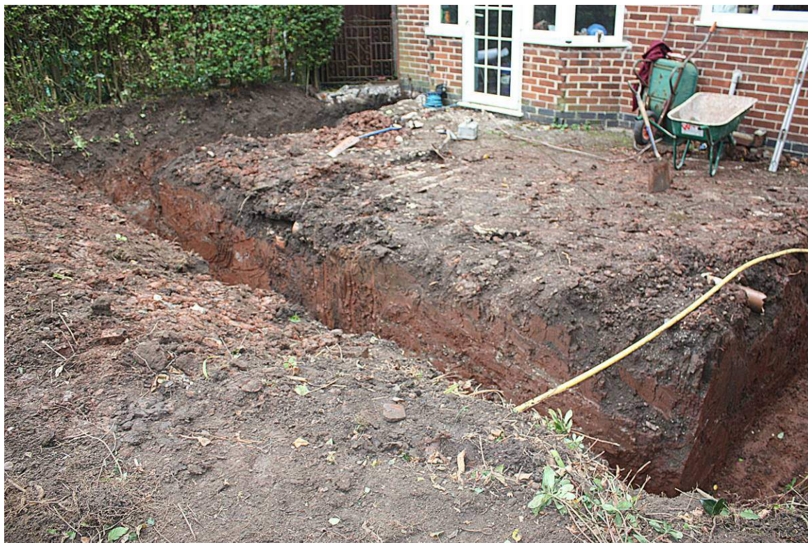
Plate 1: General view of rear extension footings trenches, looking south west.
