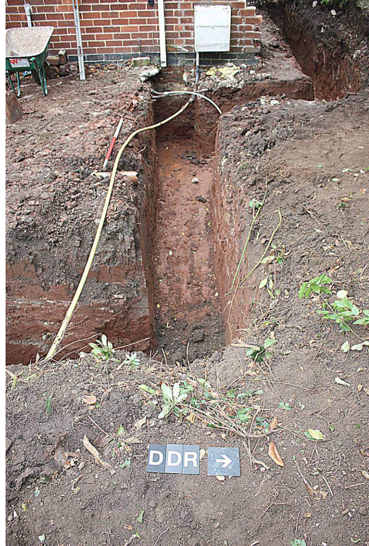
Plate 4: Footings trench for rear extension, looking west. Scale = 1m.
