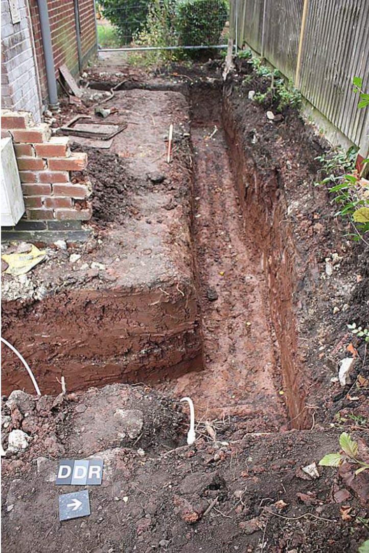
Plate 3: Footings trench for northern extension, looking west. Scale = 1m
