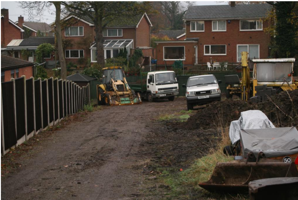
General view of the site prior to excavation, viewed looking west
