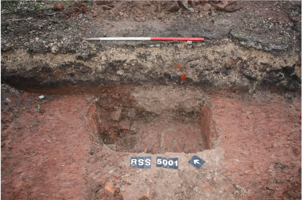
Plate 7: Foundation trench (5001) looking north east. Scale=1m
