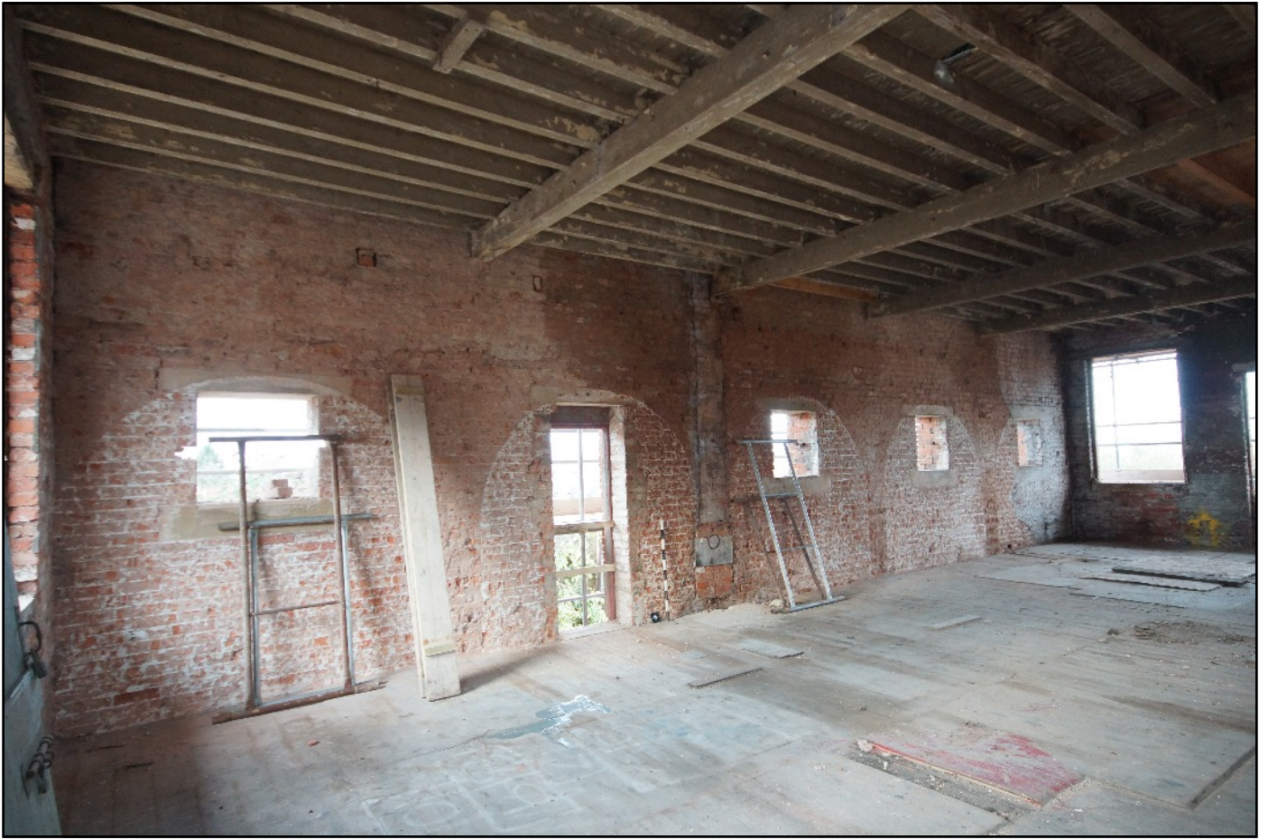
Plate 31: The north wall of the first floor of the west wing with the former cells outlined in the brickwork, viewed looking north-east.
