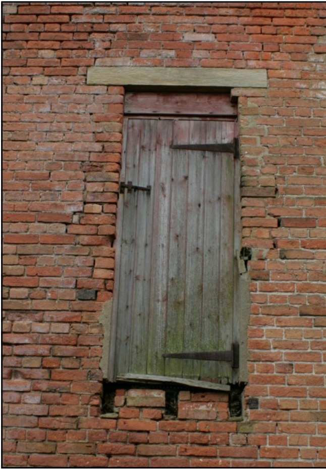
Plate 26: Inserted first floor door in the north elevation, viewed looking south.
