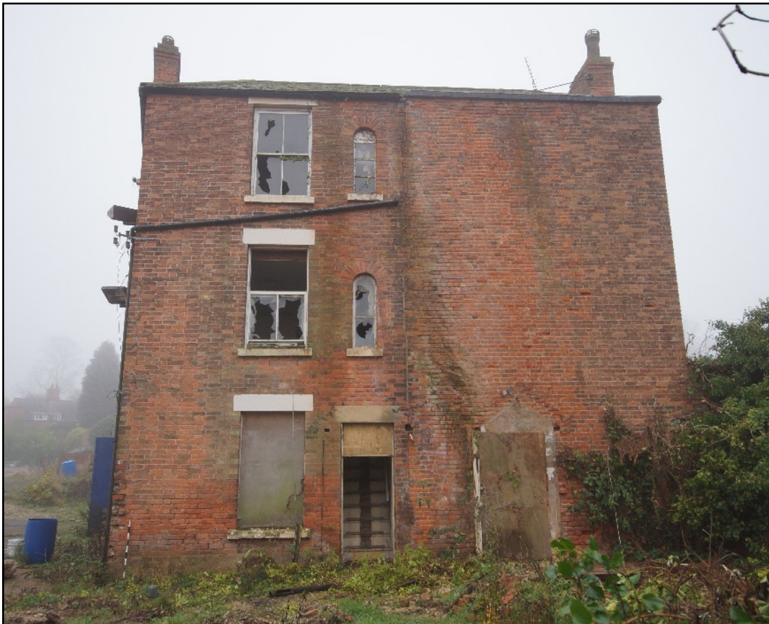
Plate 51: North elevation of the house with the building join between the east and west unit clearly visible, viewed looking south.
