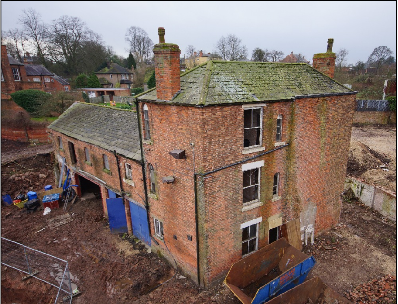
Plate 50: Aerial view of the house and the west wing looking south-west.
