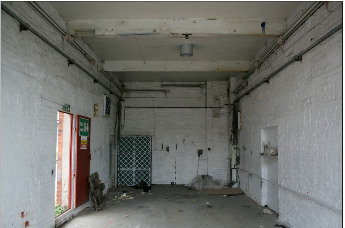
Plate 16: The interior of the engine house, viewed looking east.
