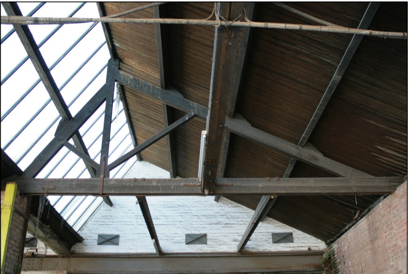
Plate 7: Truss 2, Bay 2 Unit 5, viewed looking east.
