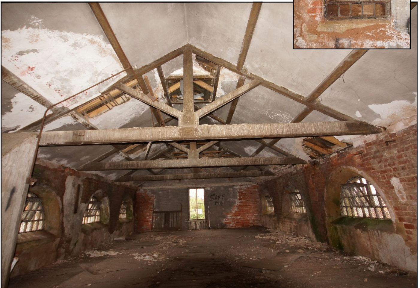
Plate 36: Second floor of the west wing viewed from Bay 5 looking west.
