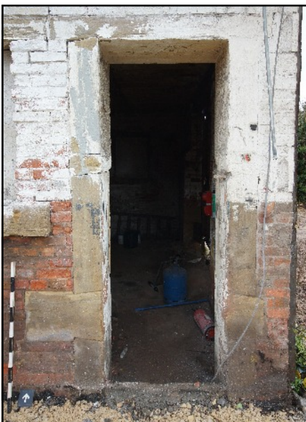
Plate 23: Ground floor doorway of the south elevation, viewed looking north.
