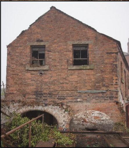
Plate 40: South gable of the west wing, viewed looking north
