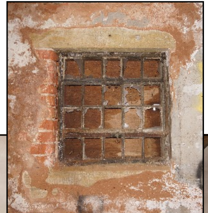
Plate 34: Infilled holes for the original ceiling beams of 1818 in the first floor north wall, viewed looking south.
