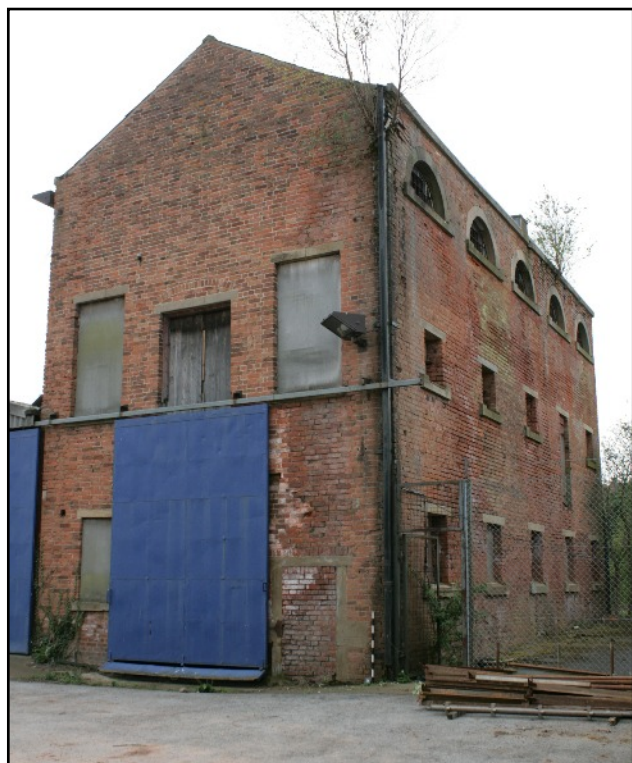
Plate 18: East gable and north elevation of the north wing of the penitentiary, viewed looking south-west.
