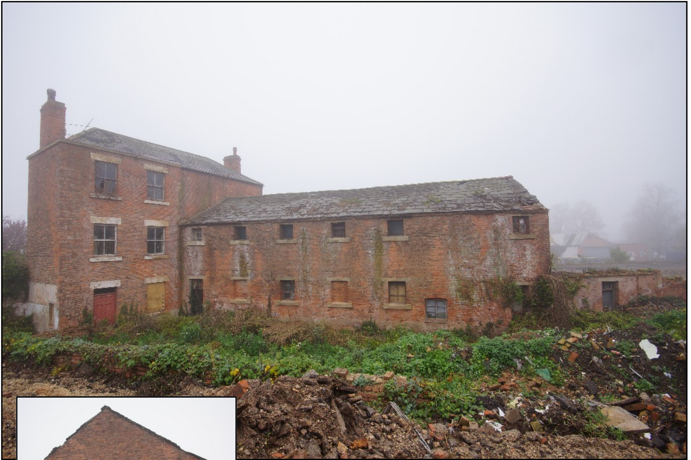
Plate 39: West wing of the penitentiary and the house, viewed looking east.
