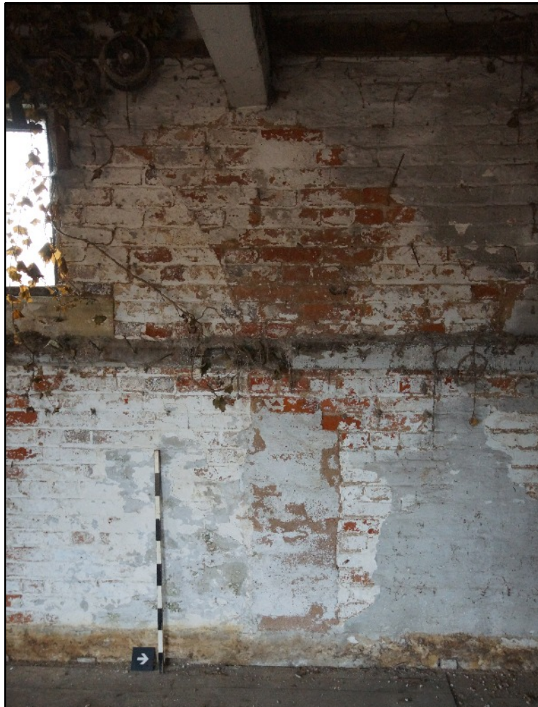
Plate 49: Outline of two prison cells on the first floor of the west wing, Bay 4 on the west wall, viewed looking west.
