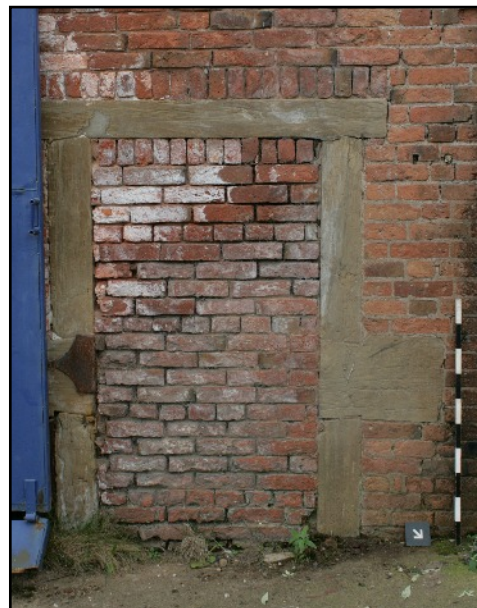
Plate 24: Ground floor doorway of the east gable, viewed looking west.
