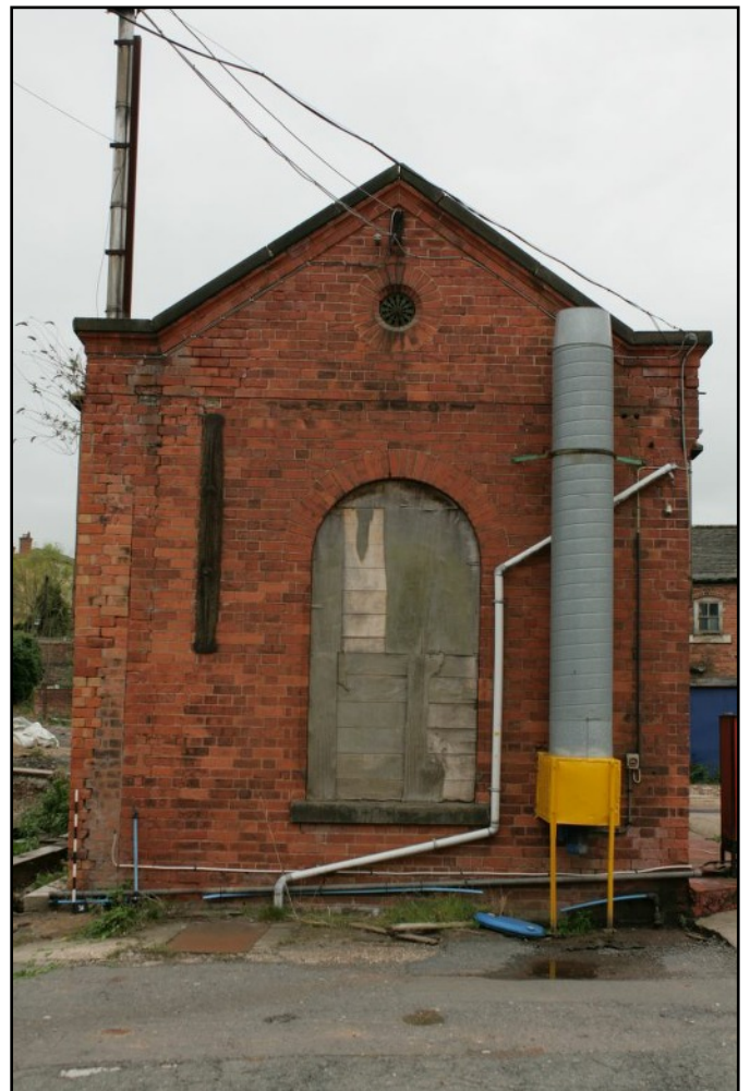
Plate 12: East gable of the engine house, viewed looking north-east.
