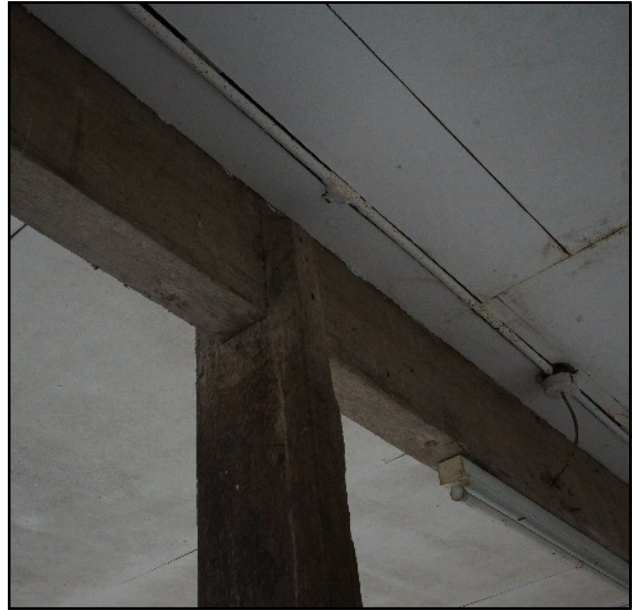
Plate 46: Sampson post in the ground floor north room of the west wing, viewed looking south-east.
