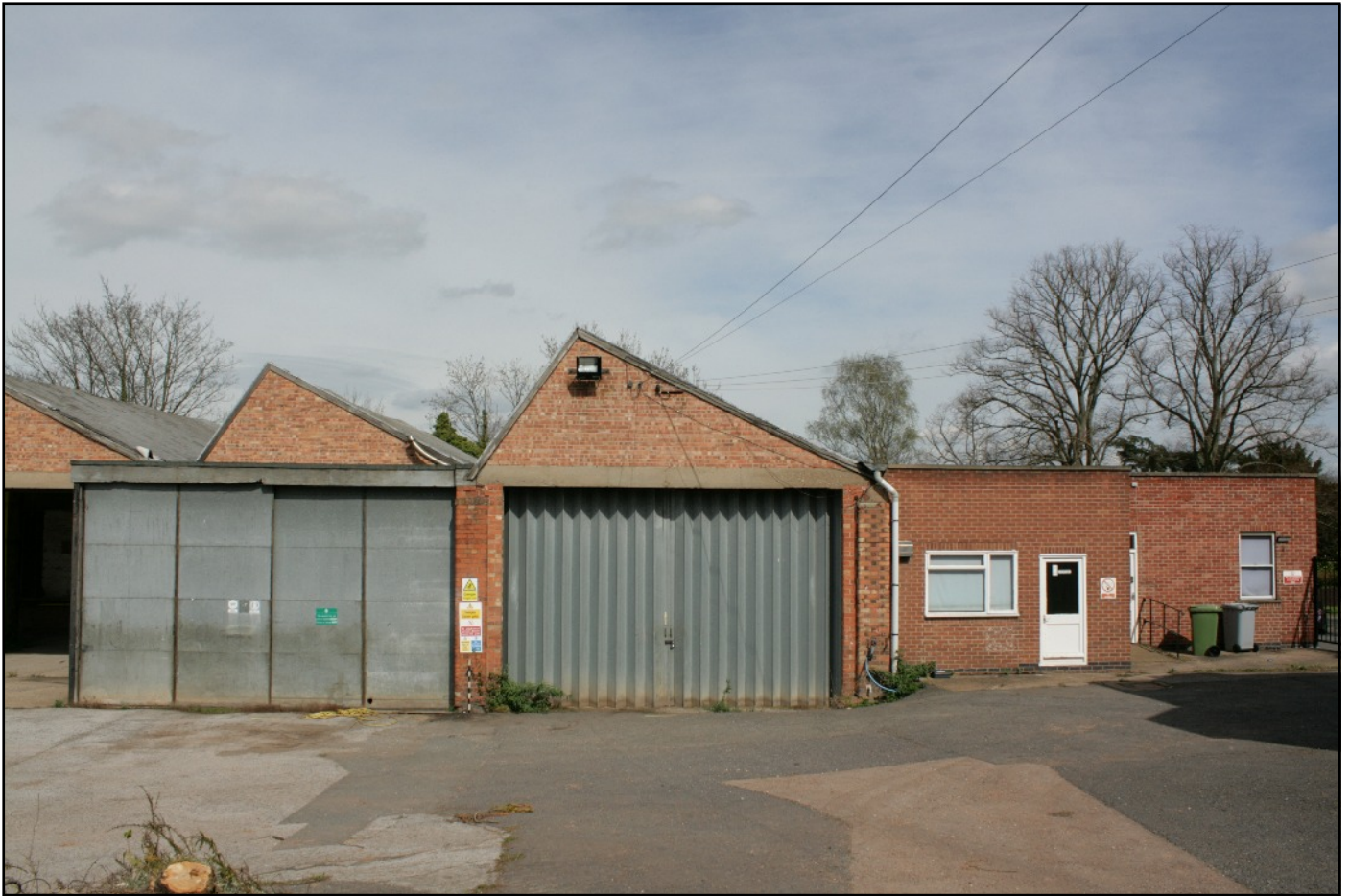
Plate 3: The south end of the former lace factory with the only surviving complete western bay dating to between 1884 and 1900 flanked by the late 20th century office to the south and garage extension to the north, viewed looking east.
