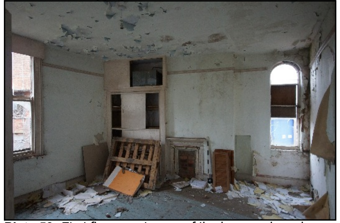
Plate 53: First floor, east room of the house, viewed looking north-east.
