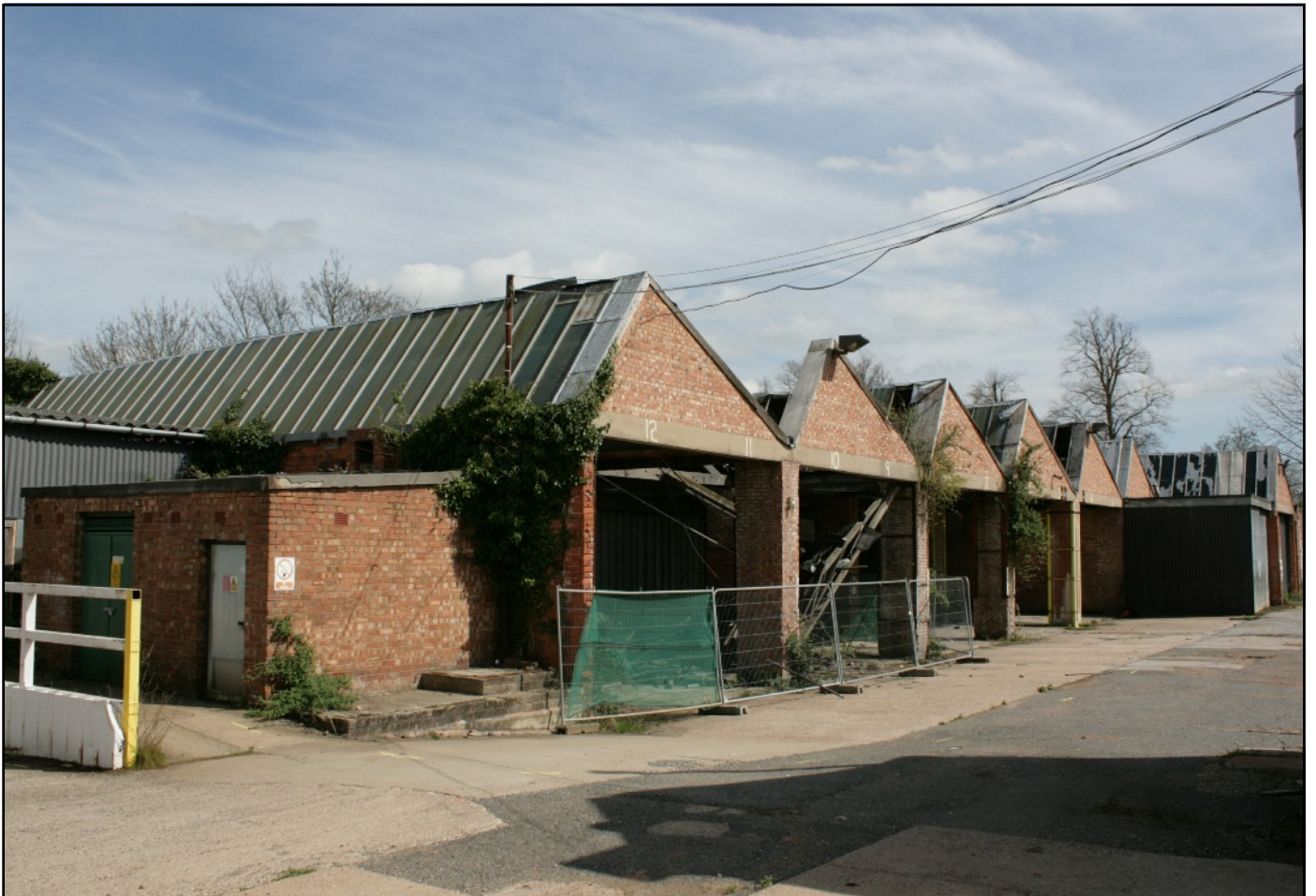
Plate 2: General view of the former lace factory, viewed looking south-east.
