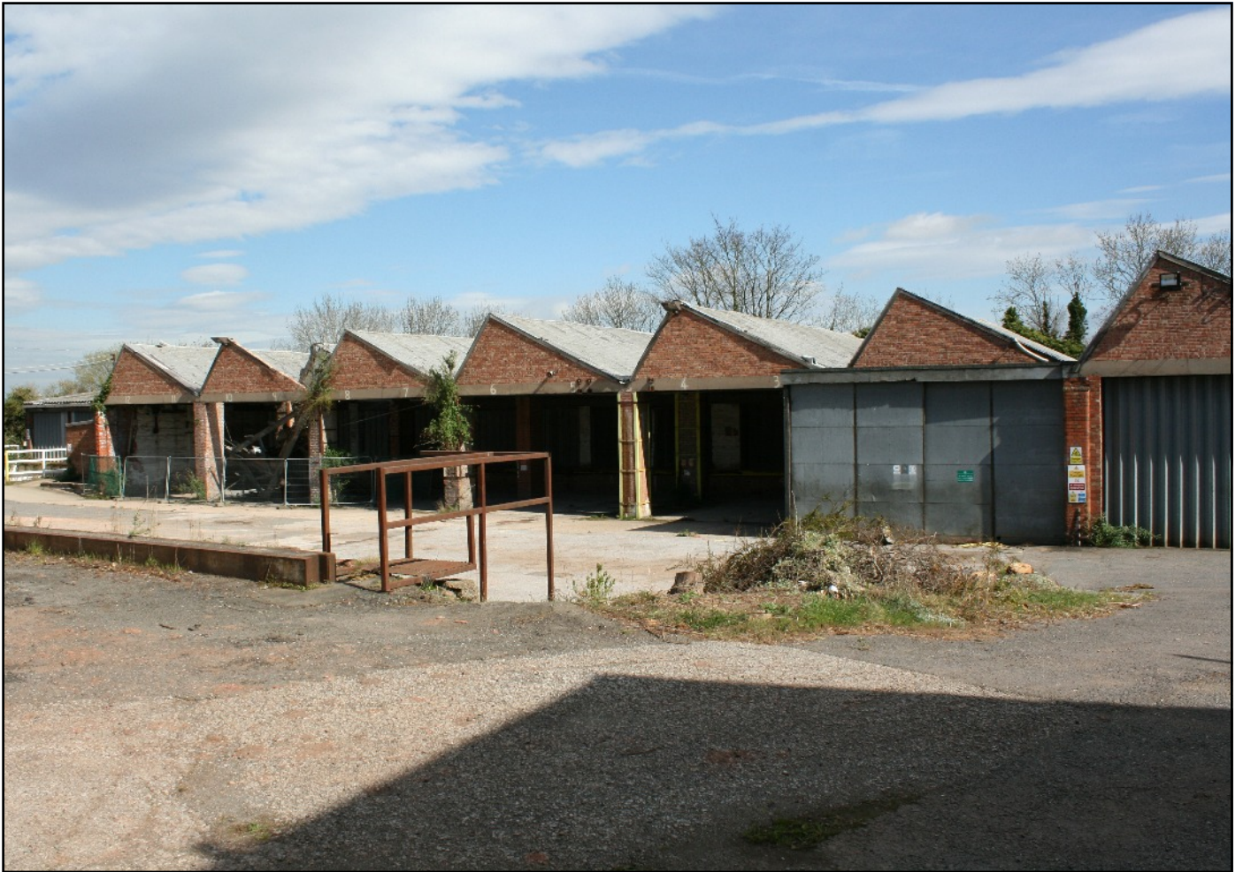
Plate 1: General view of the former lace factory, viewed looking north-east.
