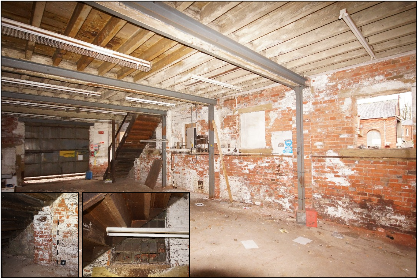
Plate 29: Ground floor of the west wing, viewed looking south-east. The inserts depict the staircase truncating the pillar supporting the ceiling beam and partially blocking the window.
