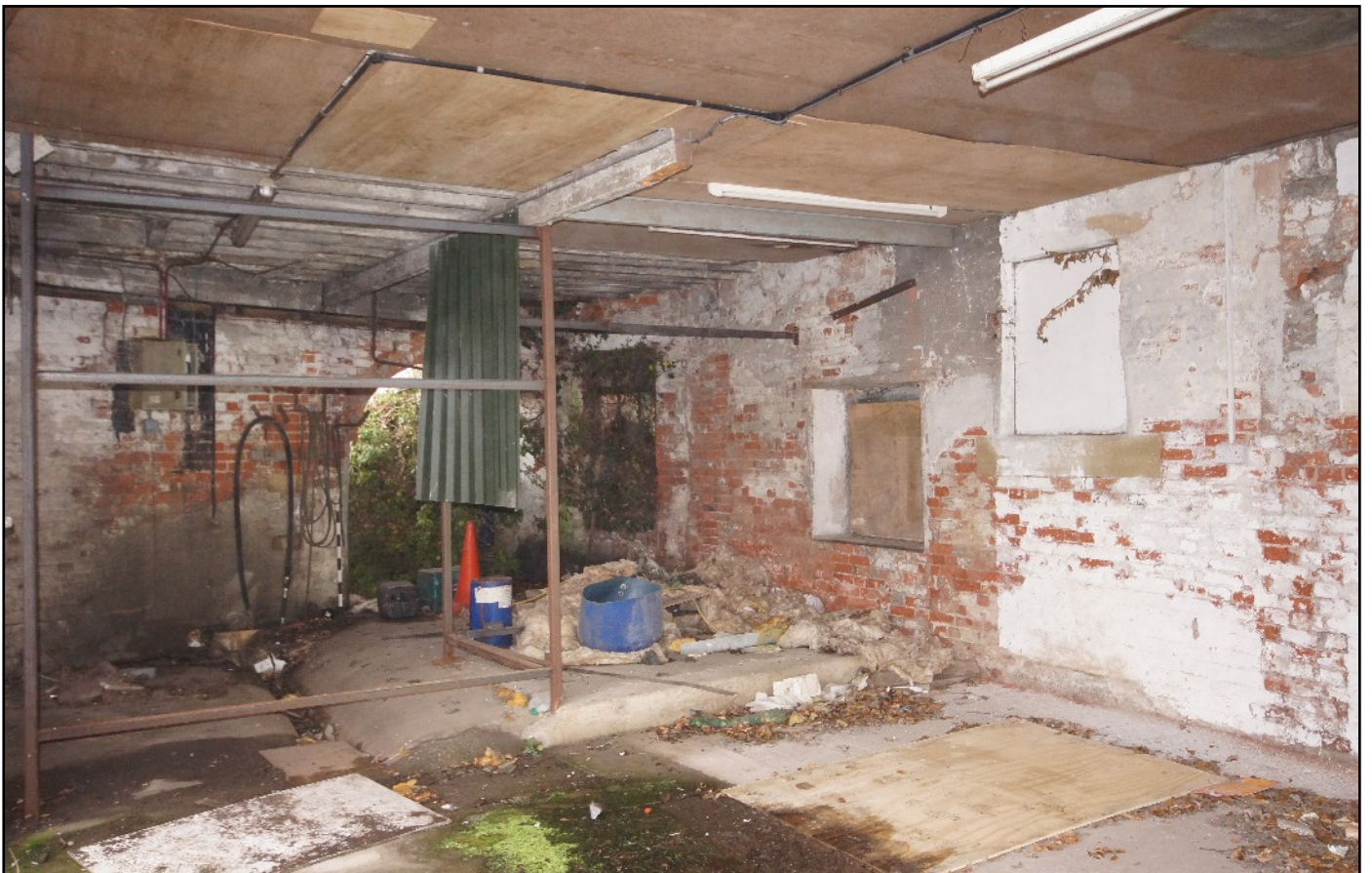
Plate 44: Ground floor, south room, of the west wing, viewed looking south-west.
