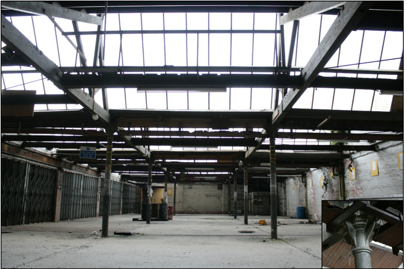
Plate 8: The interior of the former lace factory viewed looking north from Bay 4 Unit 7. The insert depicts the column capital supporting the trusses.
