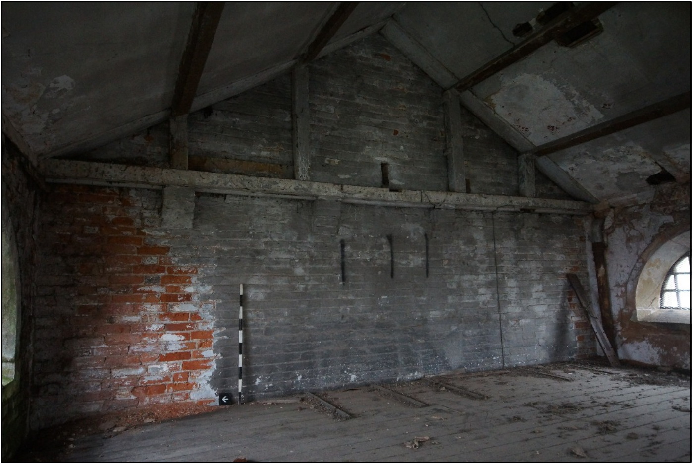
Plate 37: Truss 5 of the west wing, viewed looking south-east.
