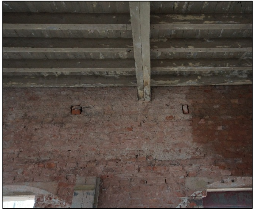
Plate 34: Infilled holes for the original ceiling beams of 1818 in the first floor north wall, viewed looking south.
