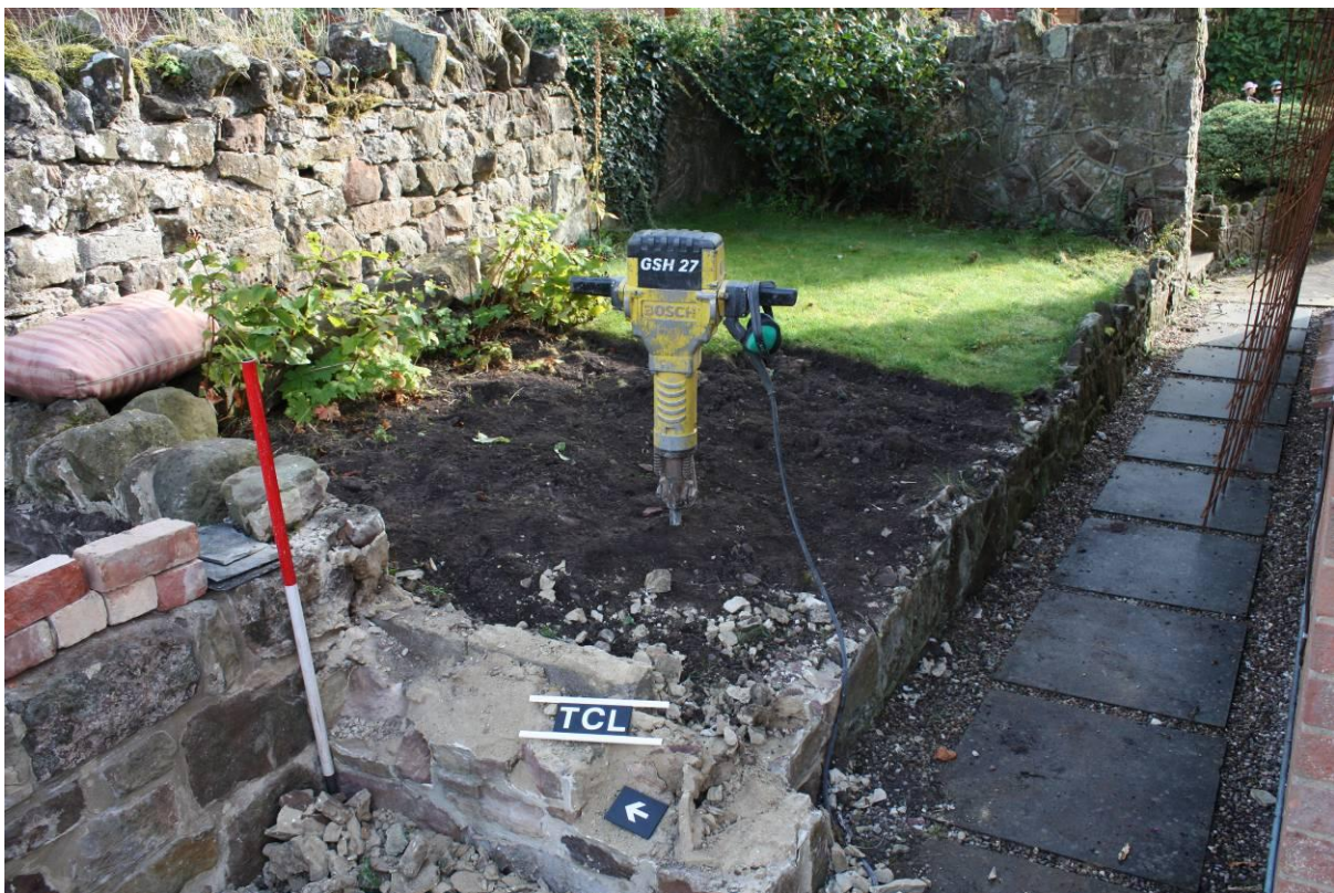
View of site prior to excavation, looking north east
