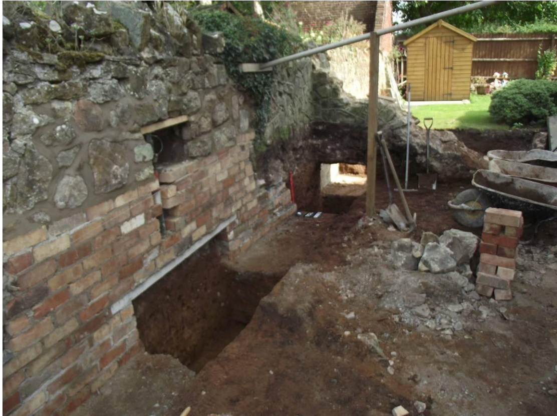
Plate 3: Garden wall with underpinning, showing the second stage of excavations.
