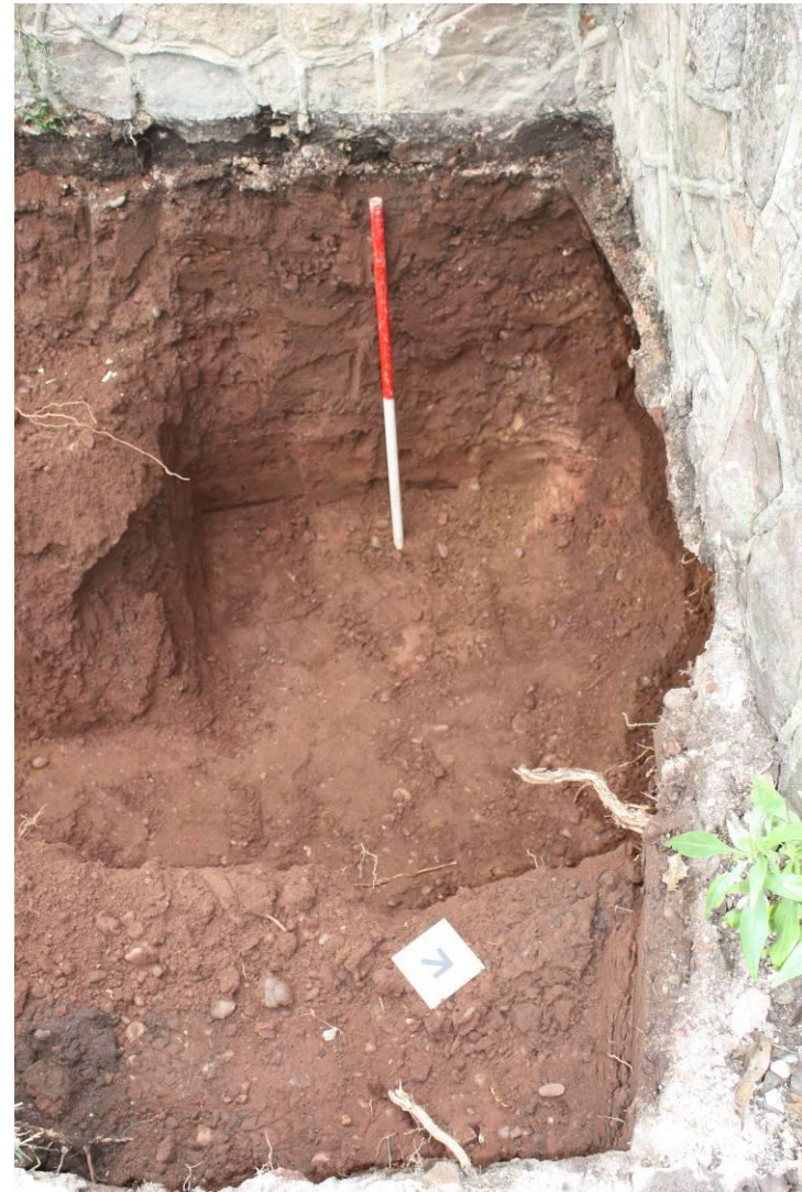
Plate 2: Eastern foundation trench looking west, showing N-S supporting wall . Scale = 1m
