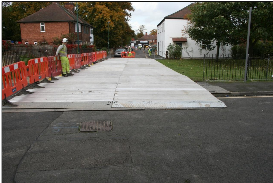
Plate 4: Site looking north on completion of fence removal and track laying.
