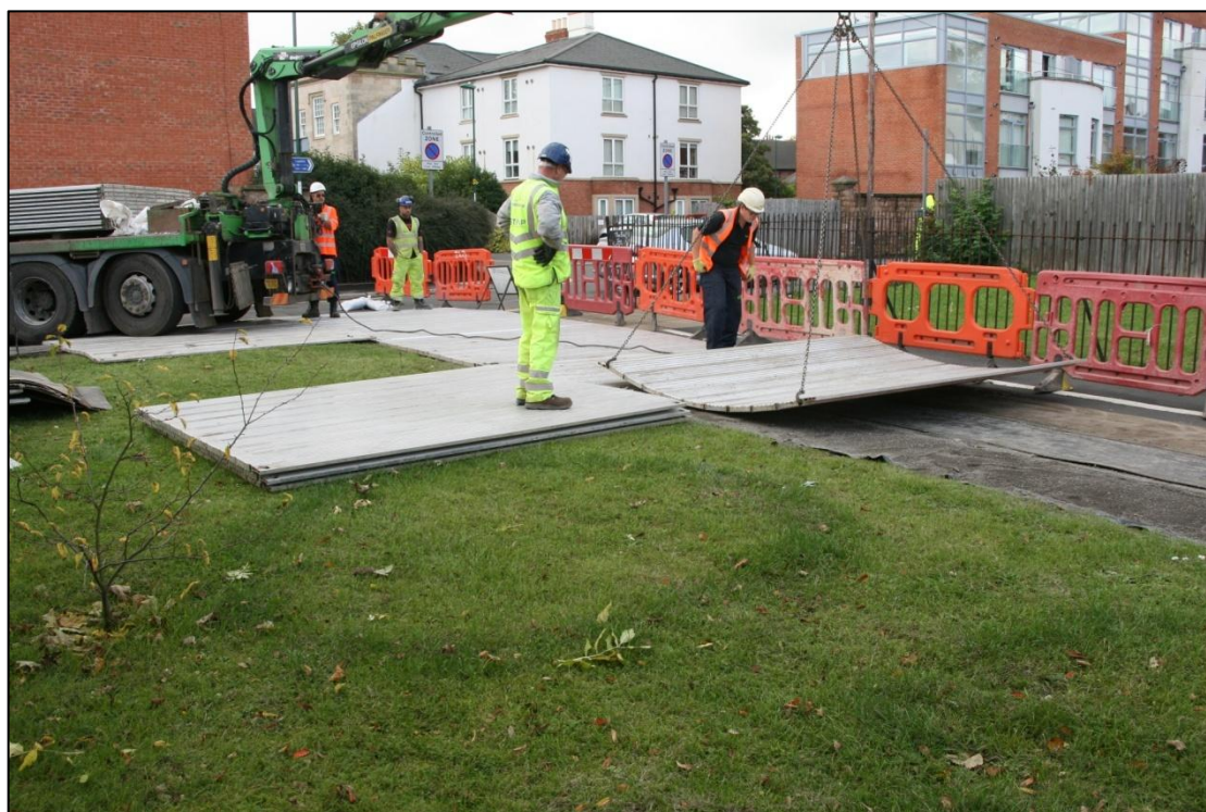
Plate 3: Placing of temporary road surface looking west
