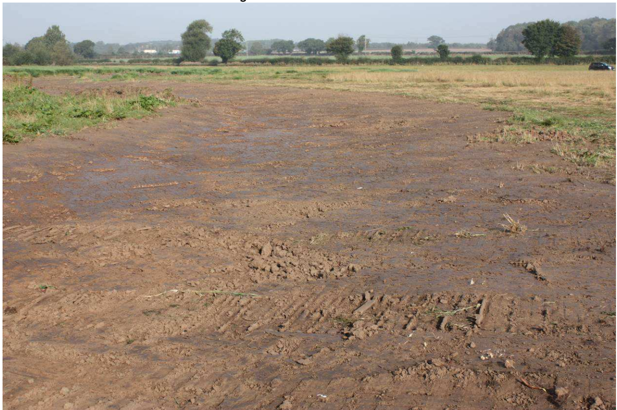
Plate 8: Area stripped for the lowering of the flood plain
