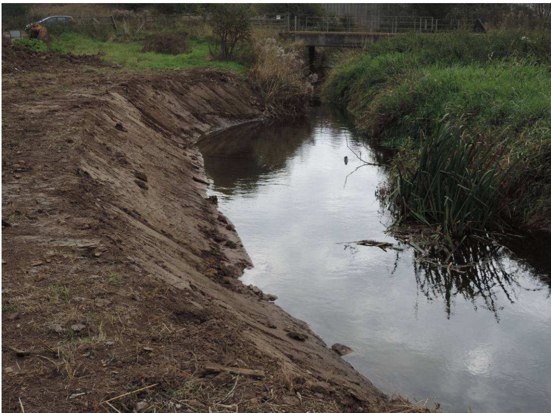
Plate 4: Regraded riverbank upstream of Weir 1
