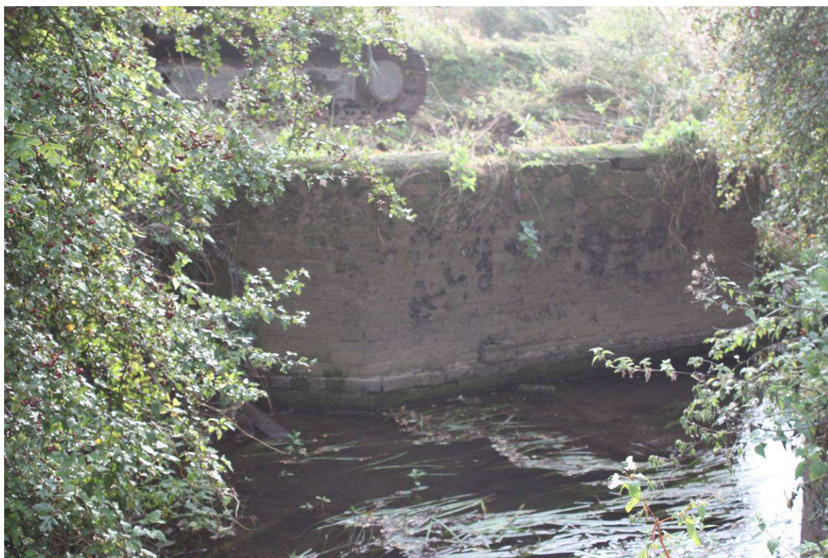
Plate 6: Weir 2 looking east
