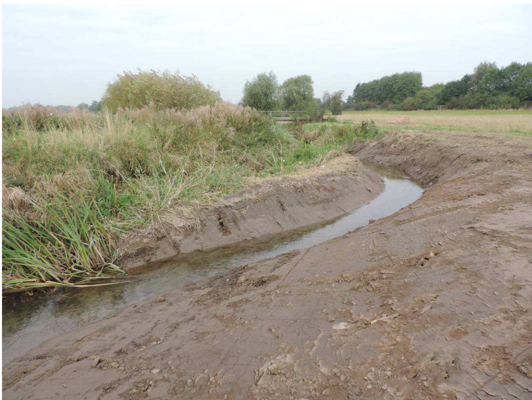
Plate 5: Regraded riverbank upstream of Weir 1
