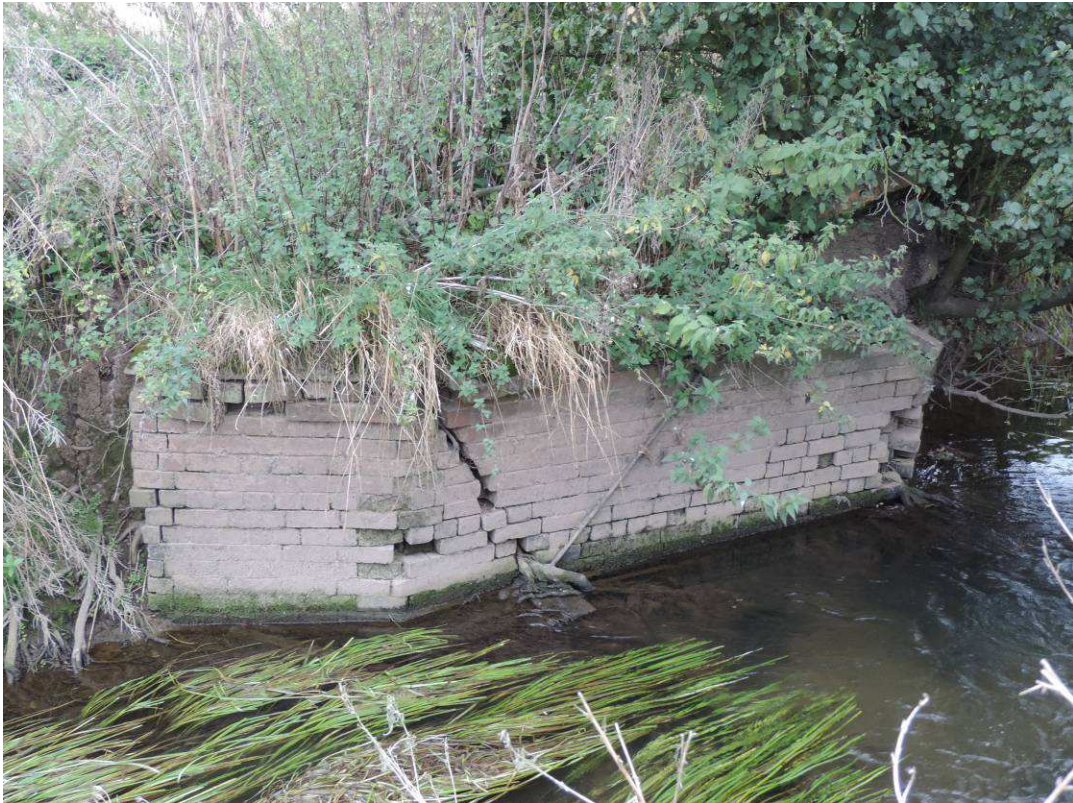
Plate 1: Weir 1 southern wall, looking south west.
