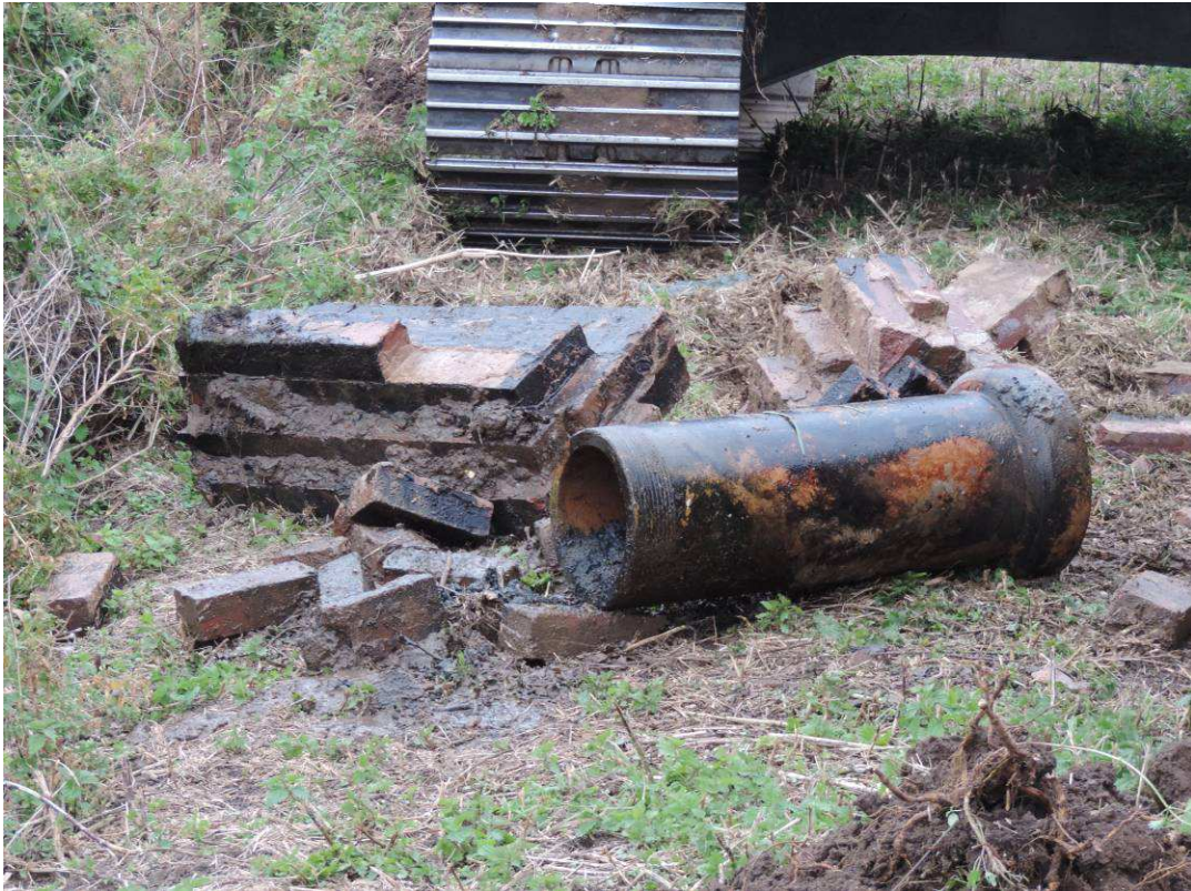
Plate 3: Remains of Weir 1 step after demolition, with ceramic pipe
