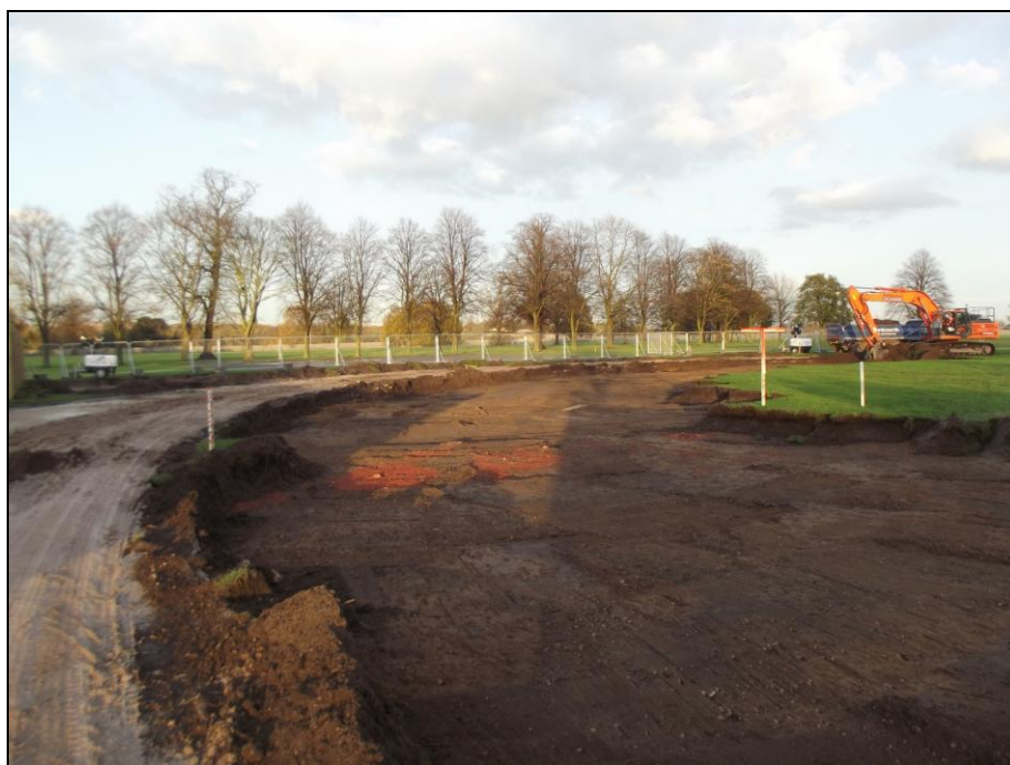
Plate 1: Area 1 looking north east
