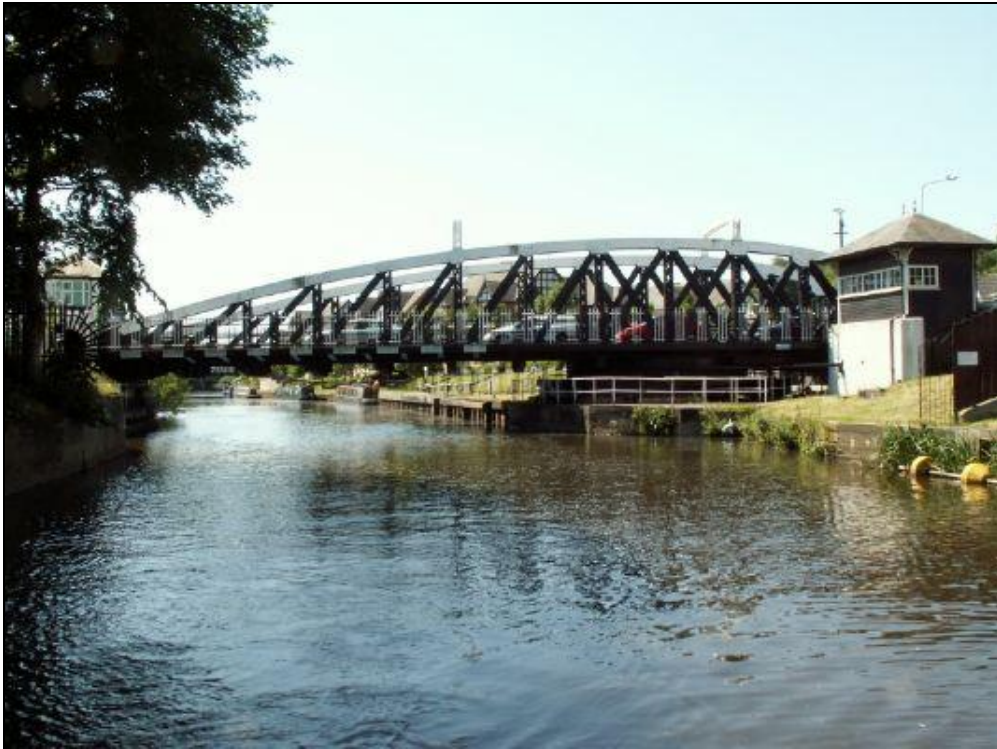
Northwich Town Bridge looking south
