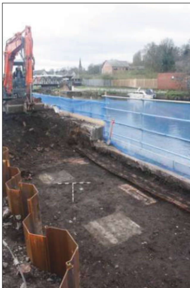
Plate 18: Footings, Reach Three at formation
