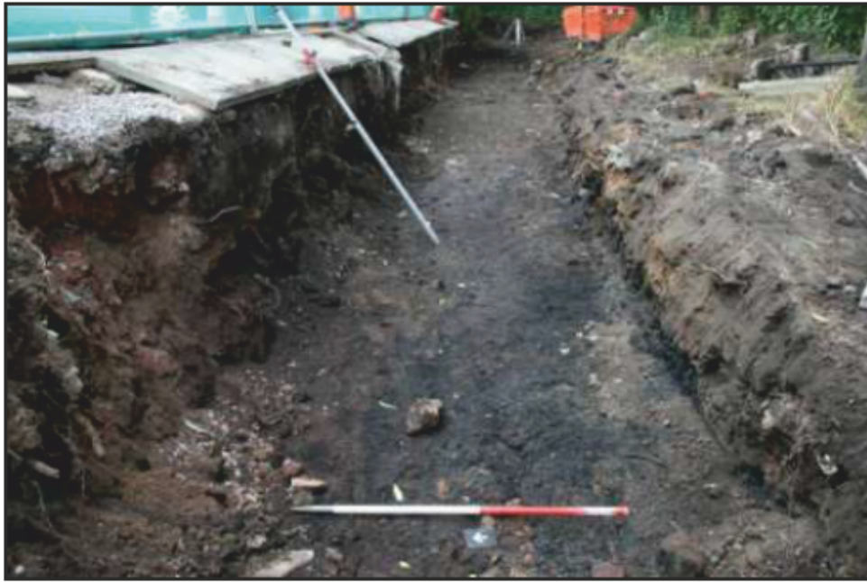
Plate 7: Excavated trench, section 2 looking east, Reach Two
