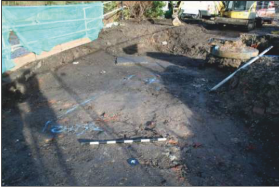
Plate 24: Extension of Reach Three for manhole
