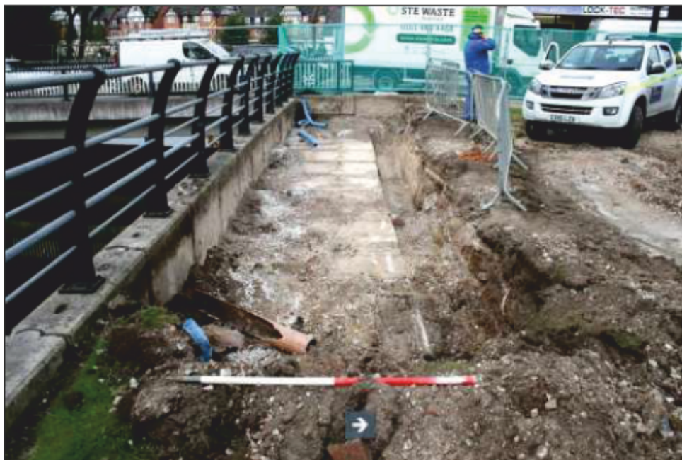
Plate 6: Concrete footings, section 2, Reach Two
