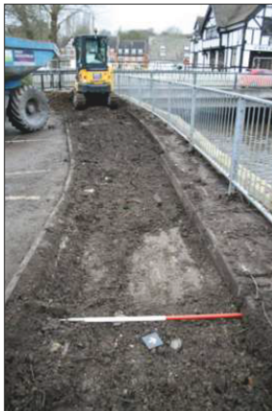
Plate 27: First phase of Reach Seven, looking north-west
