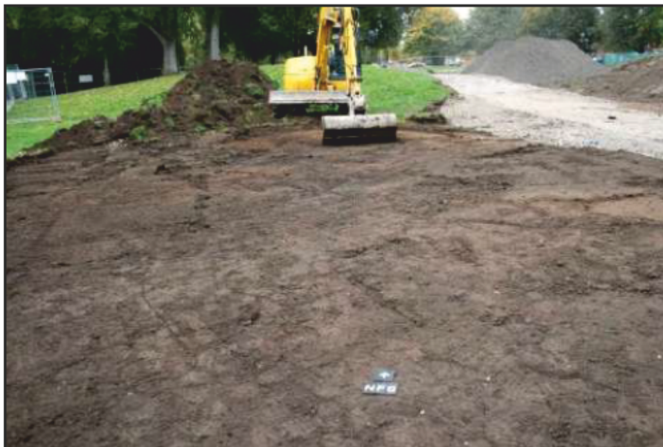
Plate 3: Topsoil strip, Reach One
