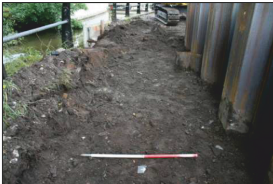
Plate 9: Excavated trench, section 2 looking west, Reach Two
