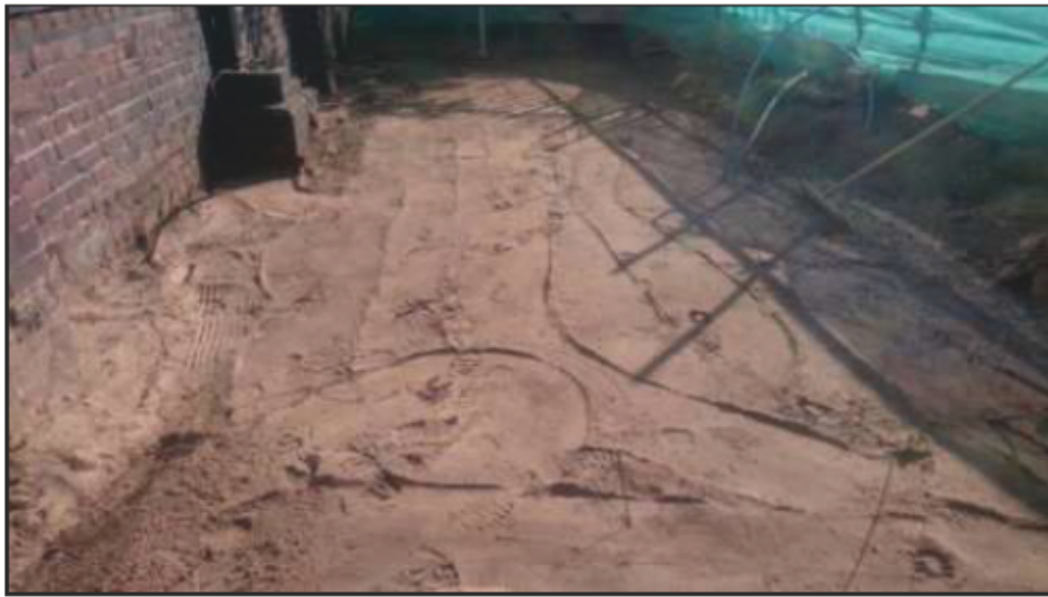
Plate 20: Slabs removed just north of Town Bridge, Reach Three
