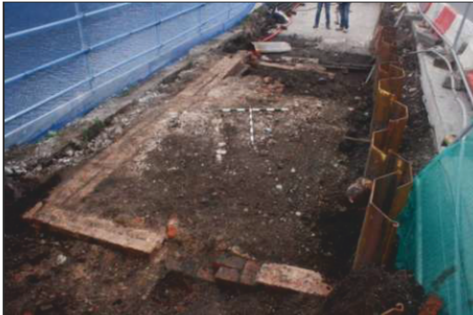
Plate 17: Brick structure (3018, 3019, 3020, 3021), Reach Three
