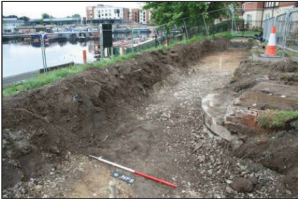
Plate 22: Reach Twelve, at formation looking south-east
