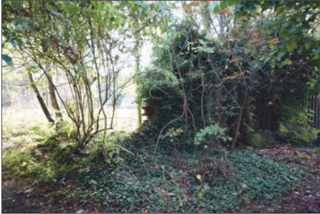
Plate 54: Wall face 20 showing ivy growth, looking south west.
