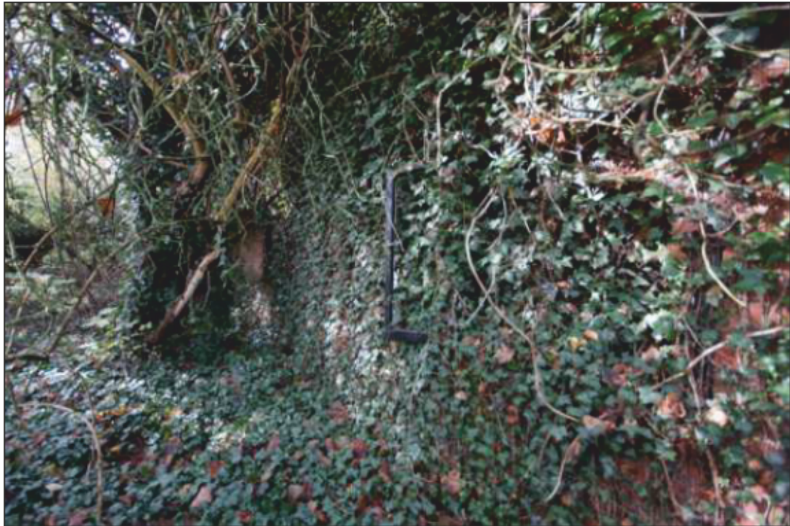
Plate 35: Wall face 11 showing window opening. looking north-west.
