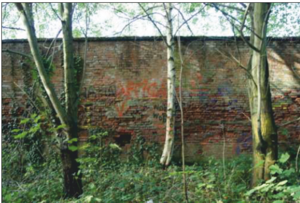
Plate 12: Wall face 6 showing condition of brickwork, looking north.
