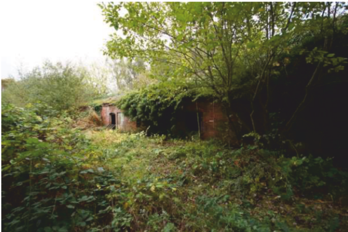
Plate 45: Wall face 18, Shed Phase 1. Looking south-east.
