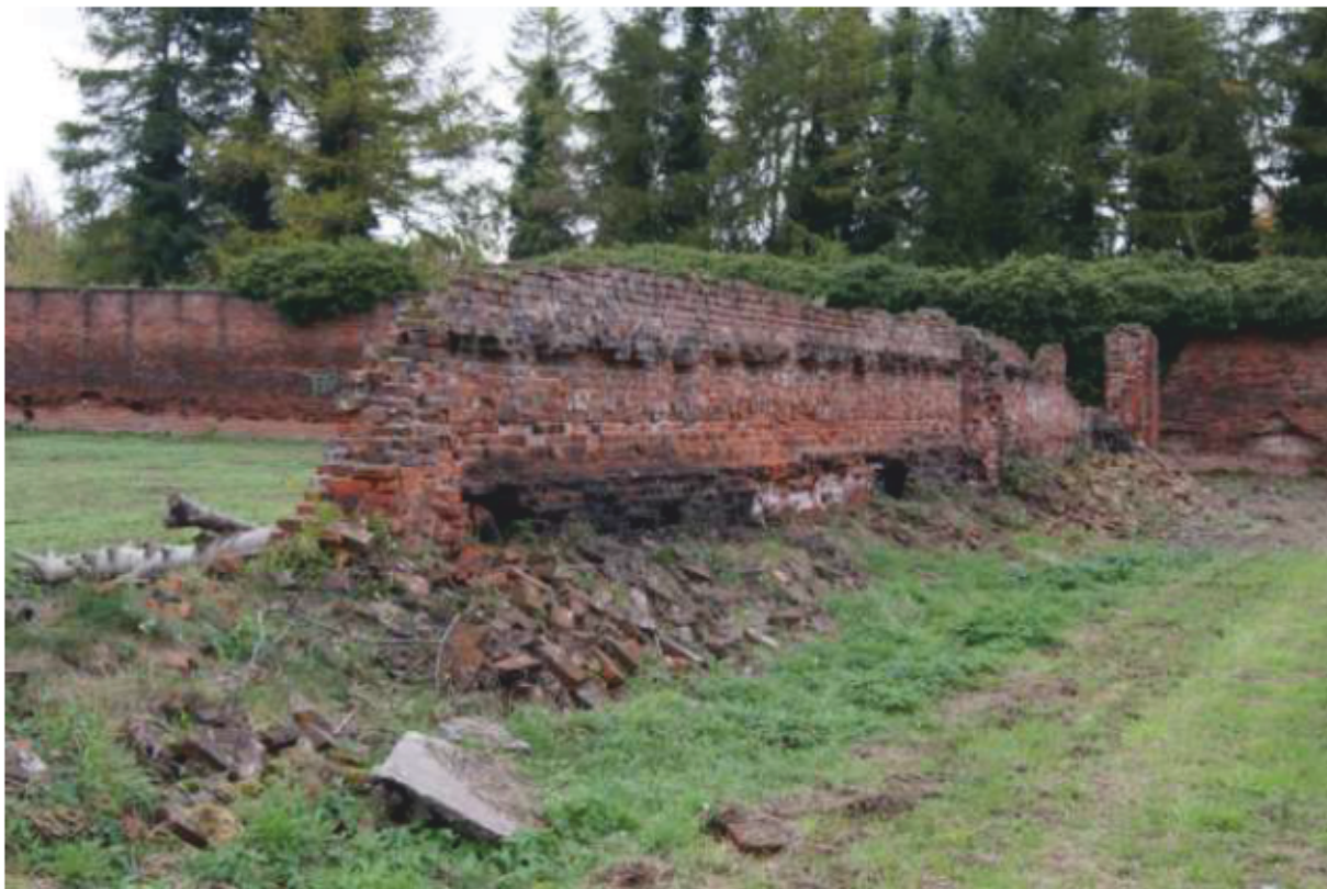
Plate 26: Wall face 15, showing exposed core of double-skinned wall. Looking north-east.
