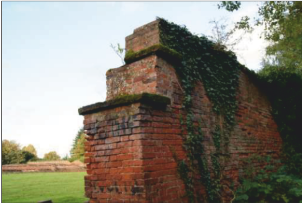
Plate 11: Wall face 6 showing condition of pillar, looking north-east.
