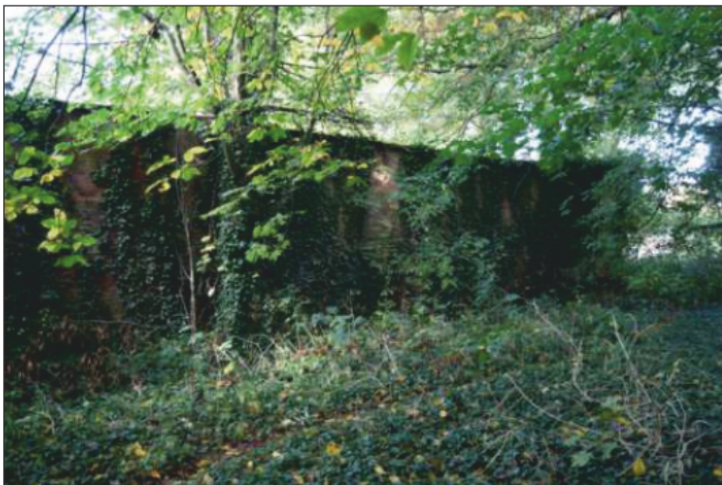
Plate 14: Wall face 6 showing ivy, looking north-east.
