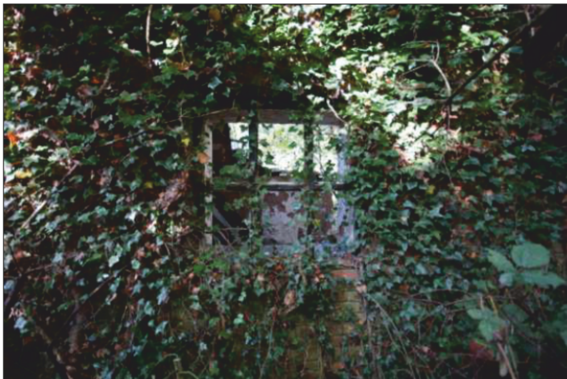
Plate 34: Wall face 11 showing window opening, looking north.
