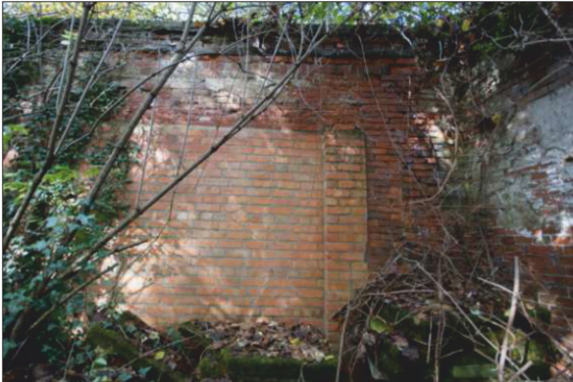
Plate 33: Wall face 11 showing infilled brickwork, looking north.
