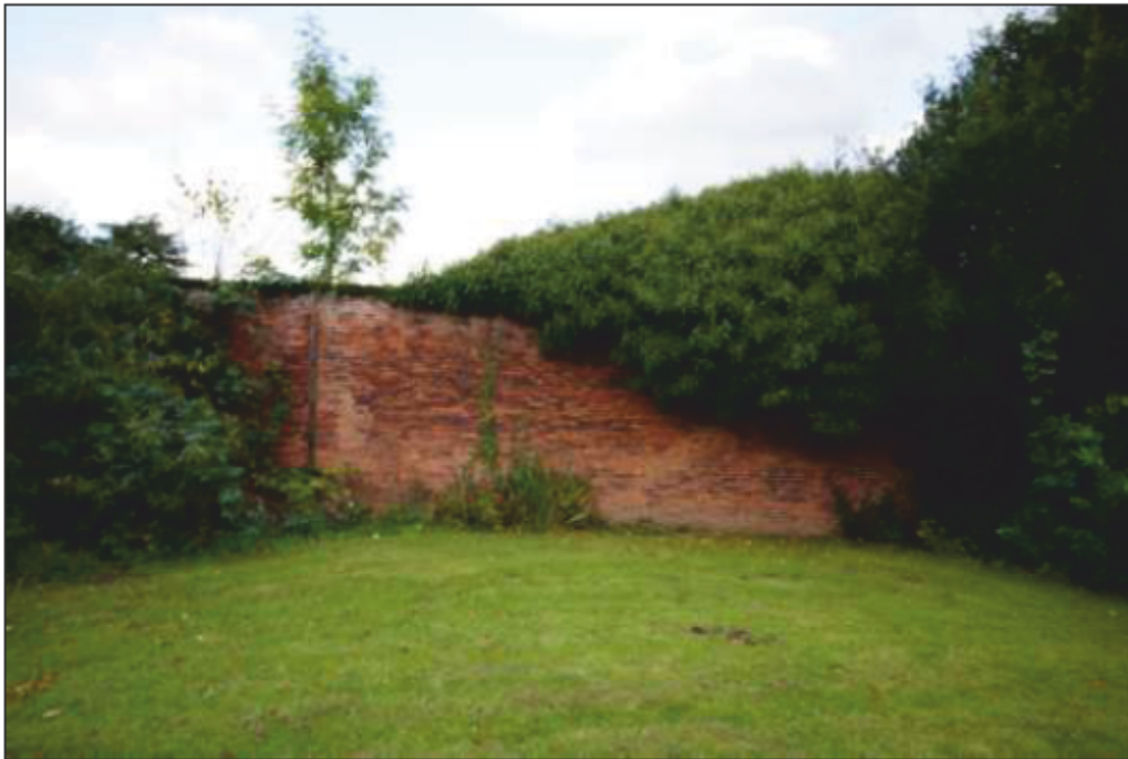
Plate 25: Wall face 14, looking east.
