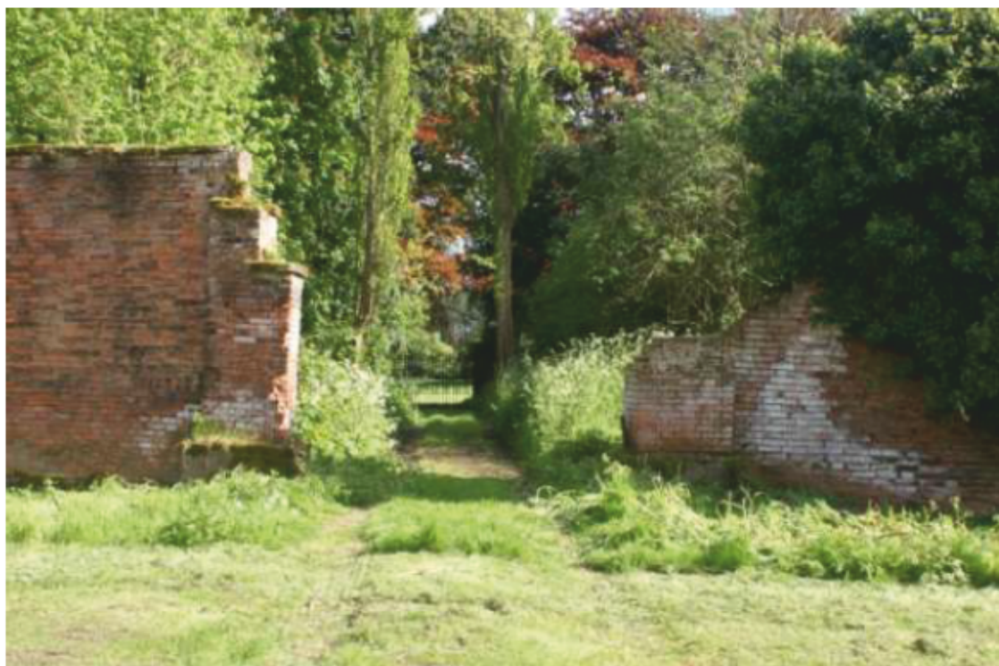
Plate 6: Wall faces 3 and 5, showing the formal southern entrance into the Park. Looking south.
