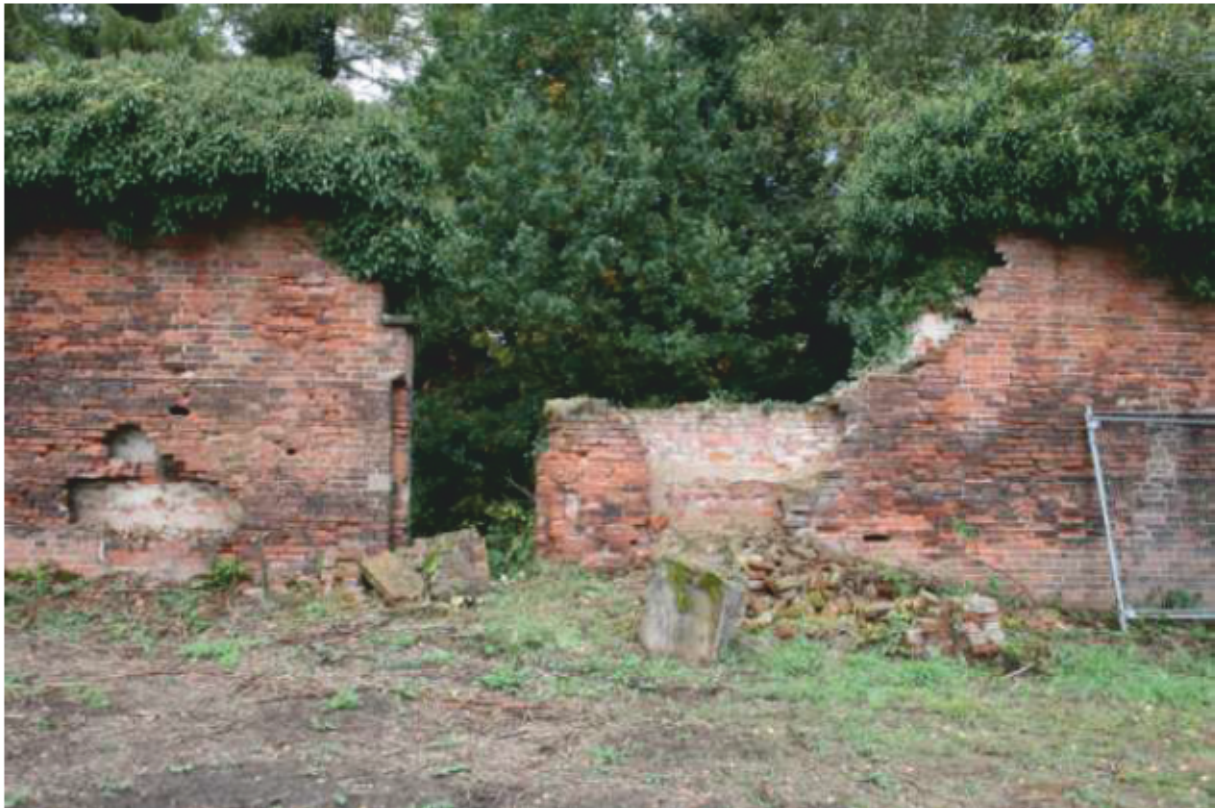
Plate 15: Wall face 7, northern end, showing the collapsed walling and gate pillar. Looking east.
