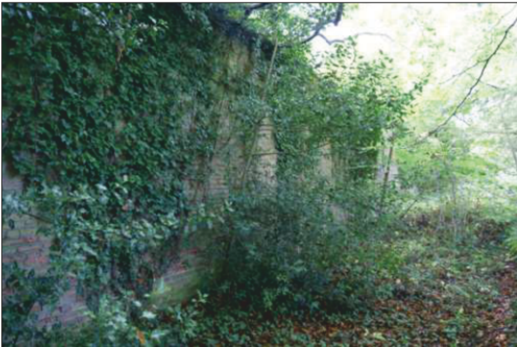
Plate 18: Wall face 8 showing ivy, looking north-west
