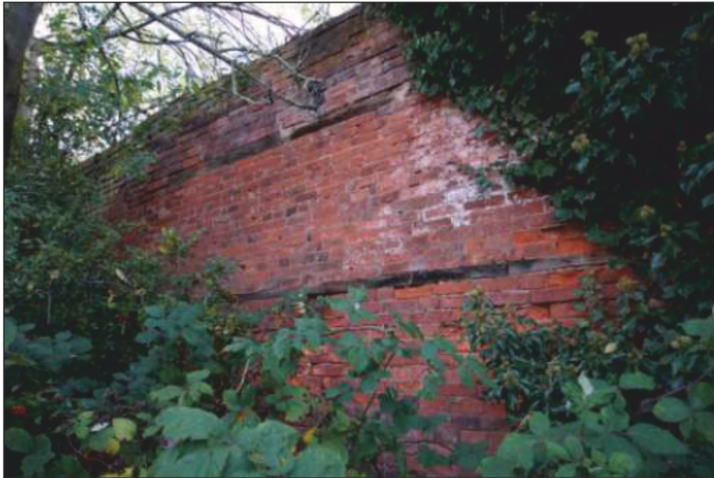
Plate 44: Wall face 17 showing wooden beams, looking north-west.
