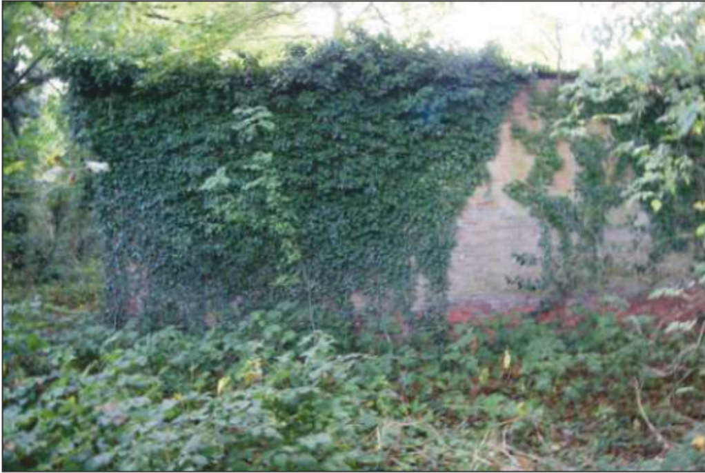
Plate 17: Wall face 8, looking west.
