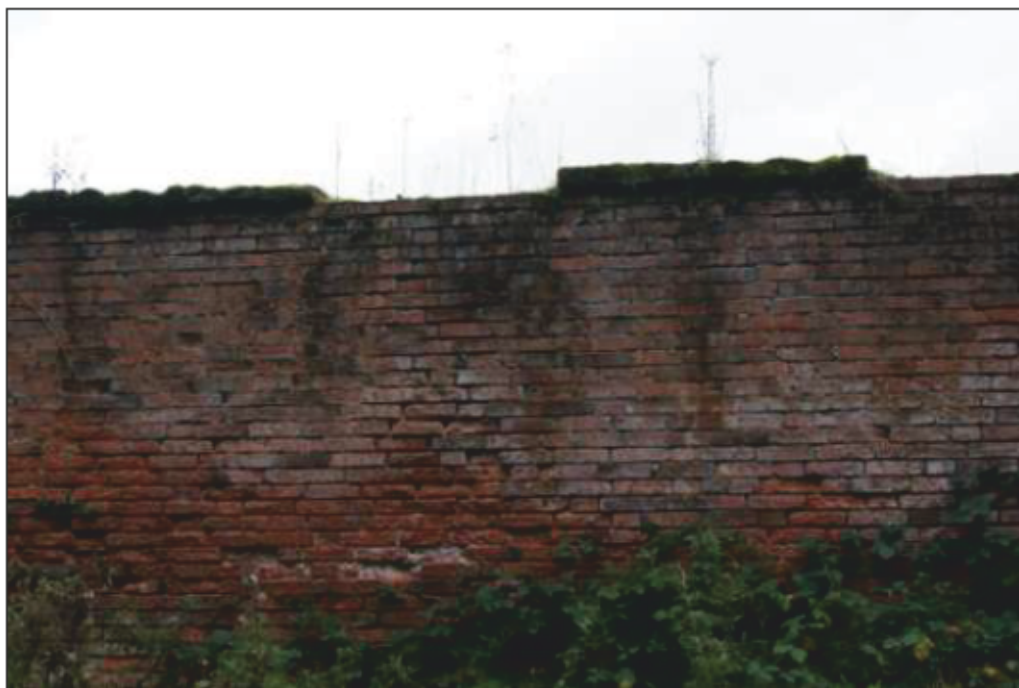
Plate 1: Wall face 1, showing remains of demolished exterior glasshouse or possible infilled entrance. Looking west.
