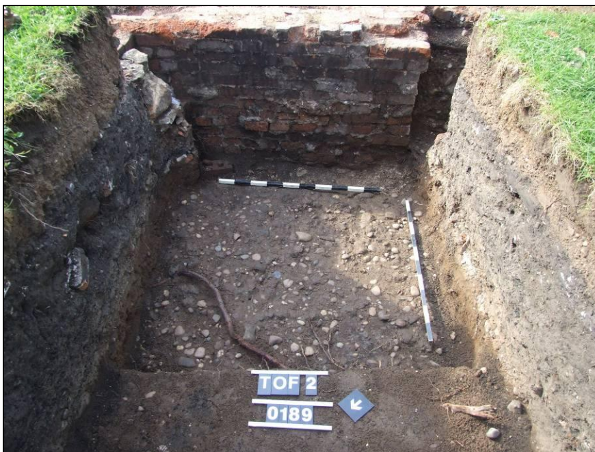
Plate 9: Compacted pebble surface (0189) looking SSE
