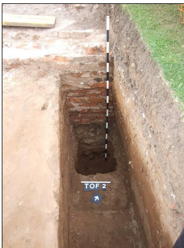
Plate 32: Sondage south of foundation (0108) showing (0223), (0224) and (0225) looking north west
