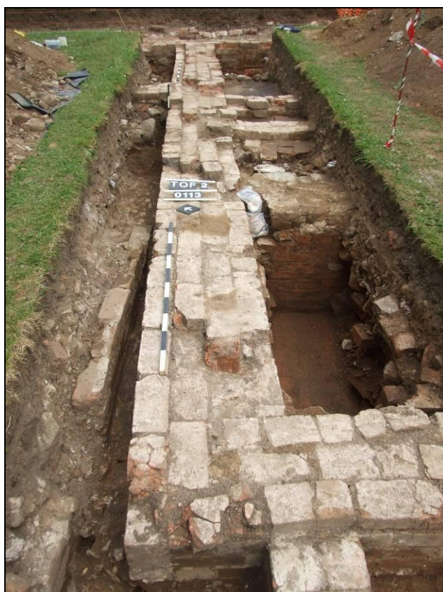
Plate 26: View of west wing of Georgian farmhouse foundations in Area 1(b) looking ENE
