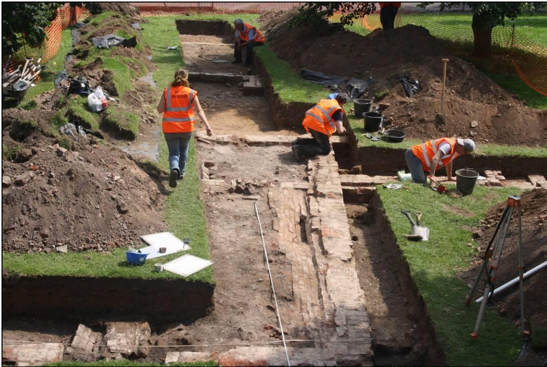
Site during cleaning looking south
