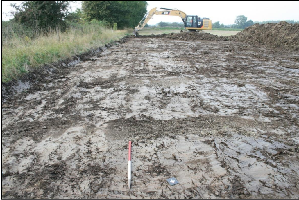
Plate 3: General shot of stripping 16/09/2014
