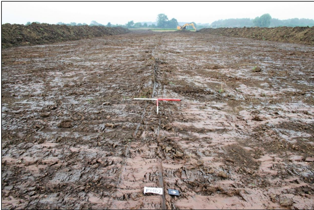
Plate 5: General shot of stripping 22/09/2014
