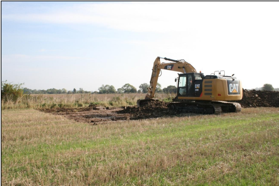
General shot of stripping at Phase 28
