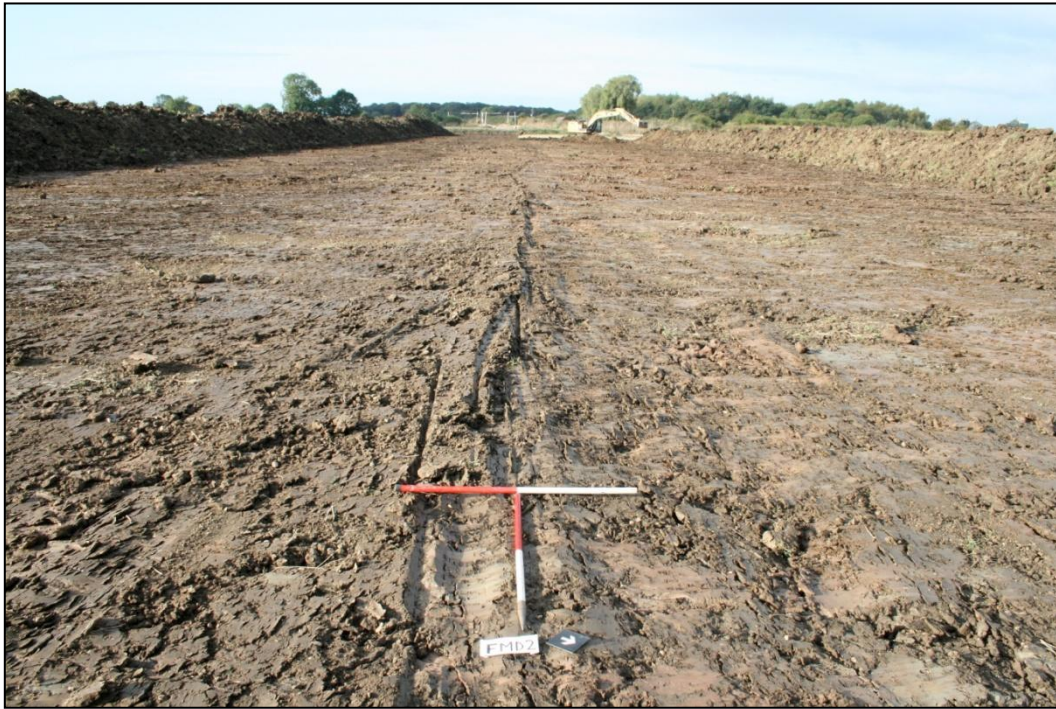
Plate 7 : General shot of stripping 1/10/2014
