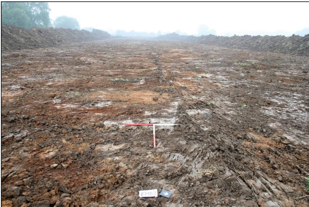
Plate 4: General shot of stripping 18/09/2014
