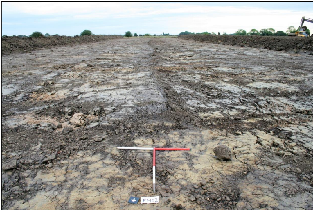
Plate 6: General shot of stripping 25/09/2014
