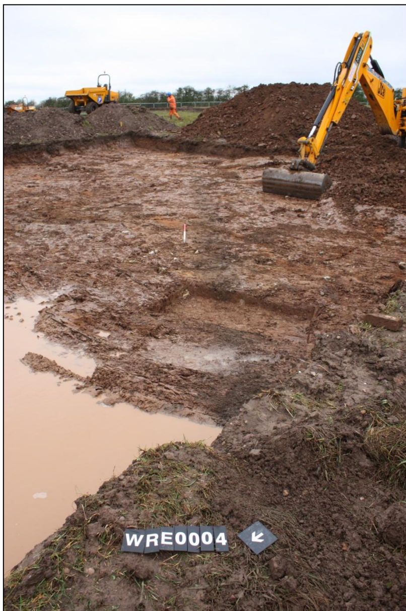
Plate 2: General view of cut [0004], looking east
