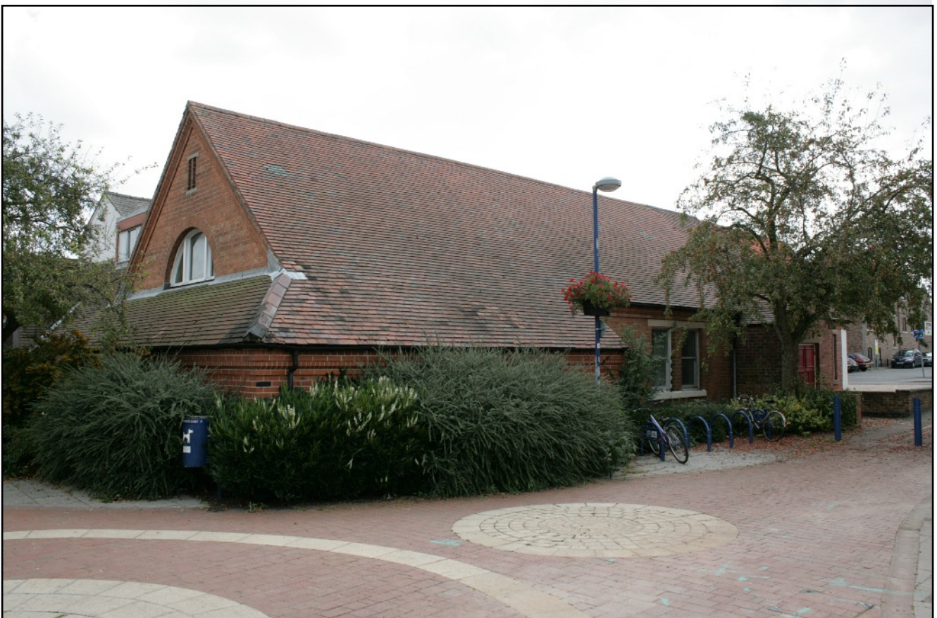
Plate 5. The Sunday School, viewed looking south east.
