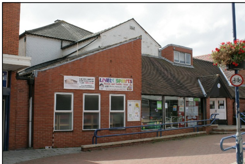
Plate 3. The north elevation of the Methodist Church complex, viewed looking south west.
