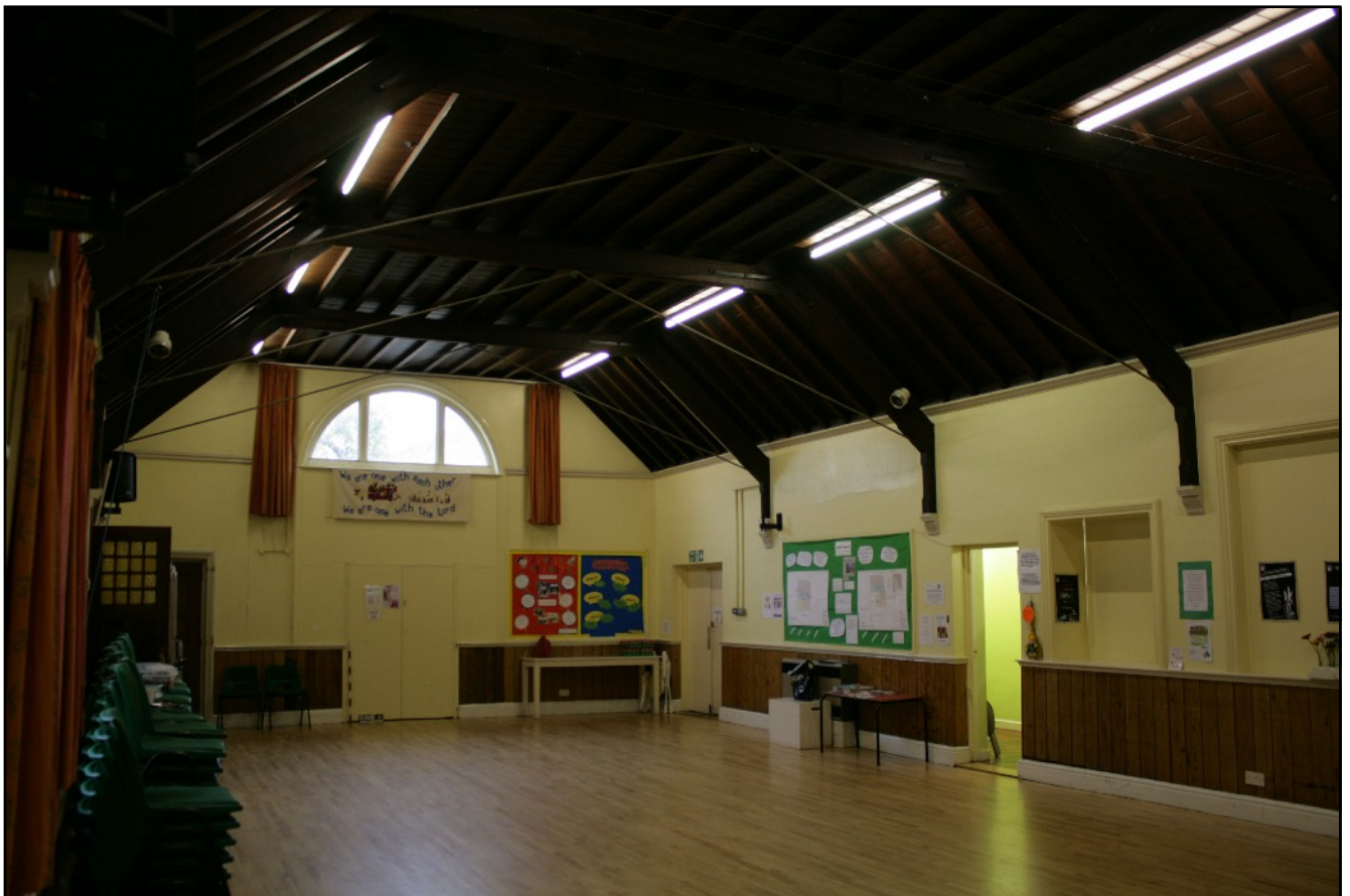
Plate 12. The interior of the earliest phase of the Sunday School viewed looking north east.
