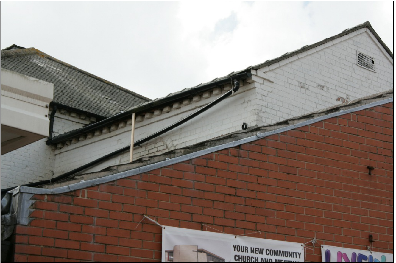
Plate 4. Detail of the northern end of the two earliest phases of the building which are painted white. Note the blocked arch windows on both the north and east elevations, viewed looking, north east.
