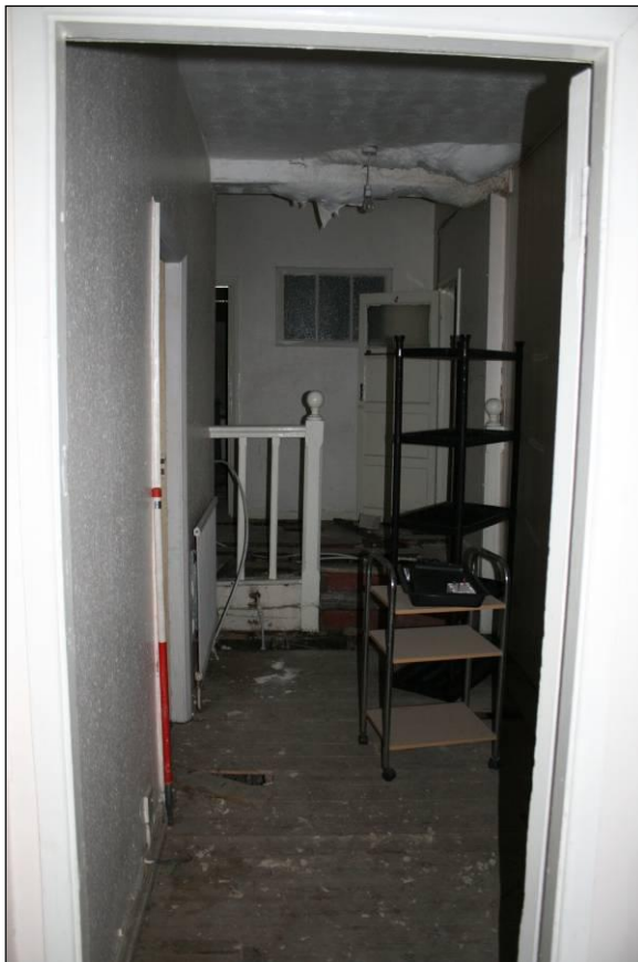
Plate 41: View of room 9, viewed looking south
