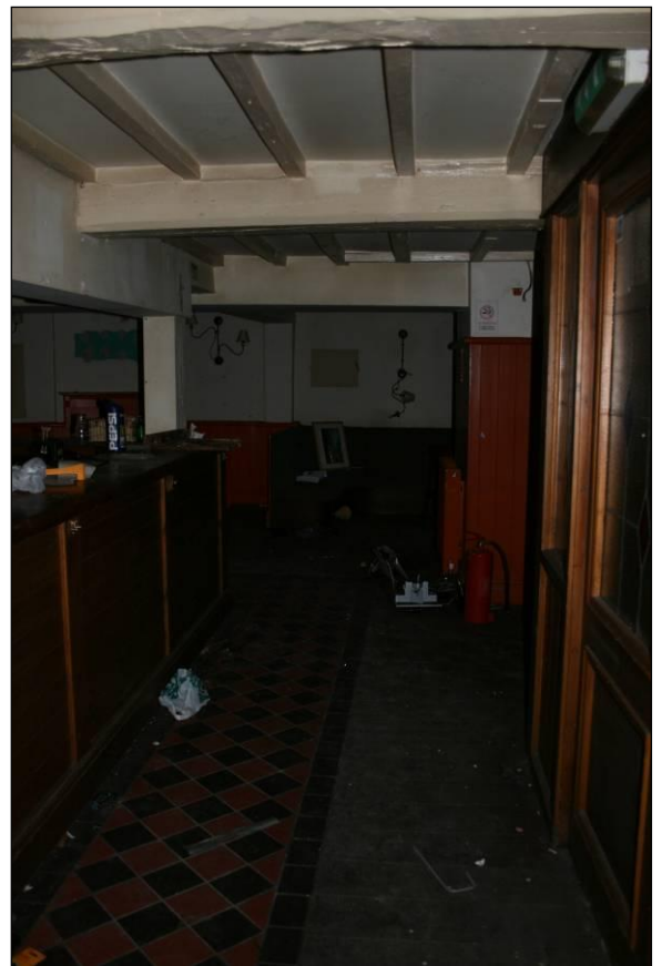
Plate 8: Detail of ceiling beam and exposed joist viewed looking west
