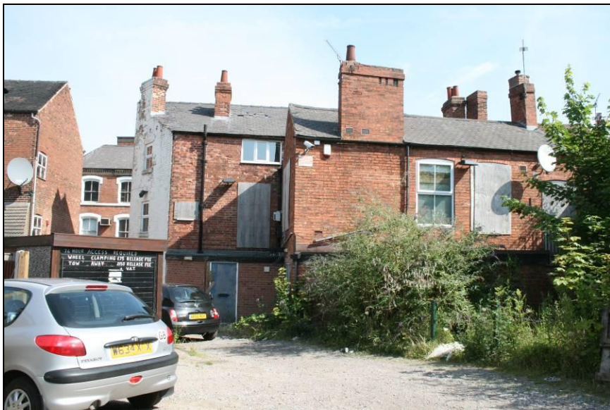
Plate 2: General shot of rear elevation, viewed looking north
