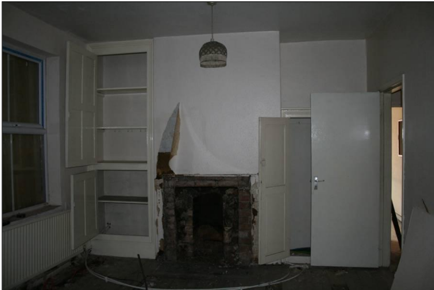
Plate 34: View of room 16, viewed looking west
