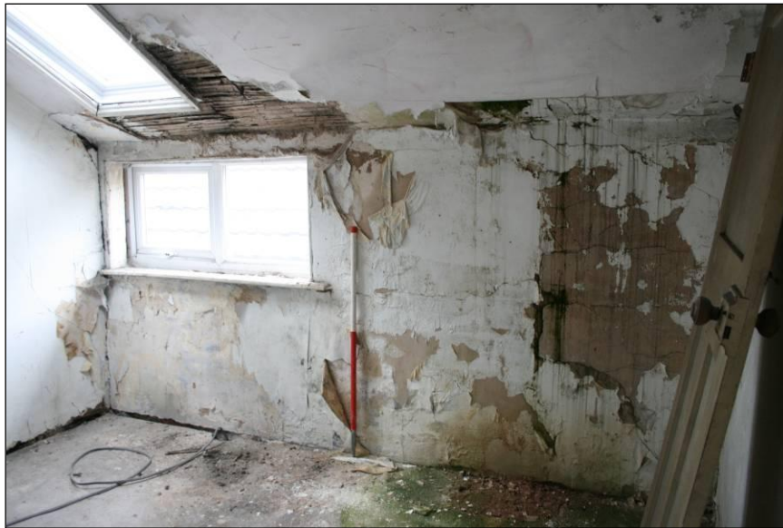
Plate 49: View of room 23, viewed looking south-east
