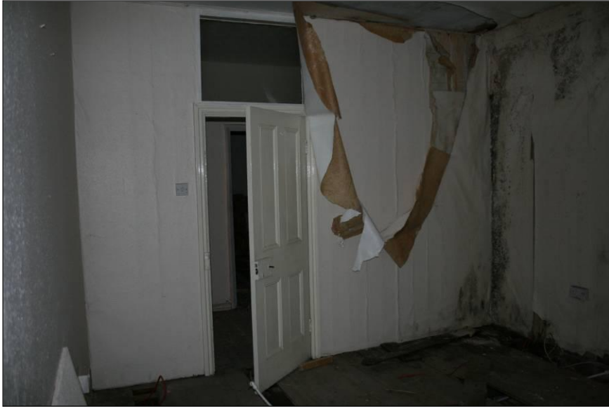
Plate 33: View of room 16, viewed looking south-east
