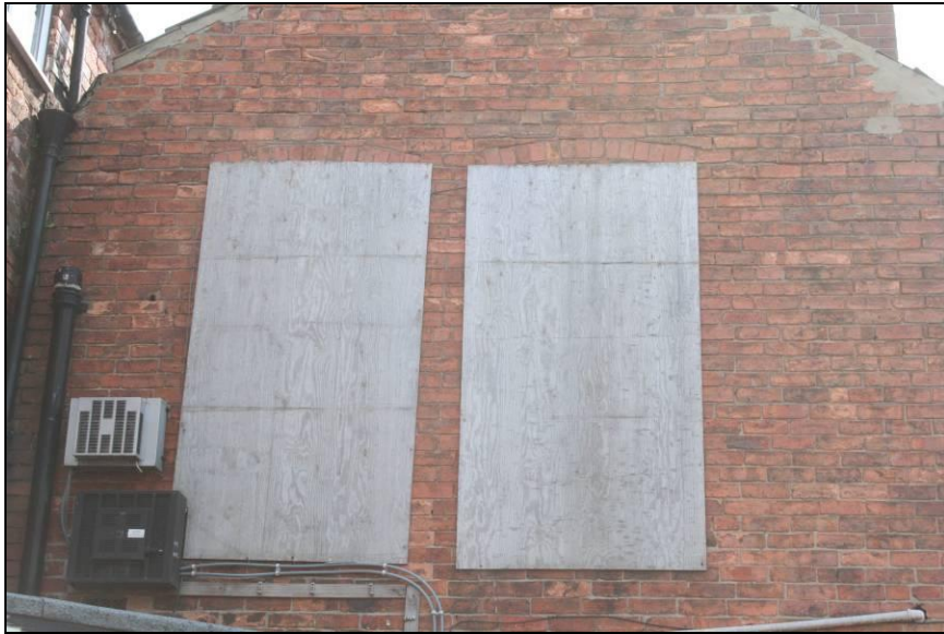
Plate 6: Detail of brick arch window in phase B, viewed looking east
