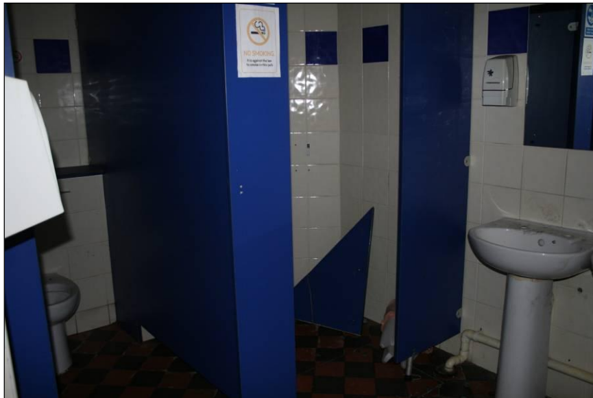
Plate 25: View of room 5, viewed looking south-west
