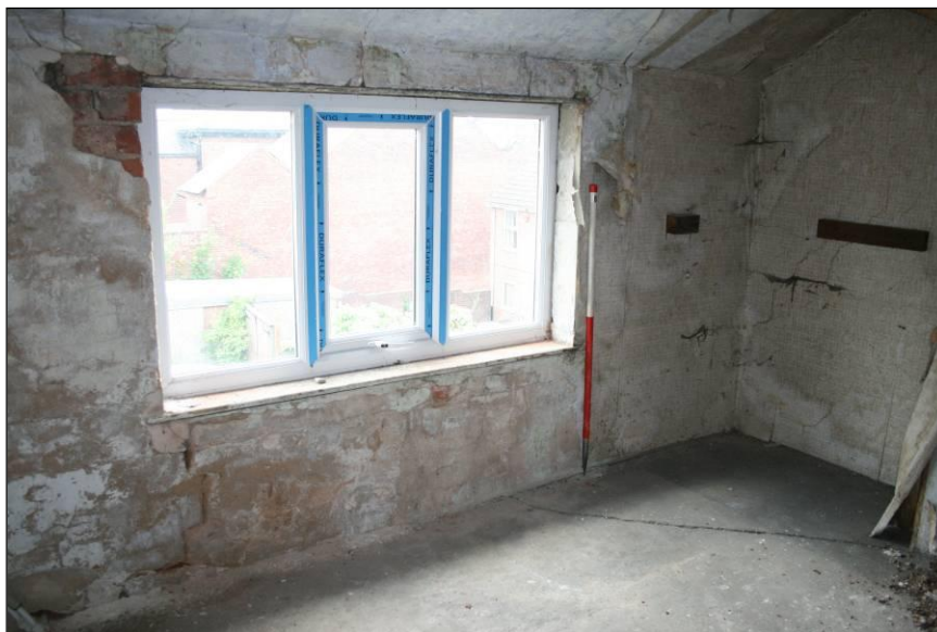
Plate 45: View of room 24, viewed looking south-west
