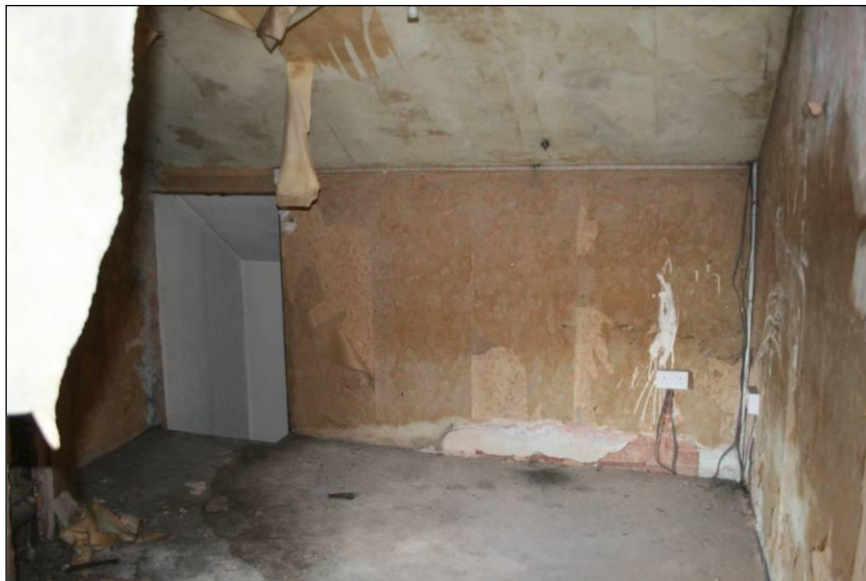
Plate 53: View of room 25, viewed looking north
