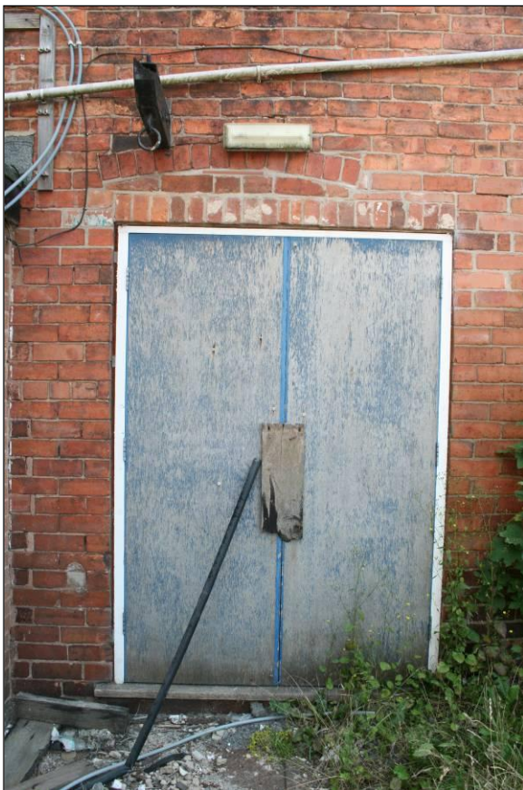
Plate 7: Detail of the former brick arch opening, viewed looking east
