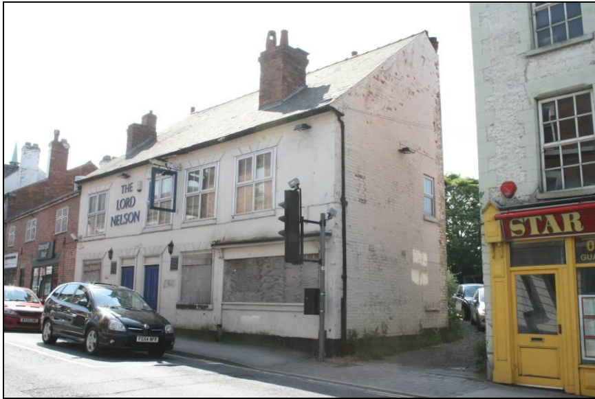
Plate 1: General shot of front elevation, viewed looking south-east
