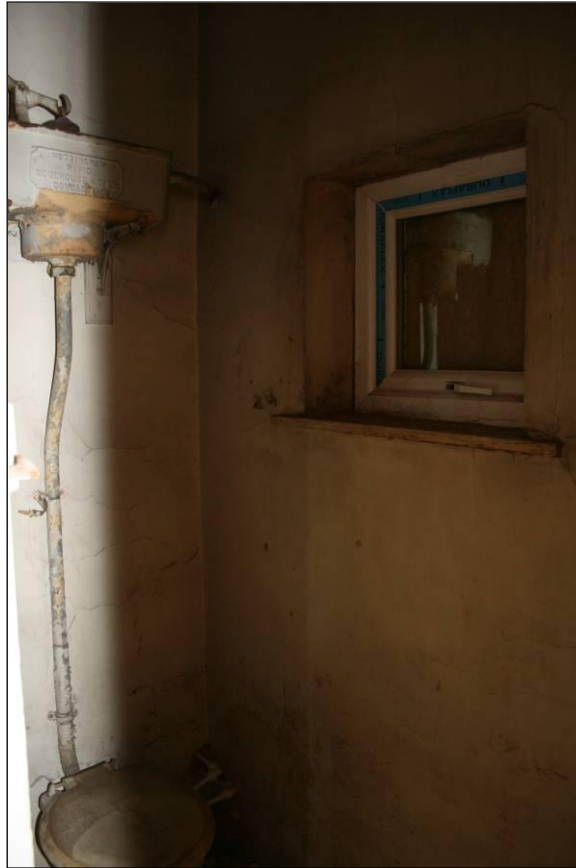
Plate 31: View of room 19, viewed looking south-east
