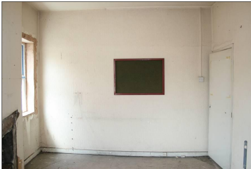
Plate 32: View of room 18, viewed looking north
