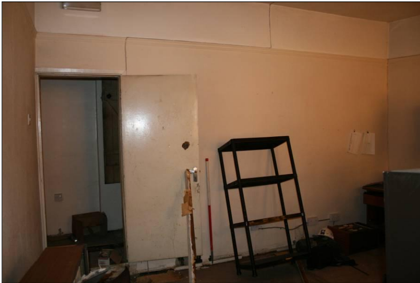
Plate 43: View of room 7, viewed looking south-west
