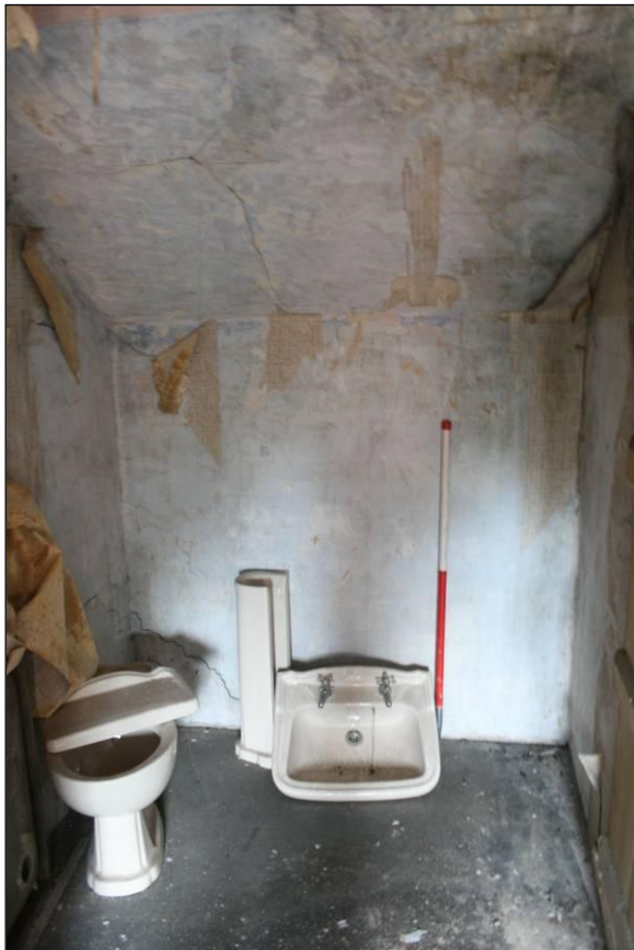
Plate 47: View of room 24, viewed looking north
