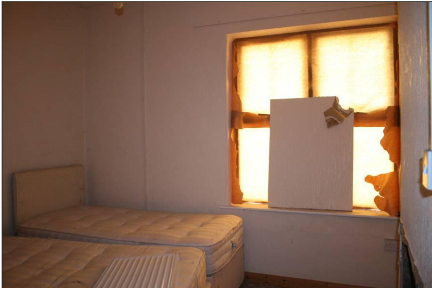
Plate 30: View of room 20, viewed looking north-west
