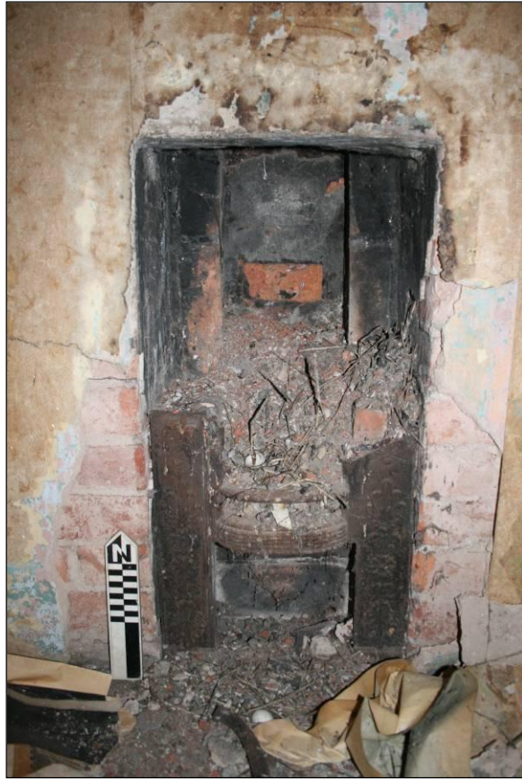
Plate 15: Detail of original hob grate fireplace in room 25, viewed looking south-west
