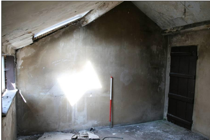
Plate 52: View of room 22, viewed looking north-west
