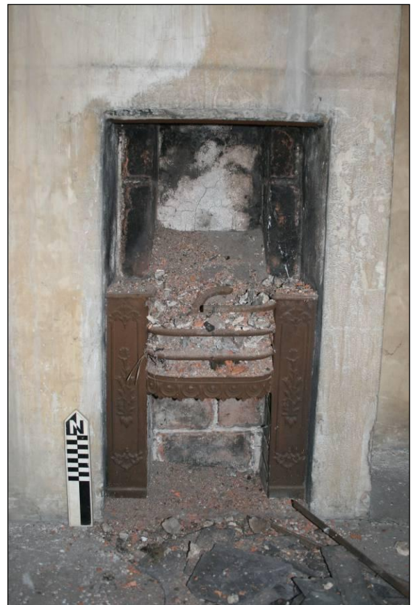
Plate 14: Detail of original hob grate fireplace in room 22, viewed looking east
