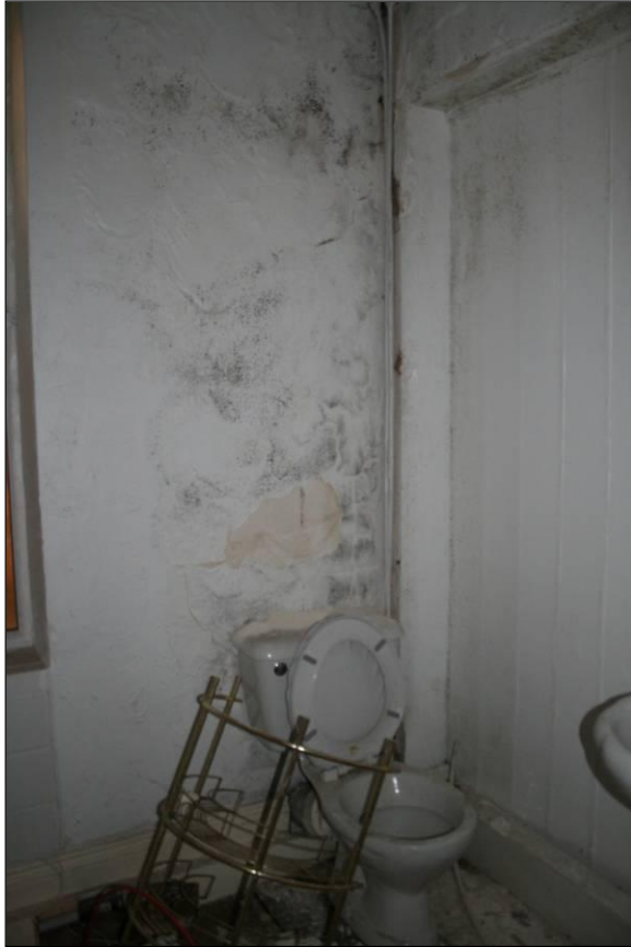
Plate 40: View of room 11, viewed looking north-west
