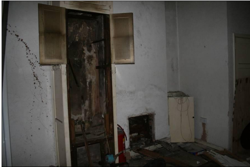
Plate 38: View of room 14, viewed looking south-east
