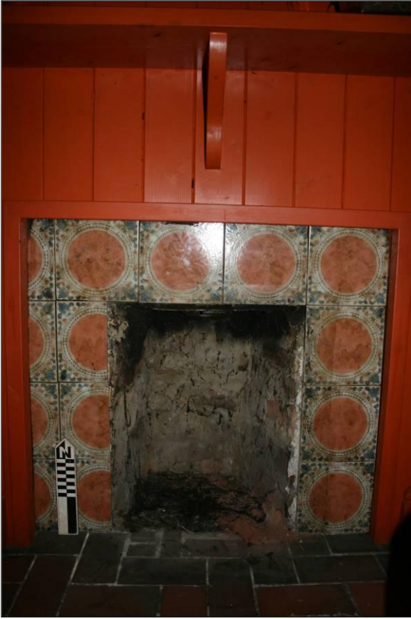
Plate 9: Detail of Victorian tiling around the fireplace, viewed looking east
