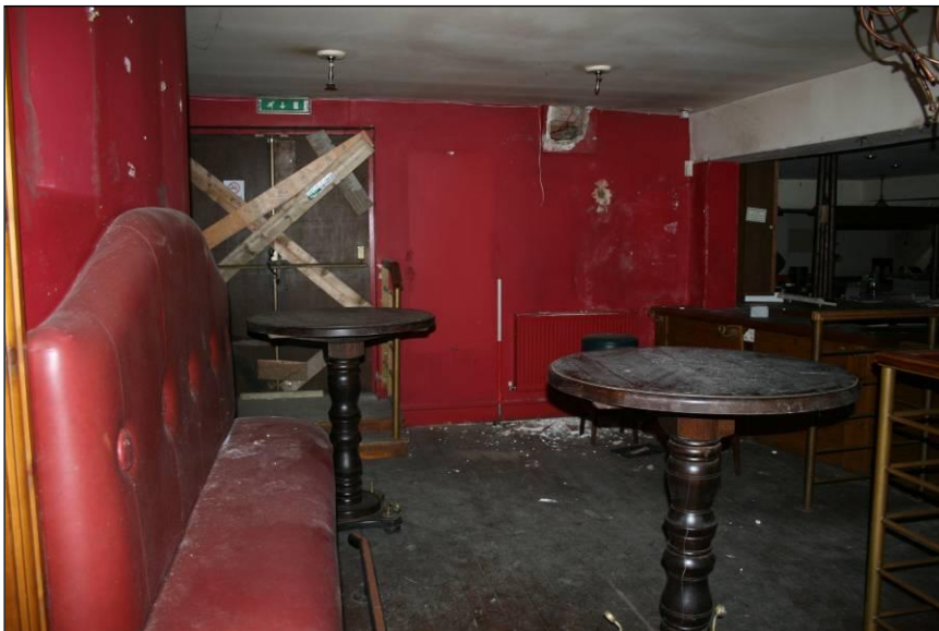
Plate 28: General shot of room 2, viewed looking west
