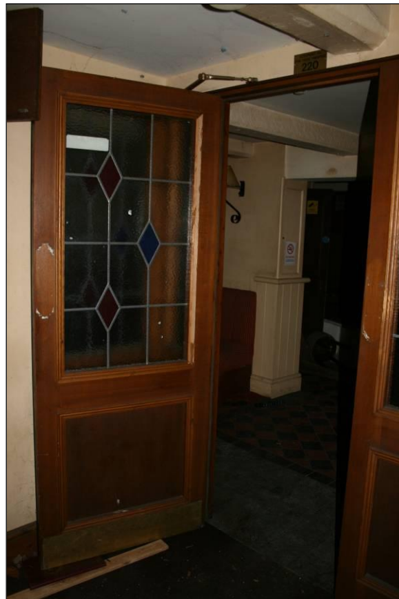
Plate 19: General shot of room 1, viewed looking south-east
