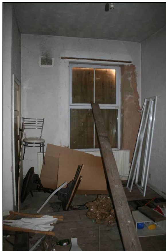
Plate 37: View of room 14, viewed looking south
