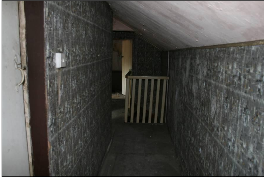
Plate 51: View of room 21, viewed looking west
