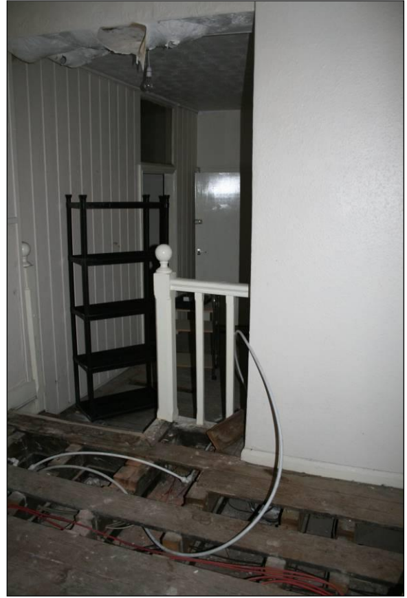
Plate 10: View of room 9, central landing area, viewed looking north-west
